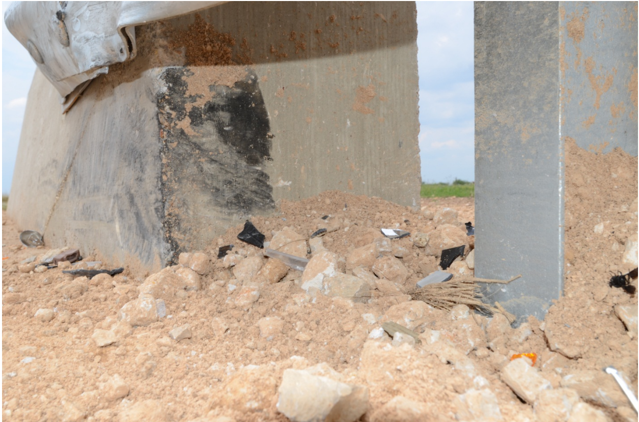
Figure 5.3. TxDOT TL-3 Transition after Test No. 490022-4.
