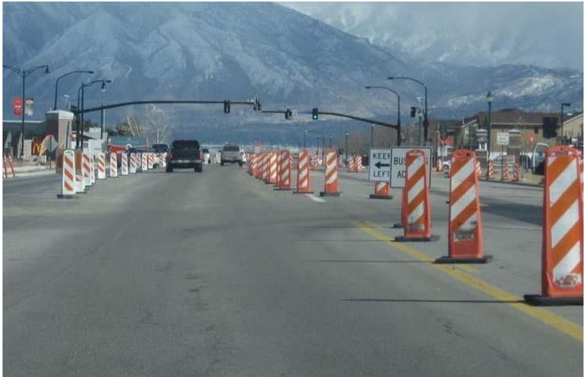
Figure 1. Improper sign height among channelizing devices.
