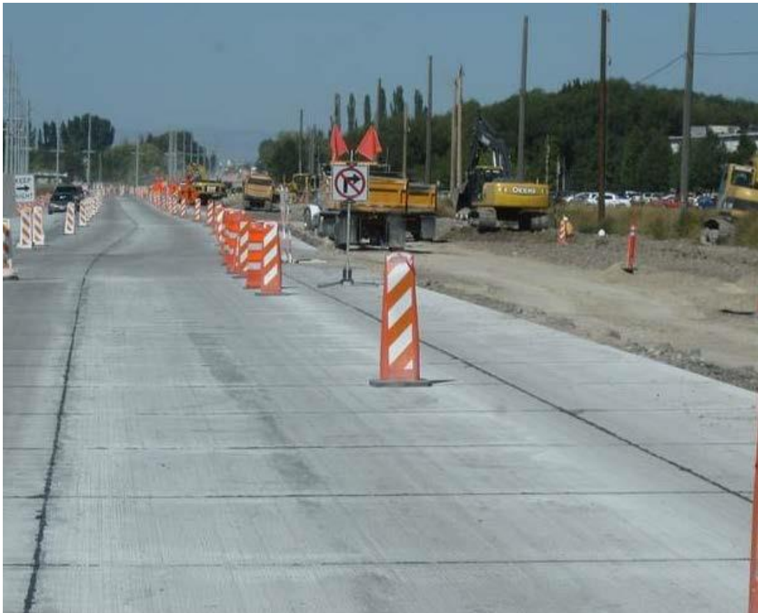
Figure 2. Proper sign height among channelizing devices.
