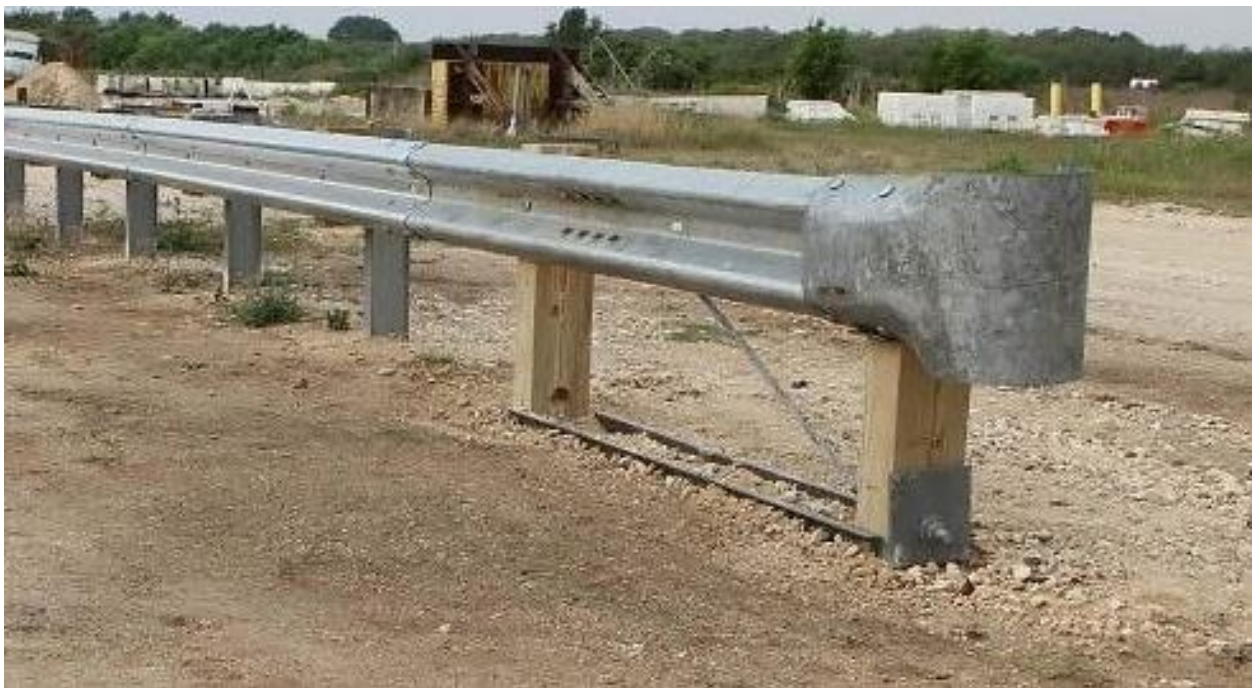
Figure 2. TxDOT Trailing-End Anchorage System [7]
