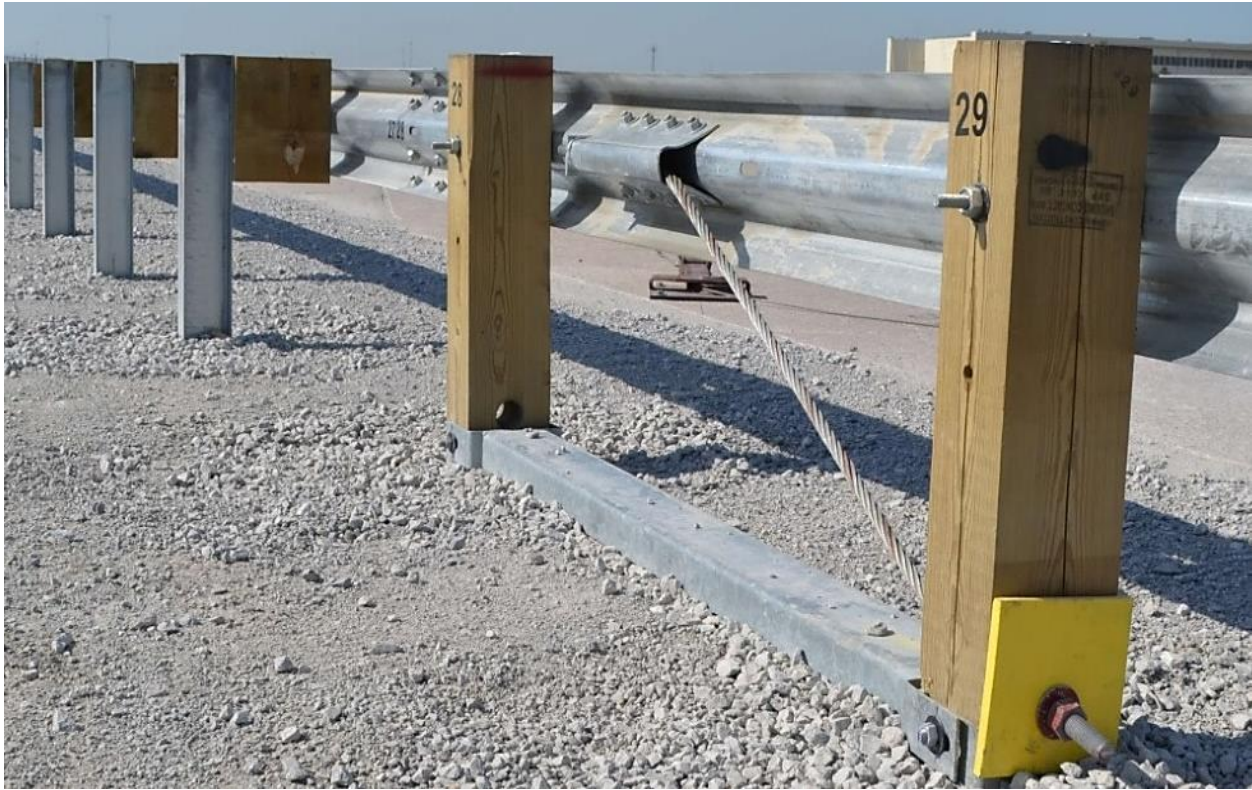
Figure 1. MGS Trailing-End Anchorage System [1-3]
