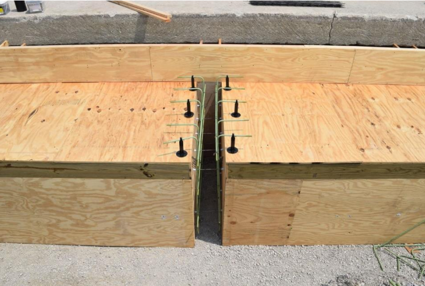
Figure 18. Concrete Culvert Support Walls Framework, Test Nos. CMGS-1 and CMGS-2
