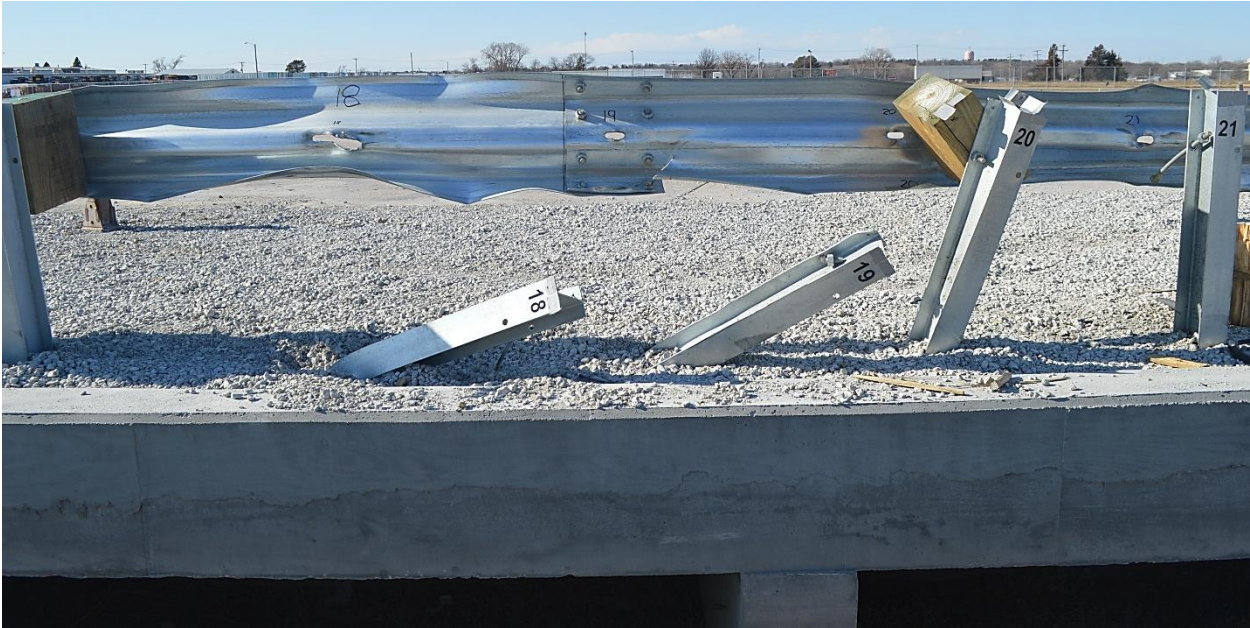
Figure 60. System Damage, Test No. CMGS-1
