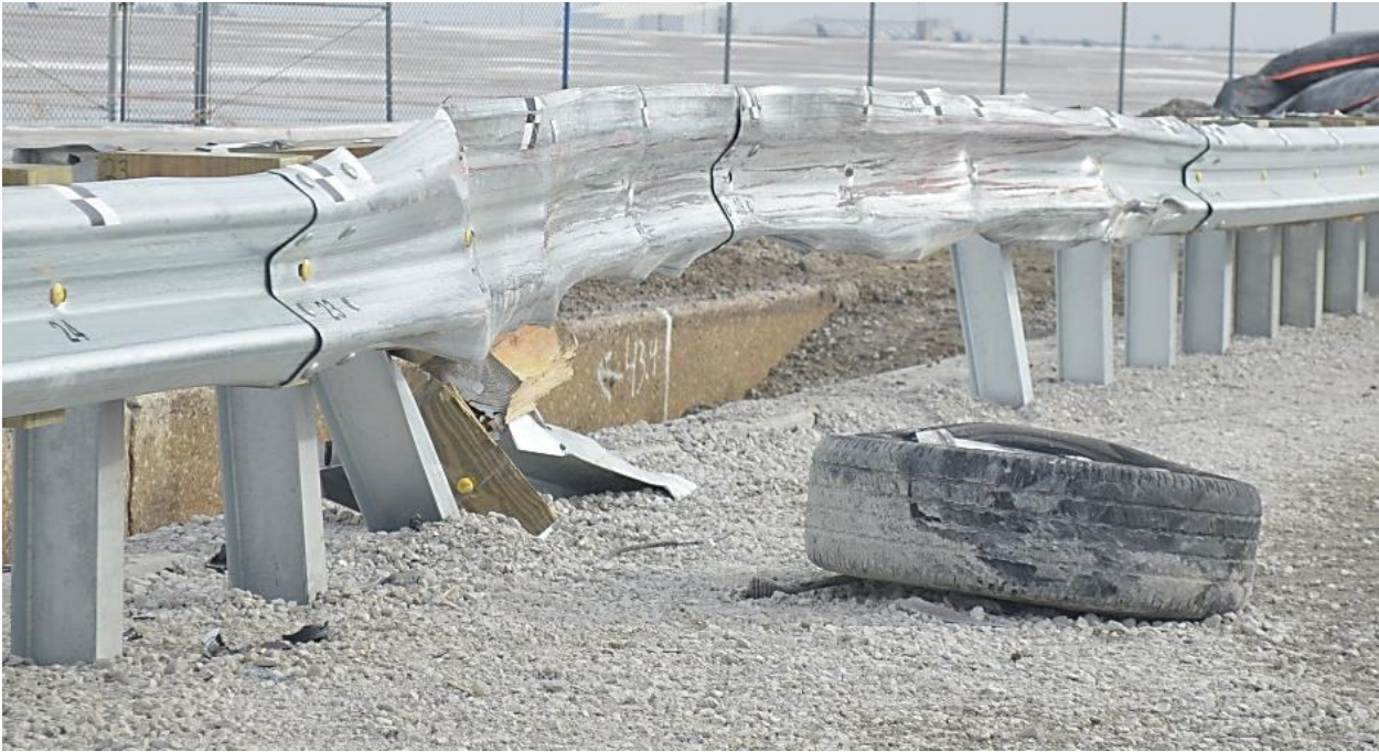
Figure 80. System Damage, Test No. CMGS-2
