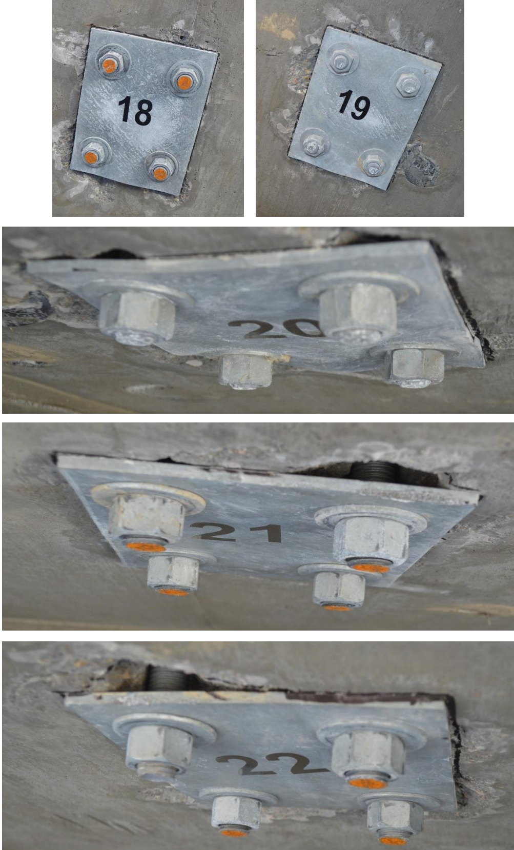
Figure 65. Washer Plate Nos. 18 through 22 After Test, Test No. CMGS-1
