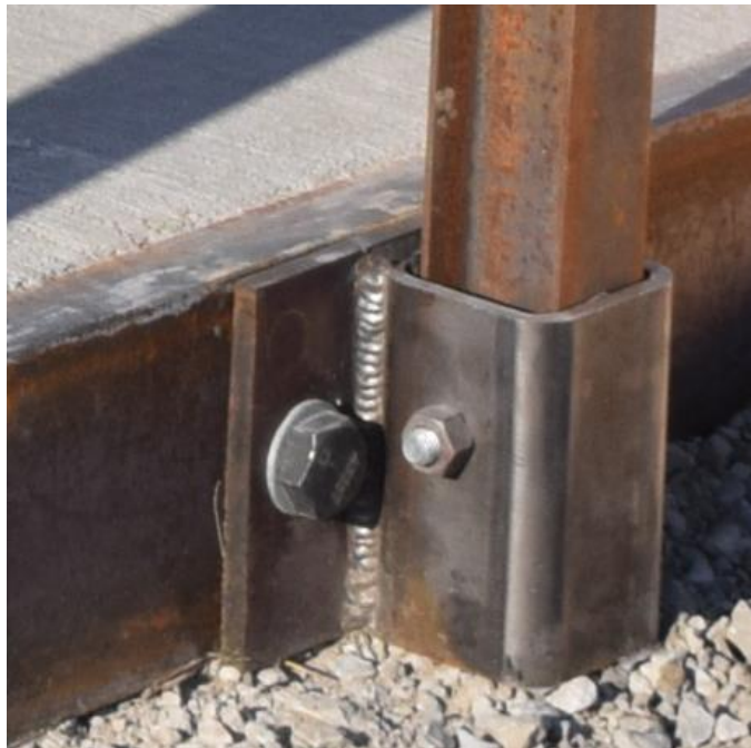
Figure 11. Coupling Nut and Threaded Rod Attachment of Socket Assembly to Deck
