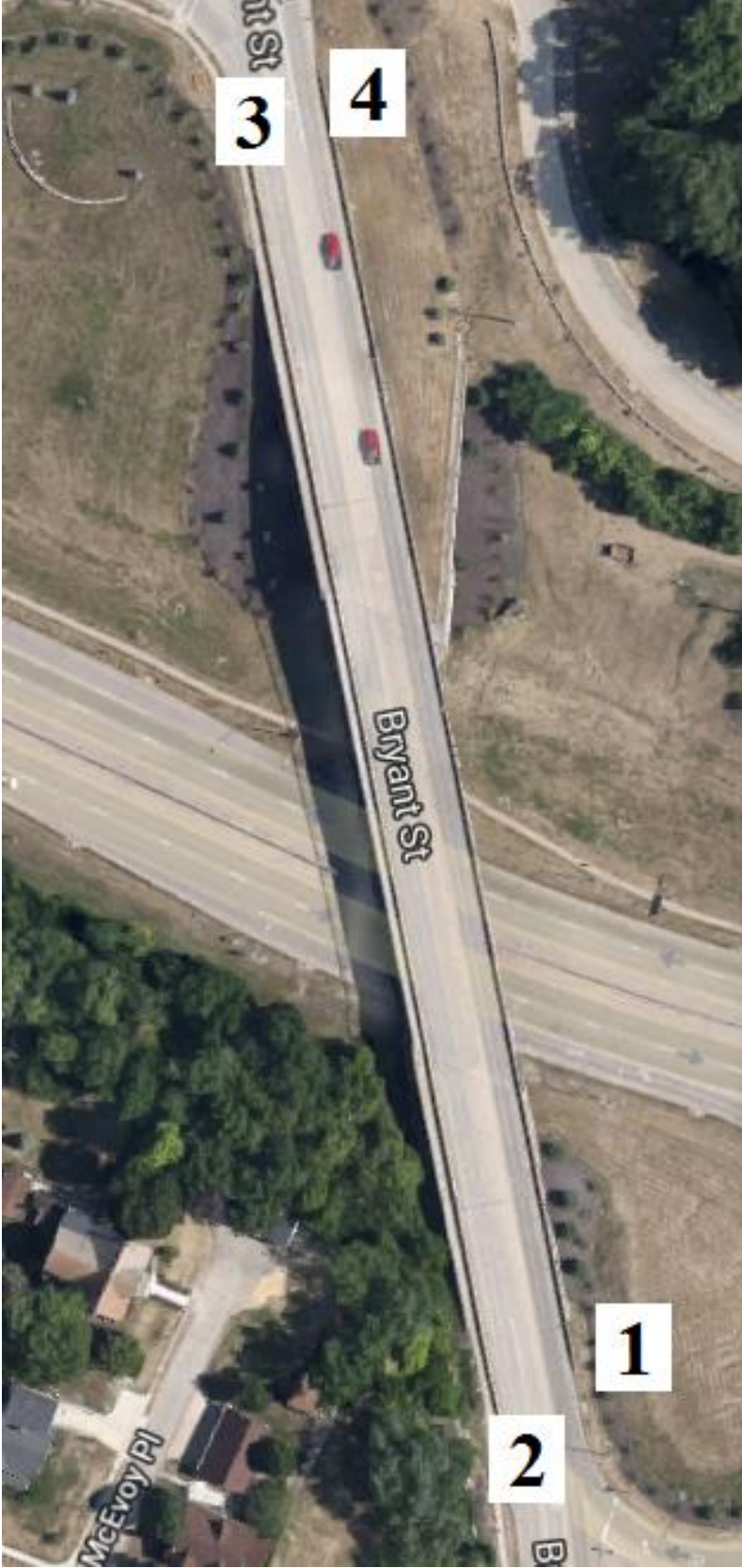
Figure B-51. Bridge No. 3119.00020 [1]
