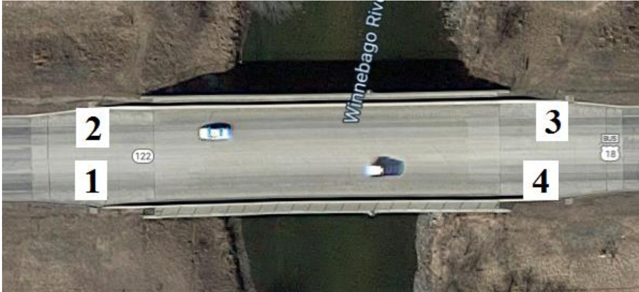
Figure B-23. Bridge No. 1710.2S122 [1]
