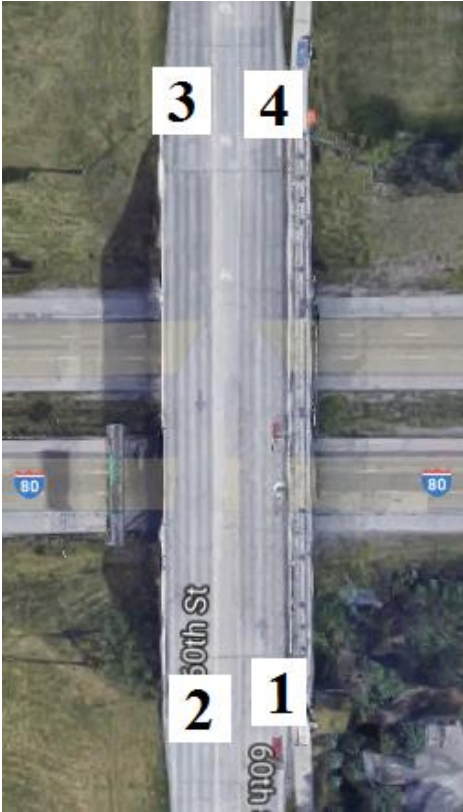
Figure B-138. Bridge No. 7722.4O080 [1]
