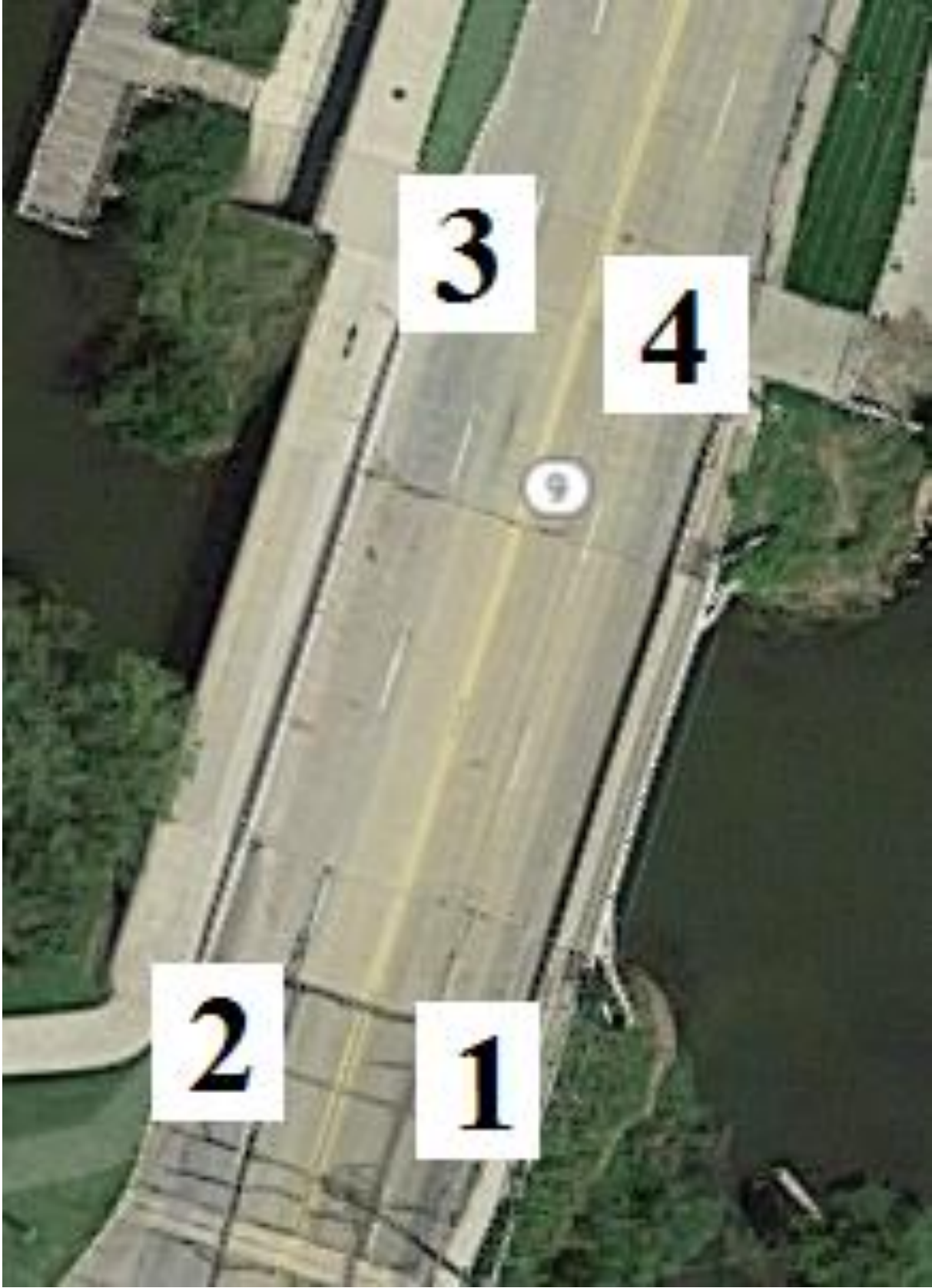
Figure B-48. Bridge No. 3026.6S071 [1]
