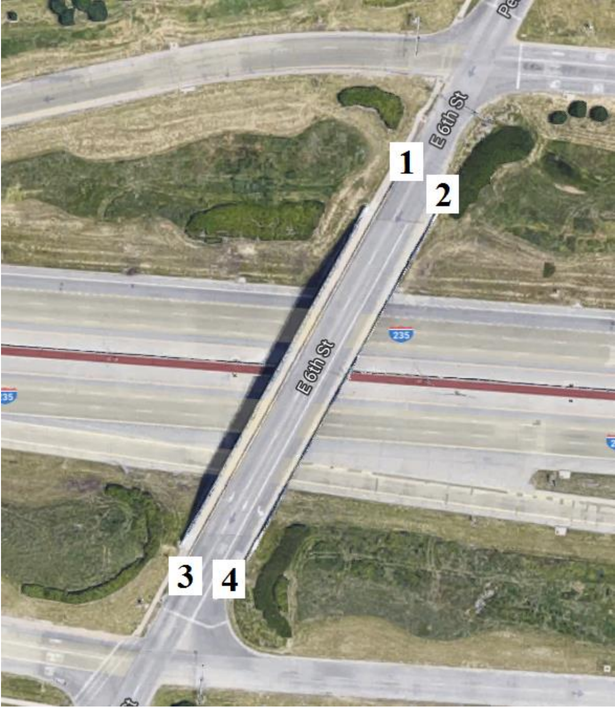
Figure B-131. Bridge No. 7708.8O235 [1]
