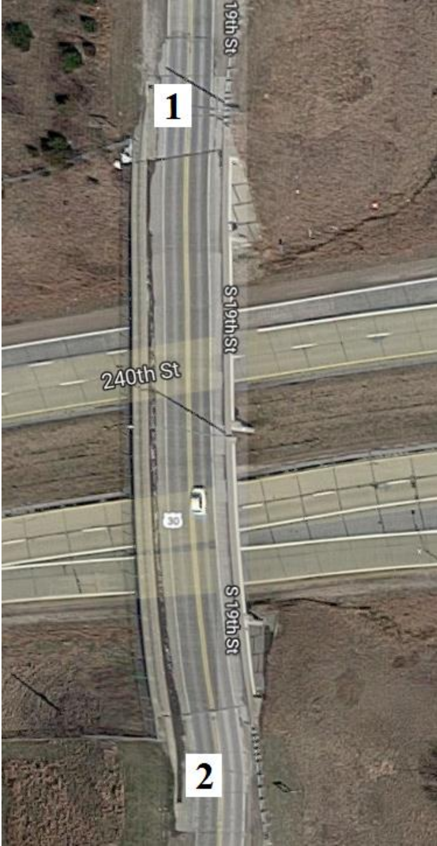
Figure B-163. Bridge No. 8558.4O030 [1]
