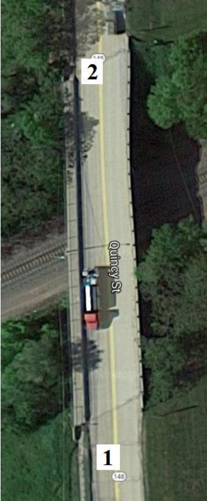
Figure B-2. Bridge No. 0230.5S148 [1]
