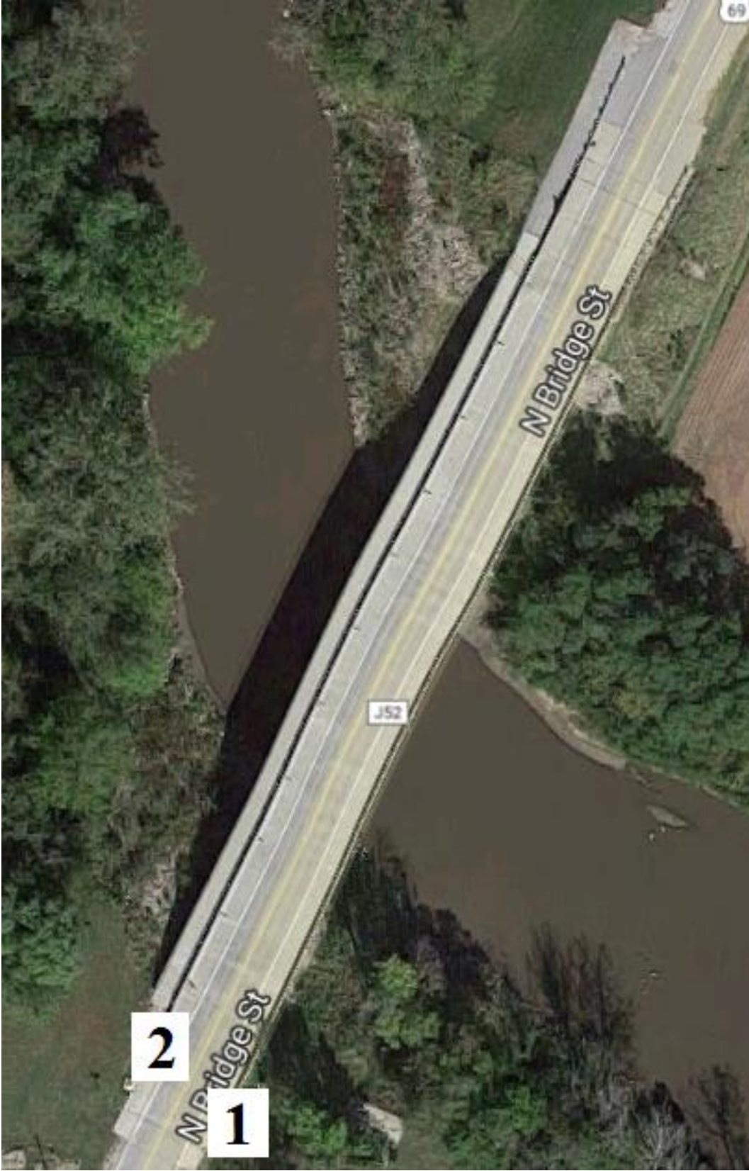
Figure B-34. Bridge No. 2711.3S069 [1]
