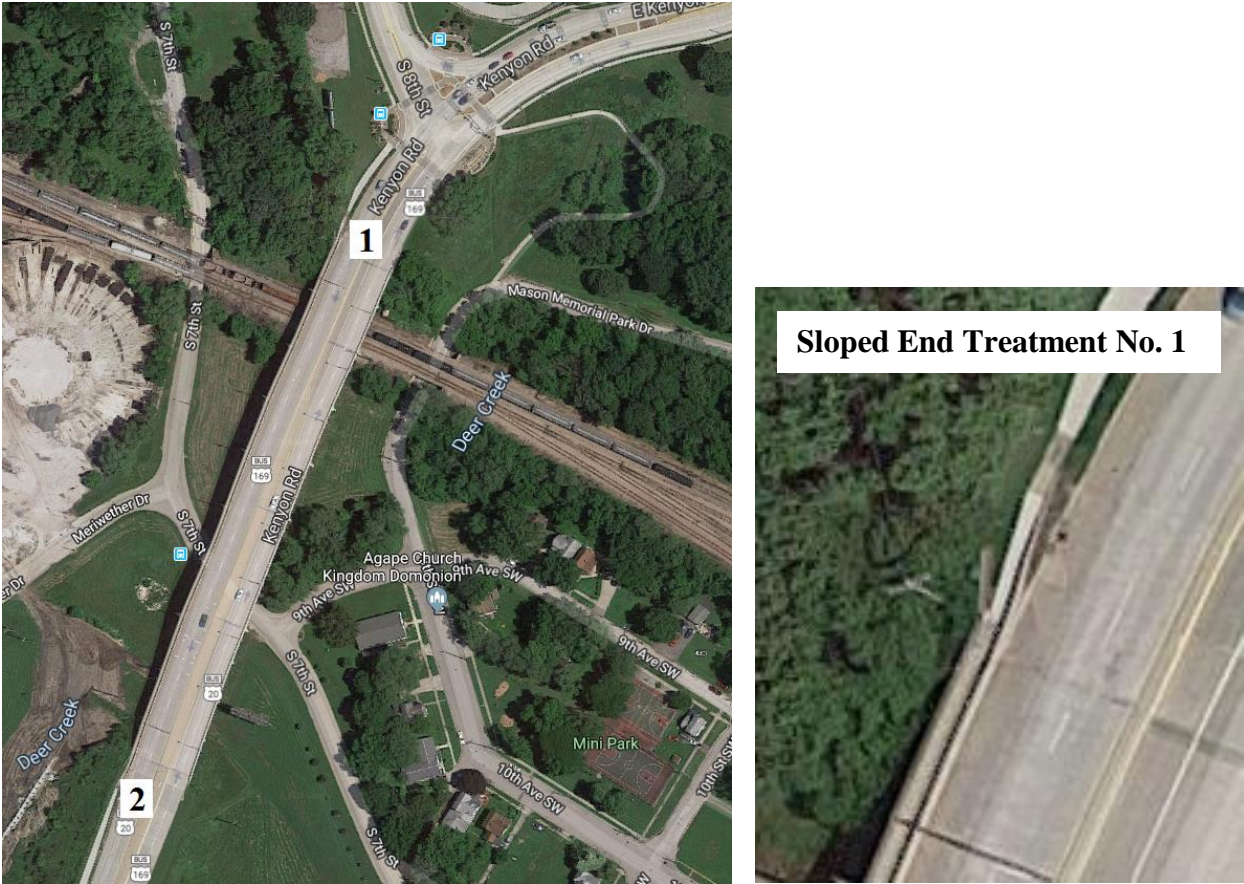
Figure 153. Bridge No. 9401.5L926 with Sloped End Treatments Labeled [1]
