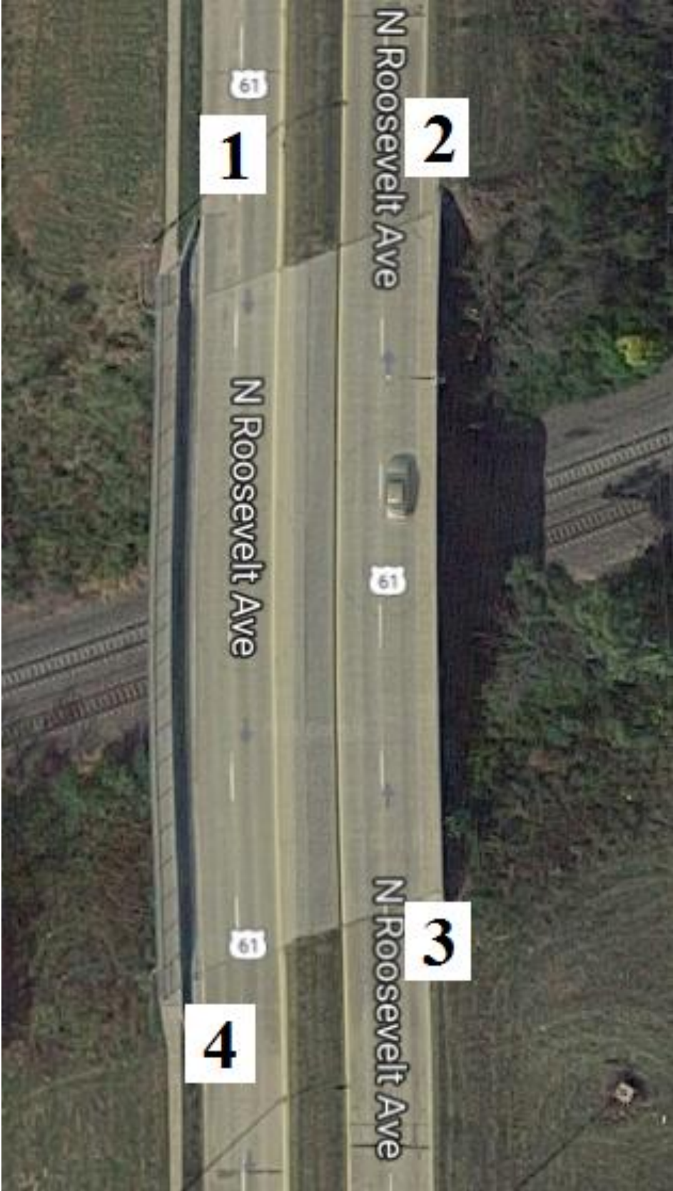
Figure B-39. Bridge No. 2942.2L061 [1]
