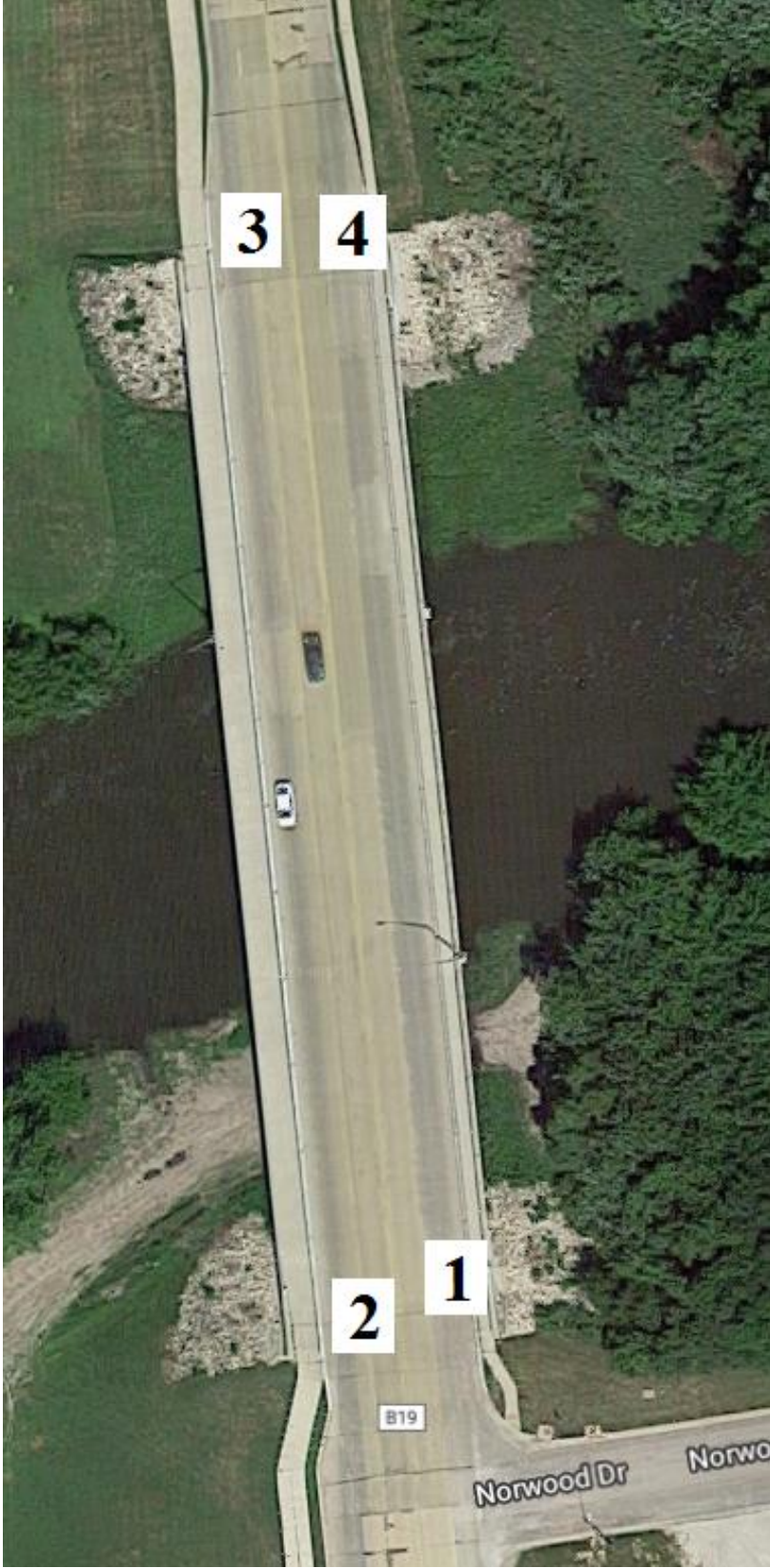
Figure B-88. Bridge No. 5598.7S169 [1]
