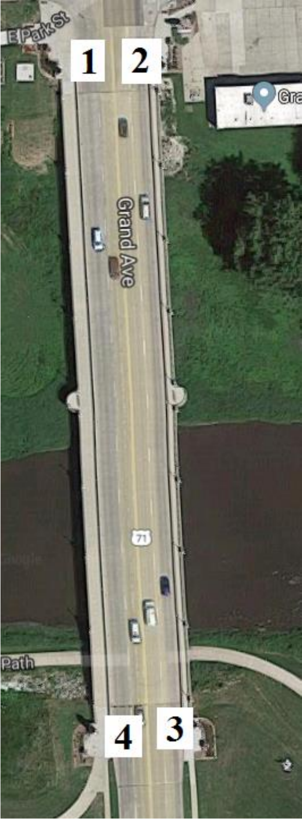
Figure B-28. Bridge No. 2181.0S018 [1]
