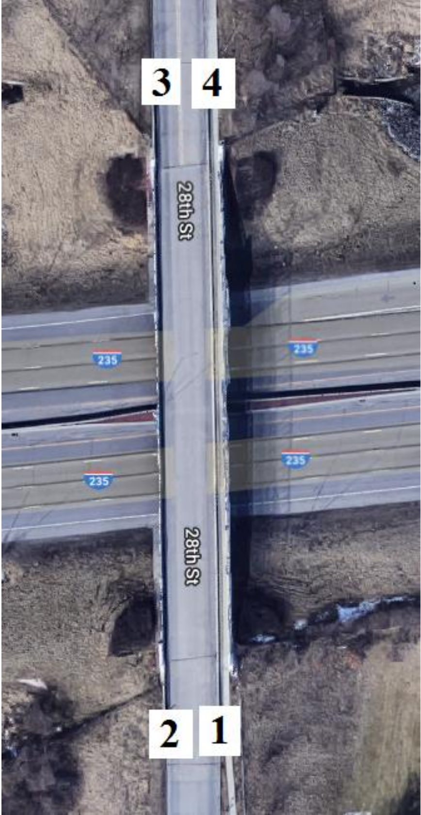
Figure B-117. Bridge No. 7701.8O235 [1]
