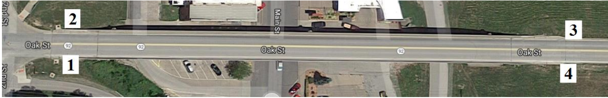
Figure B-101. Bridge No. 5851.3S092 [1]
