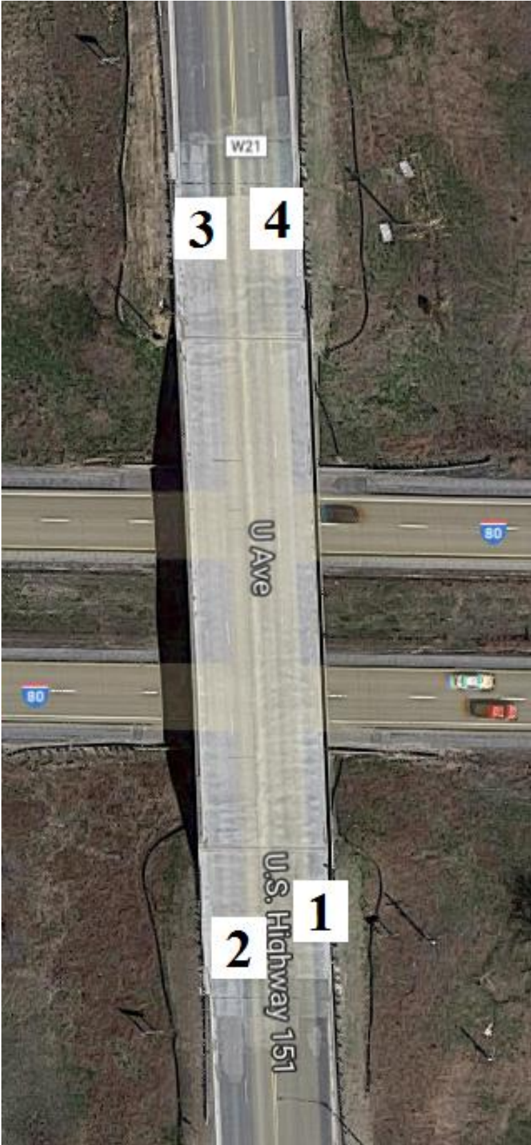
Figure B-70. Bridge No. 4800.2S151 [1]
