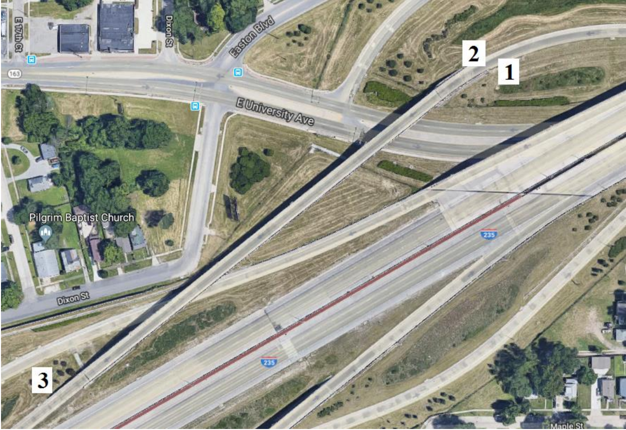
Figure B-135. Bridge No. 7710.0A235 [1]
