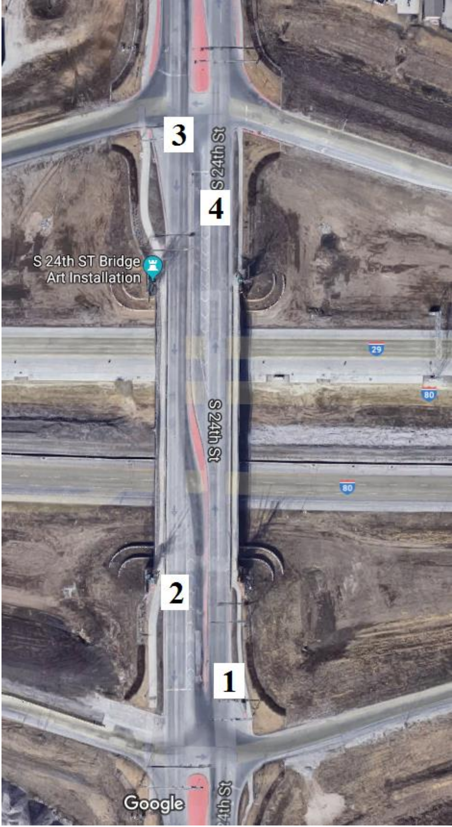
Figure B-148. Bridge No. 7801.7O080 [1]
