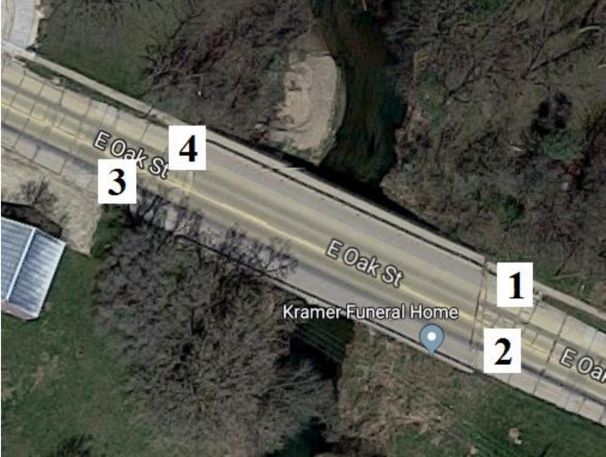
Figure B-87. Bridge No. 5363.6S038 [1]
