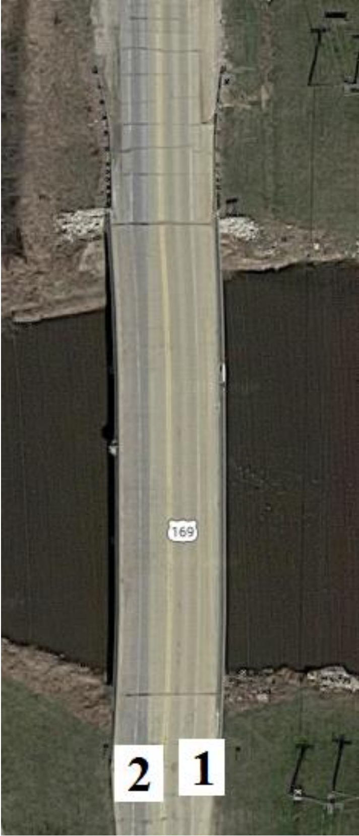
Figure B-33. Bridge No. 2589.1S169 [1]
