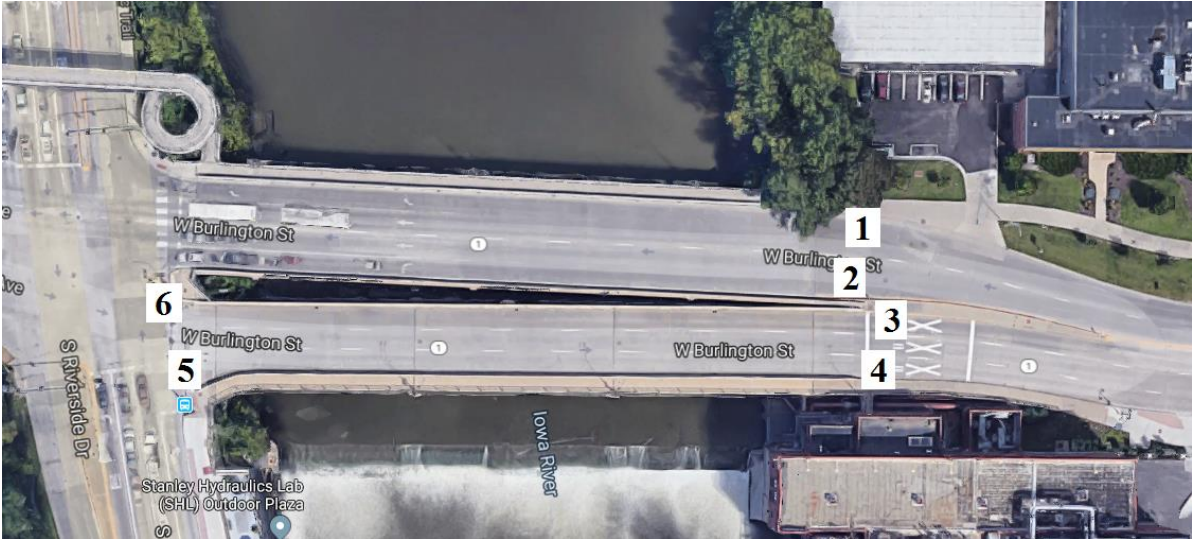
Figure B-81. Bridge No. 5285.9L001 [1]
