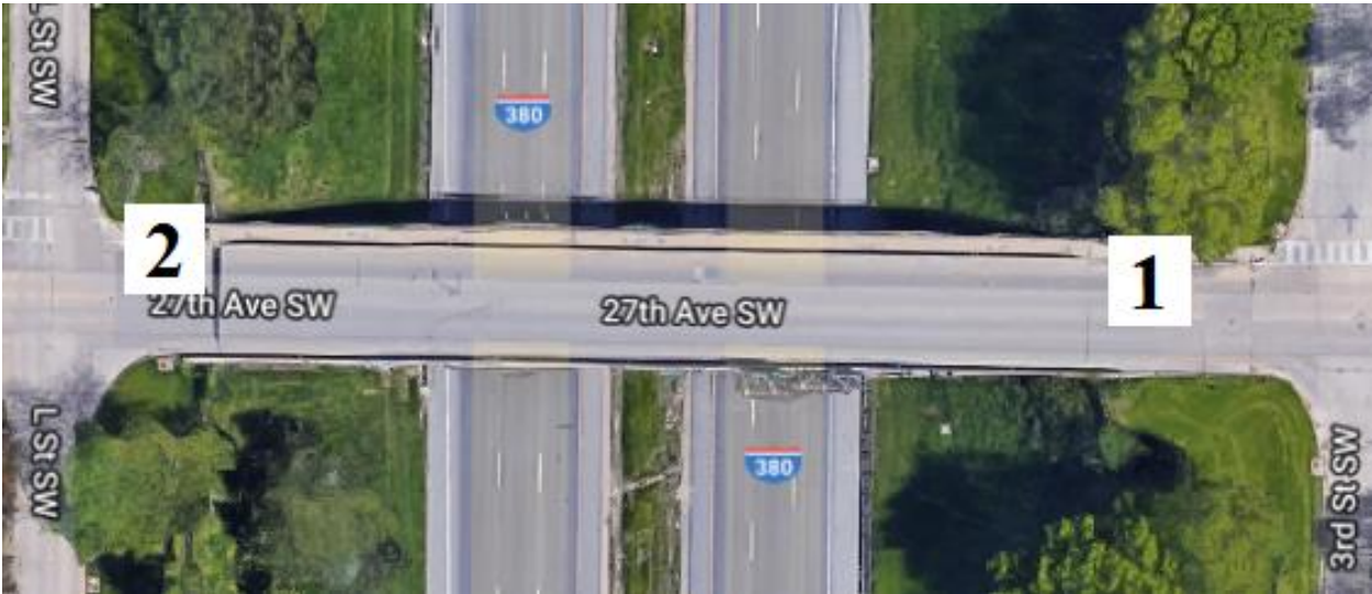
Figure B-90. Bridge No. 5718.00380 [1]
