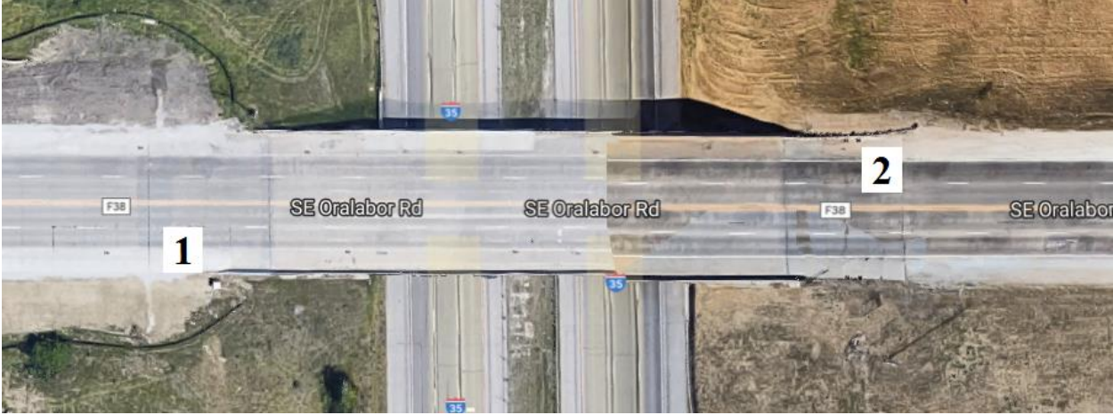
Figure B-118. Bridge No. 7702.4S160 [1]
