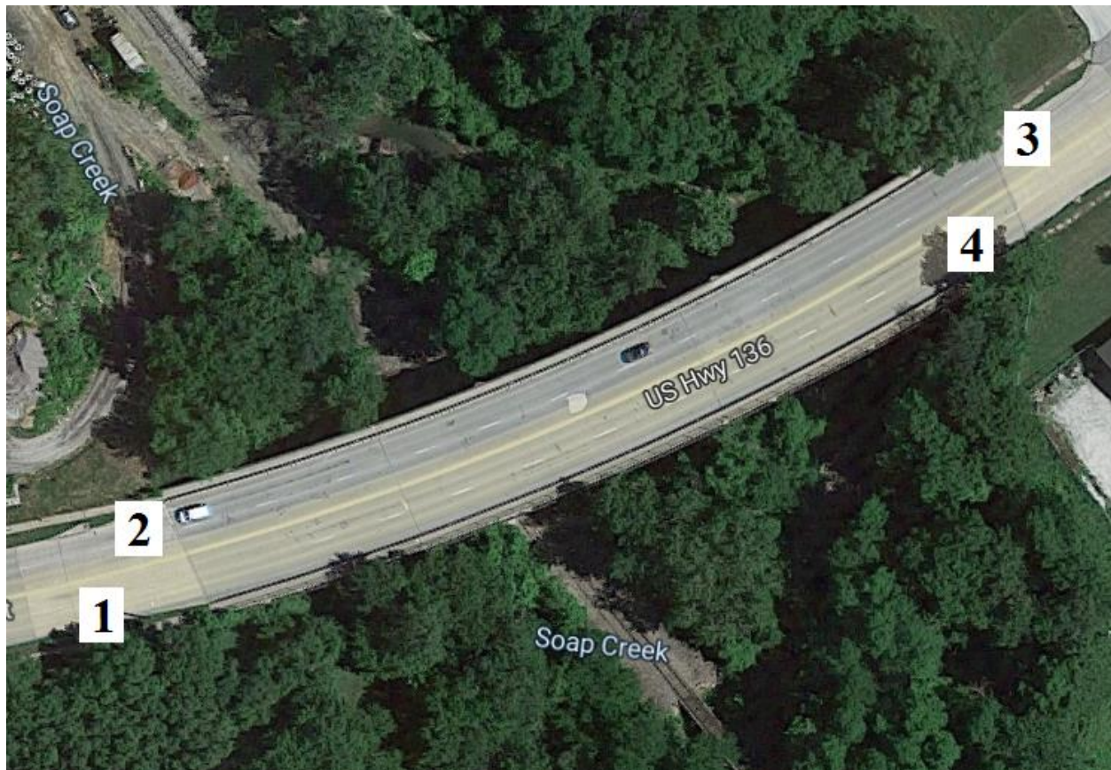
Figure 158. Bridge No. 5602.4S136 with Sloped End Treatments Labeled [1]
