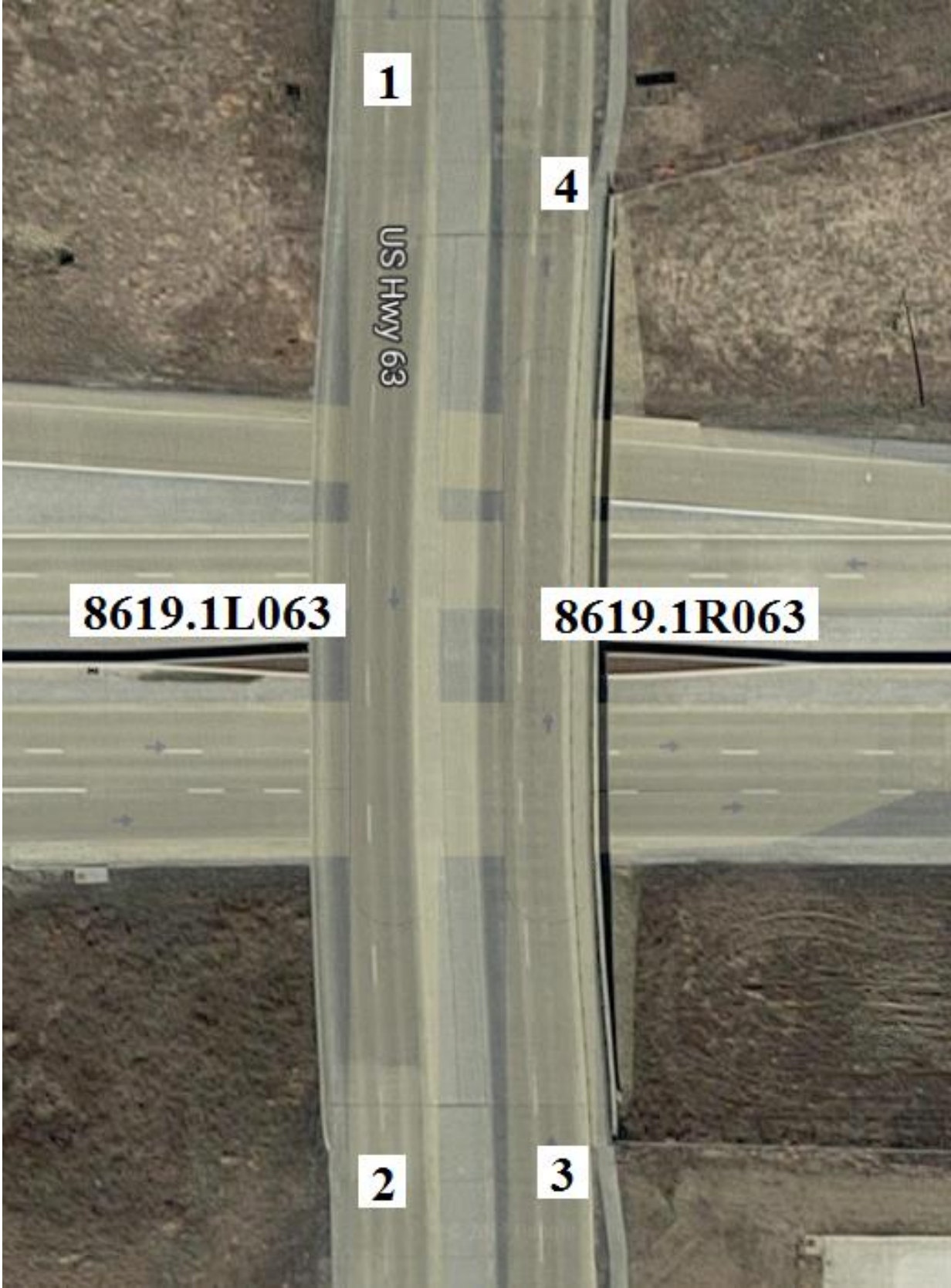
Figure B-166. Bridge Nos. 8619.1L063 and 8619.1R063 [1]
