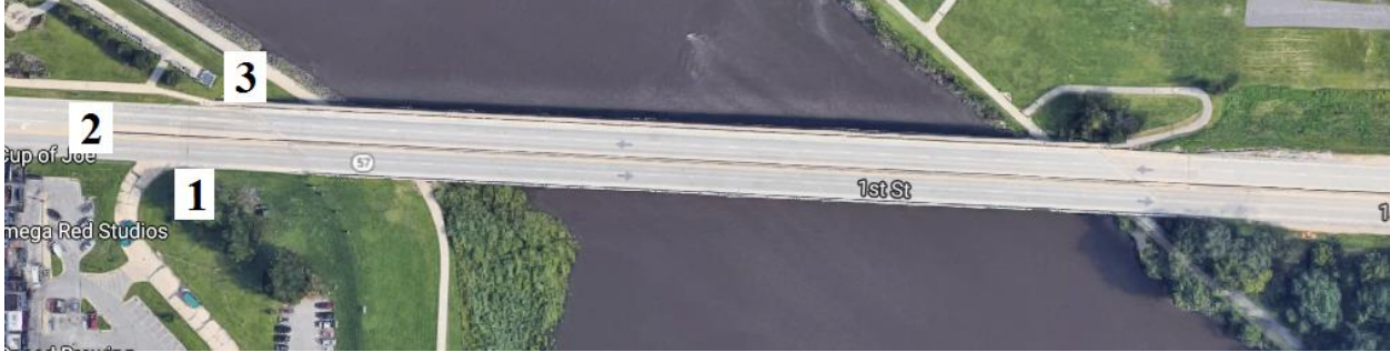
Figure B-10. Bridge No. 0743.1S057 [1]
