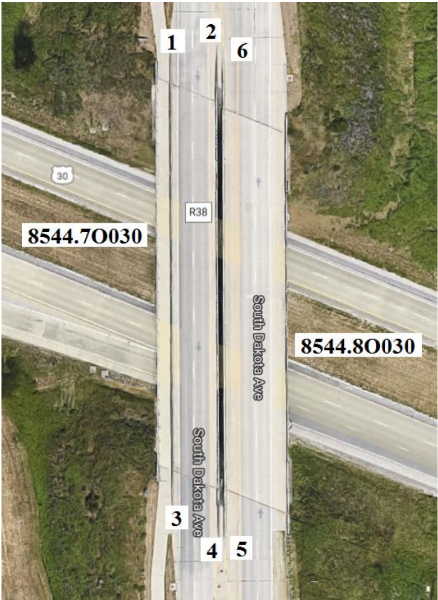
Figure 94. Bridge Nos. 8544.70030 and 8544.80030 [1]
