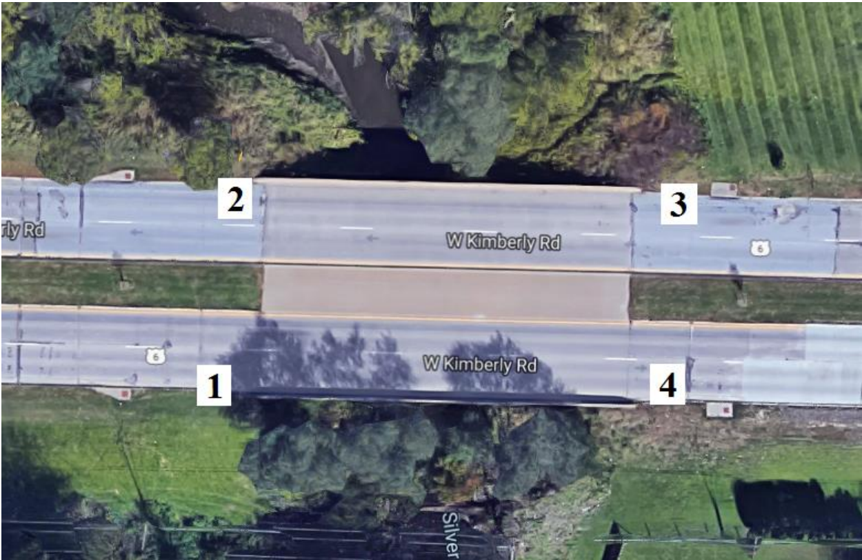
Figure B-152. Bridge No. 8204.9S006 [1]
