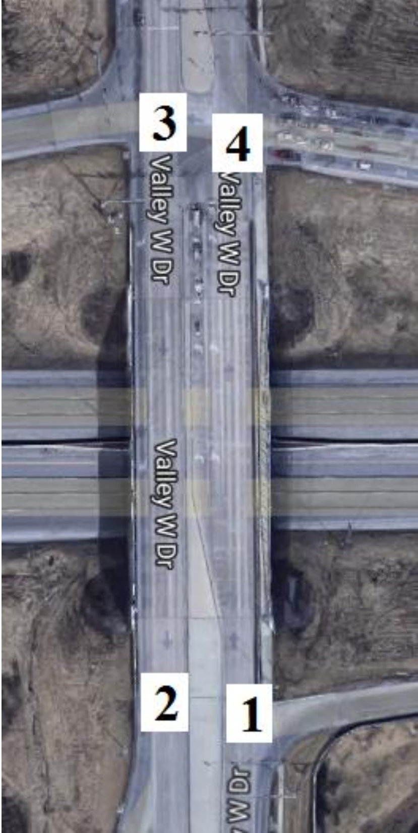
Figure B-116. Bridge No. 7701.3O235 [1]
