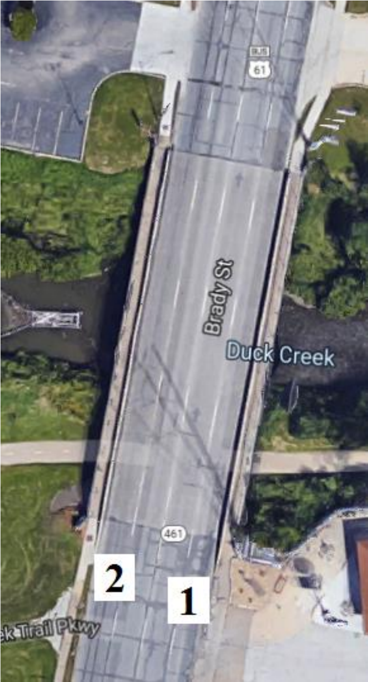
Figure 84. Bridge No. 8220.1R061 [1]
