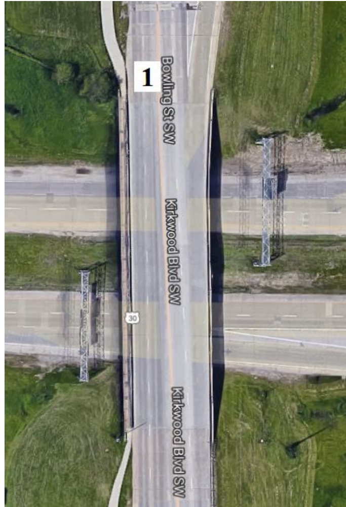
Figure 71. Bridge No. 5753.4O030 [1]
