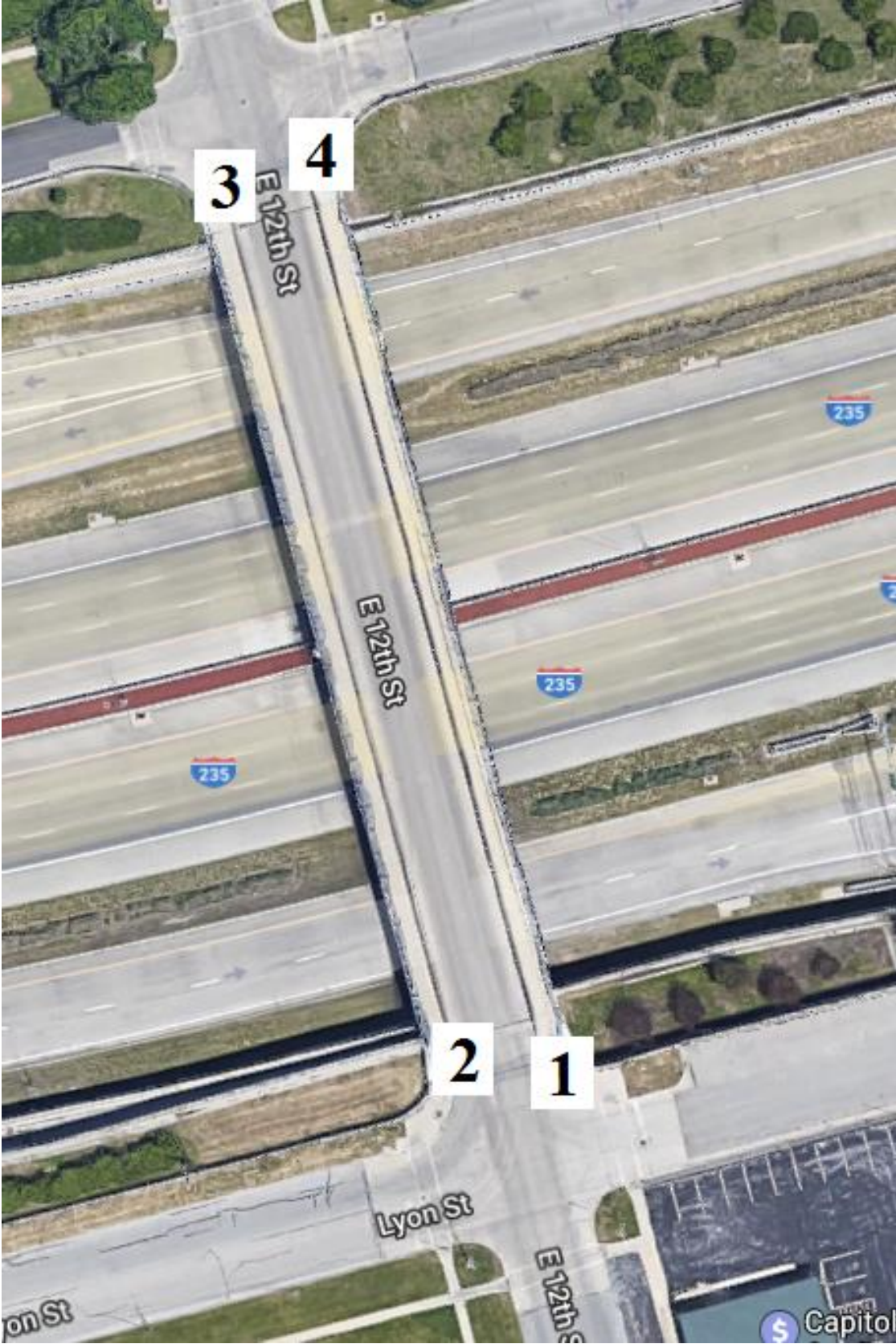
Figure B-134. Bridge No. 7709.1O235 [1]
