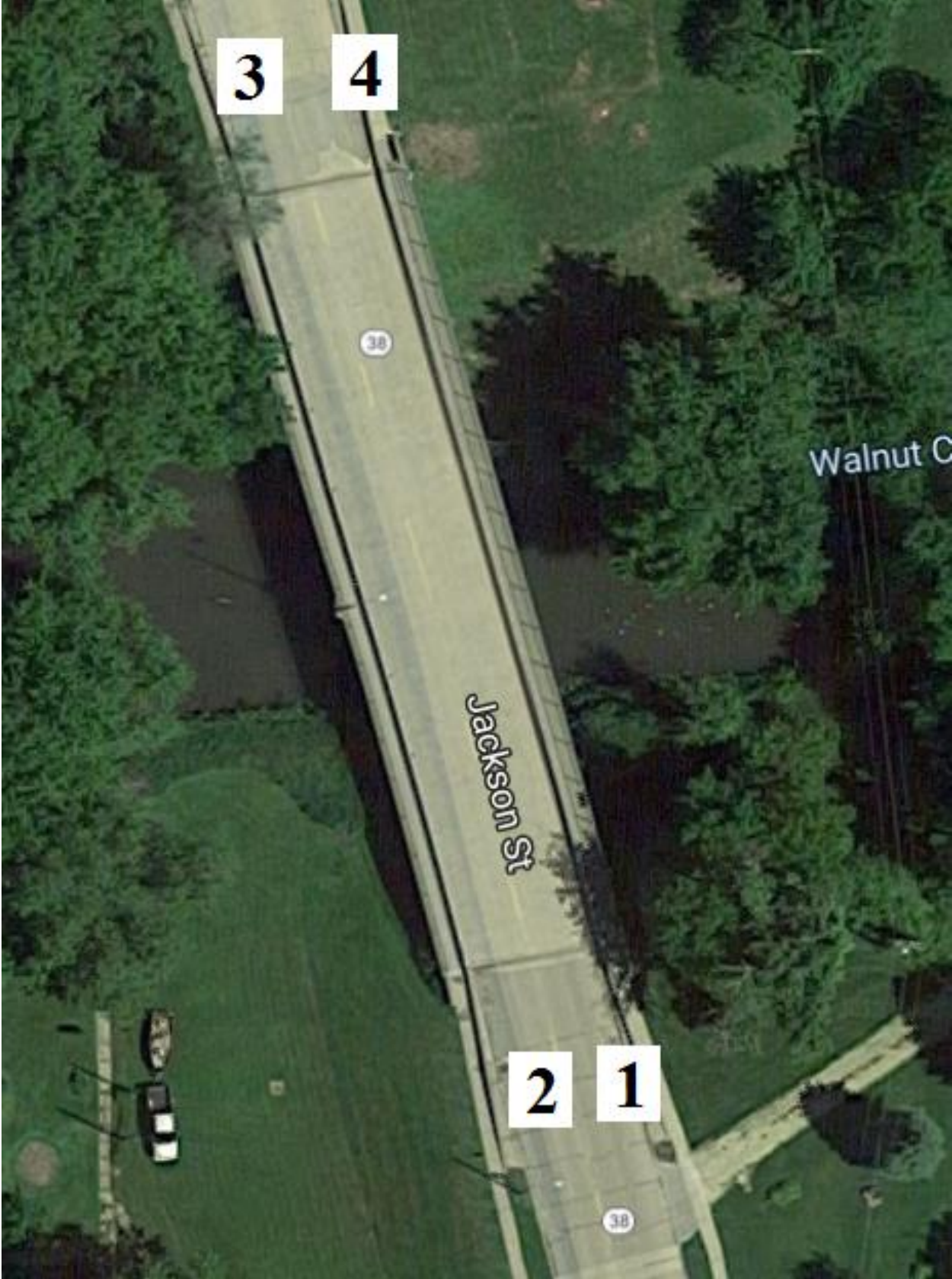
Figure B-86. Bridge No. 5342.8S038 [1]
