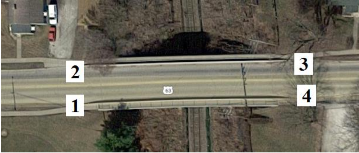
Figure B-105. Bridge No. 6276.0S063 [1]
