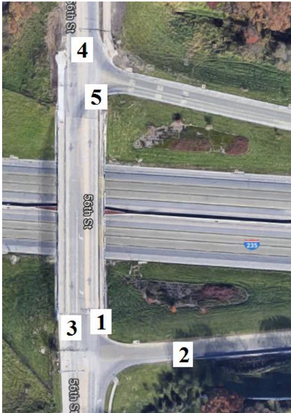
Figure 148. Bridge No. 7704.4O235 with Sloped End Treatments Labeled [1]
