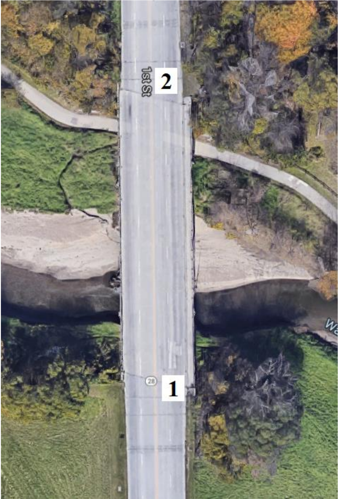
Figure B-136. Bridge No. 7717.8S028 [1]
