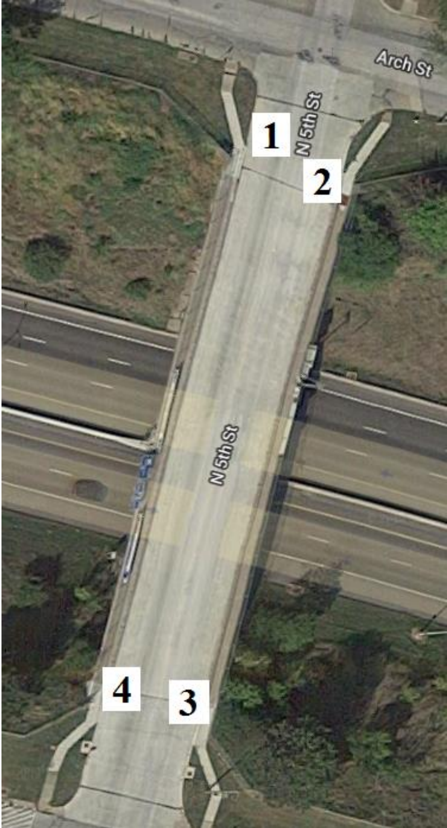
Figure B-44. Bridge No. 2963.20034 [1]
