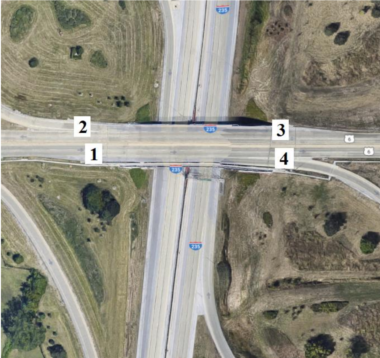
Figure B-144. Bridge No. 7738.9S006 [1]
