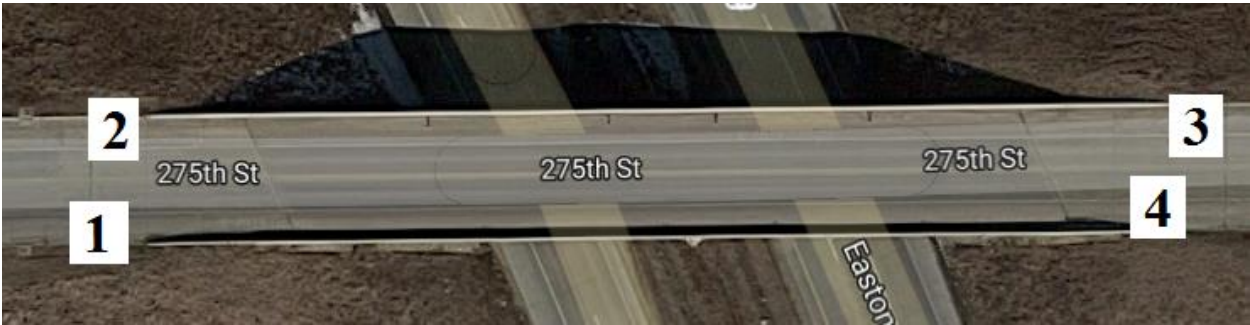
Figure B-15. Bridge No. 0995.4O218 [1]
