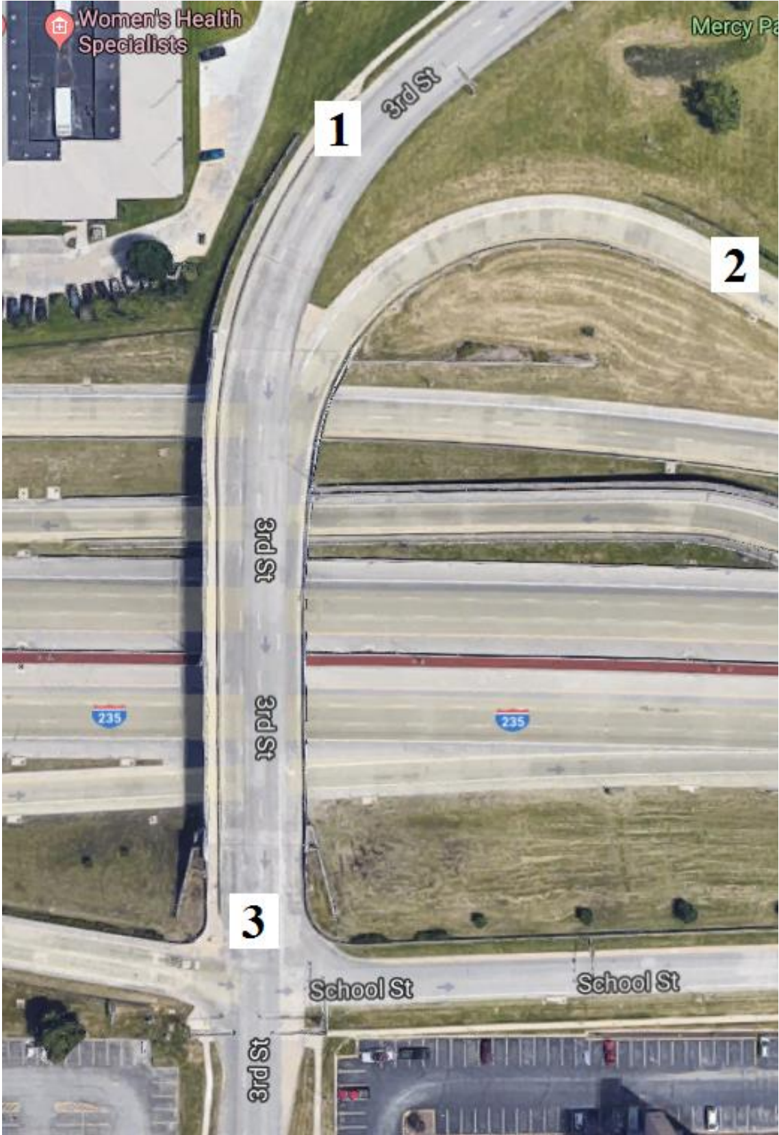
Figure B-129. Bridge No. 7708.2O235 [1]
