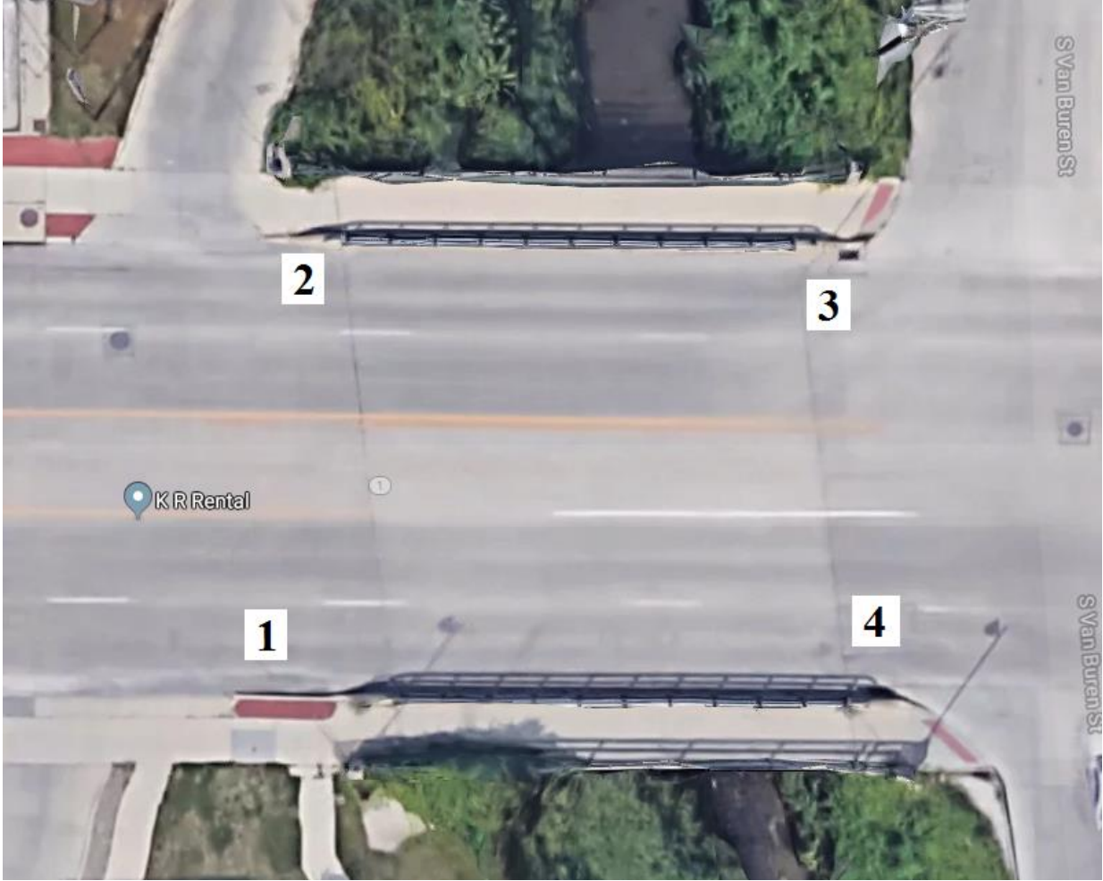
Figure B-82. Bridge No. 5286.5S001 [1]
