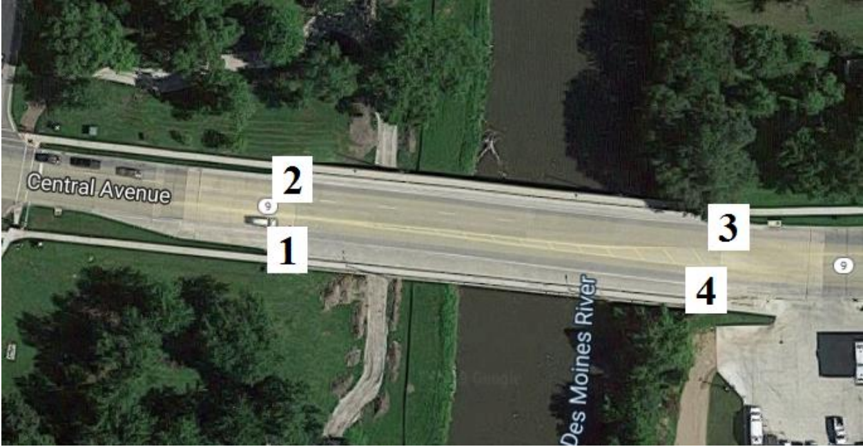
Figure B-57. Bridge No. 3288.1S009 [1]
