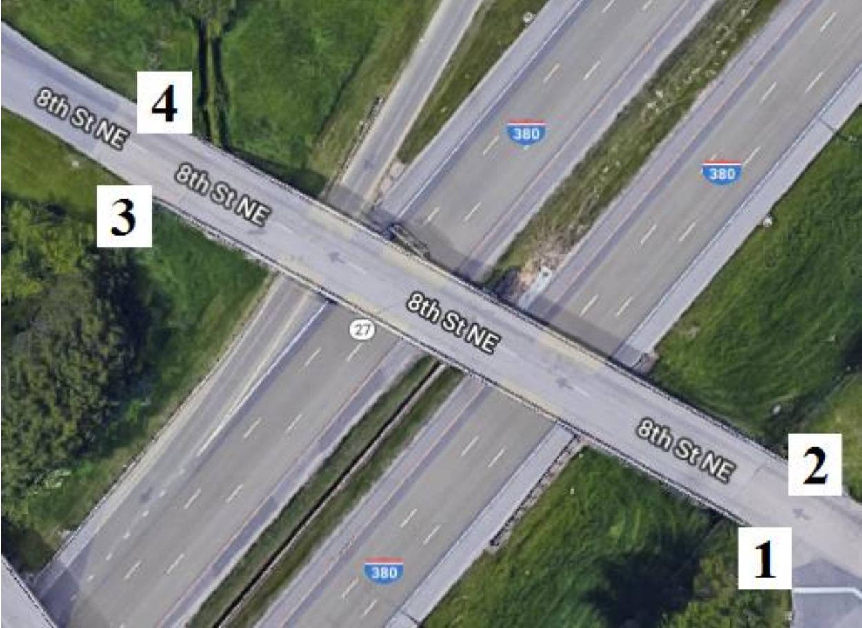
Figure B-93. Bridge No. 5720.8O380 [1]
