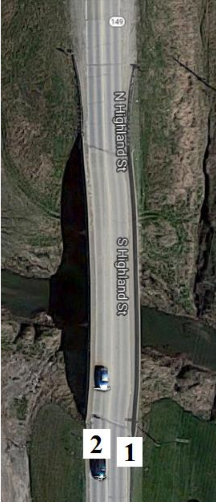
Figure B-71. Bridge No. 4864.8S149 [1]
