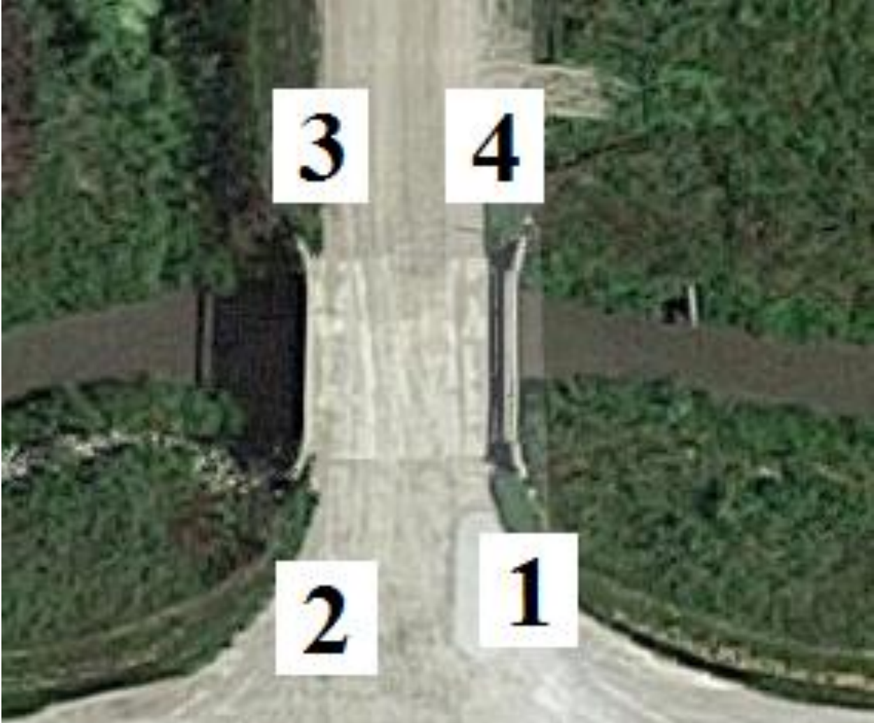
Figure B-110. Bridge No. 7403.2A018 [1]
