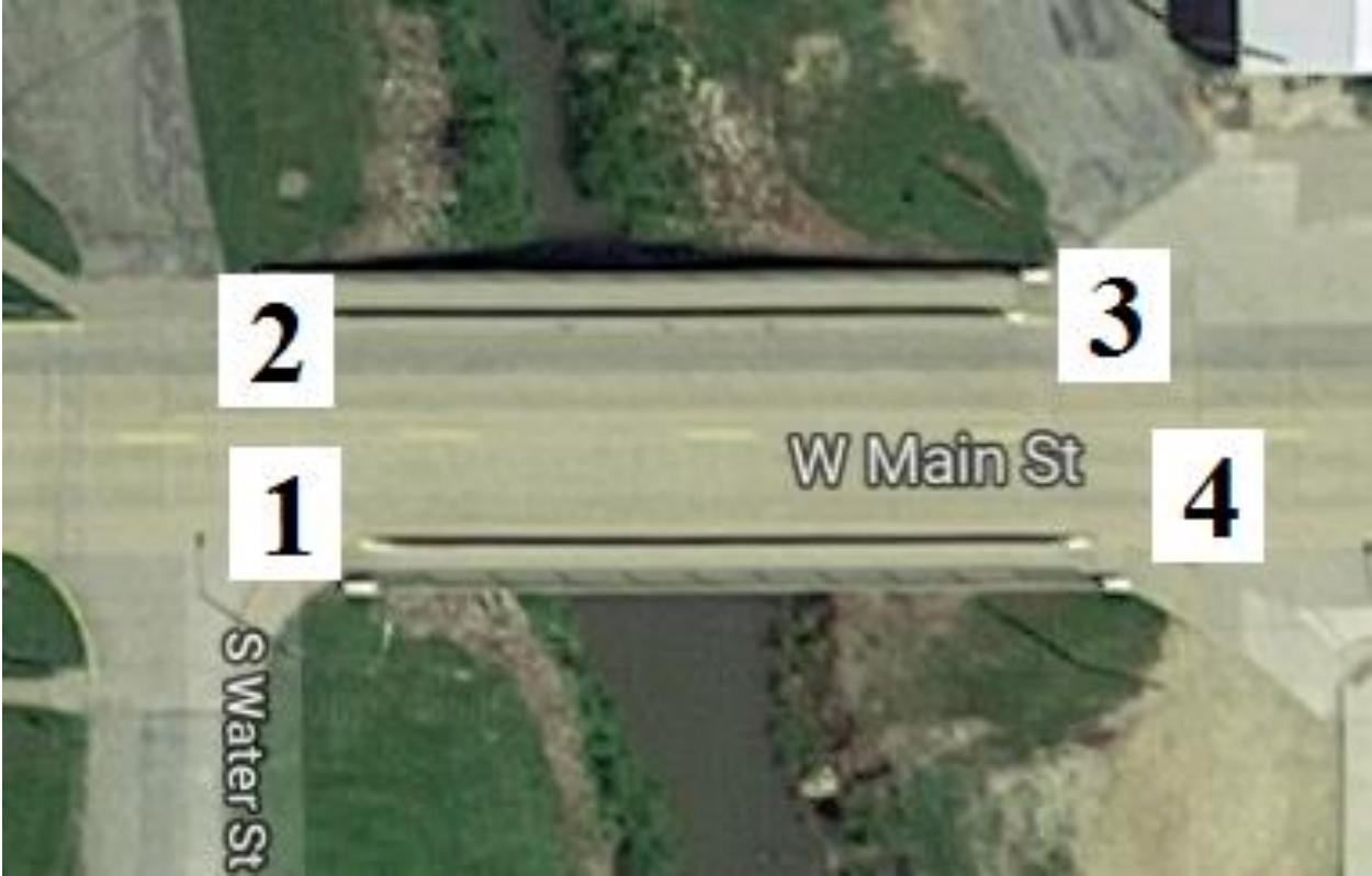
Figure B-85. Bridge No. 5314.8S064 [1]
