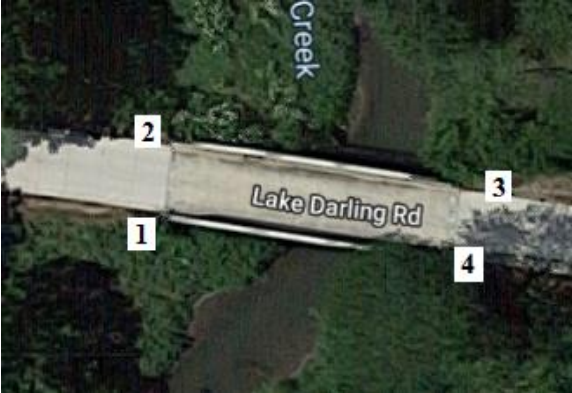
Figure B-171. Bridge No. 9200.4S612 [1]
