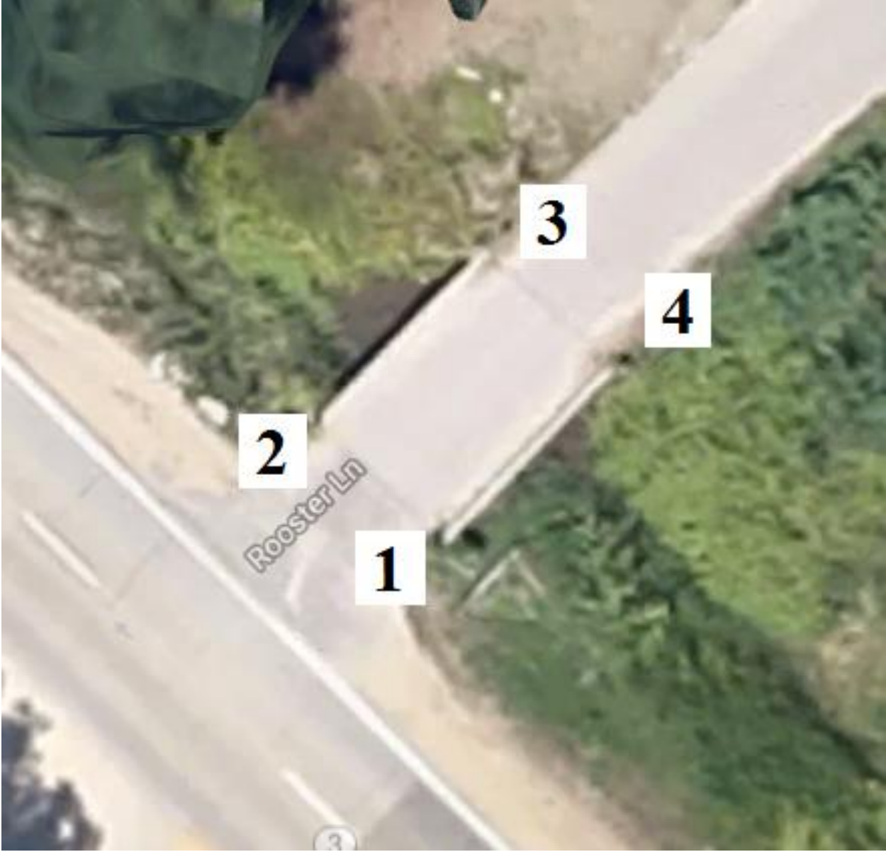
Figure B-54. Bridge No. 3150.7A052 [1]
