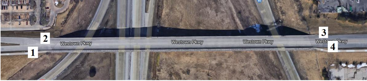
Figure B-139. Bridge No. 7723.8O080 [1]
