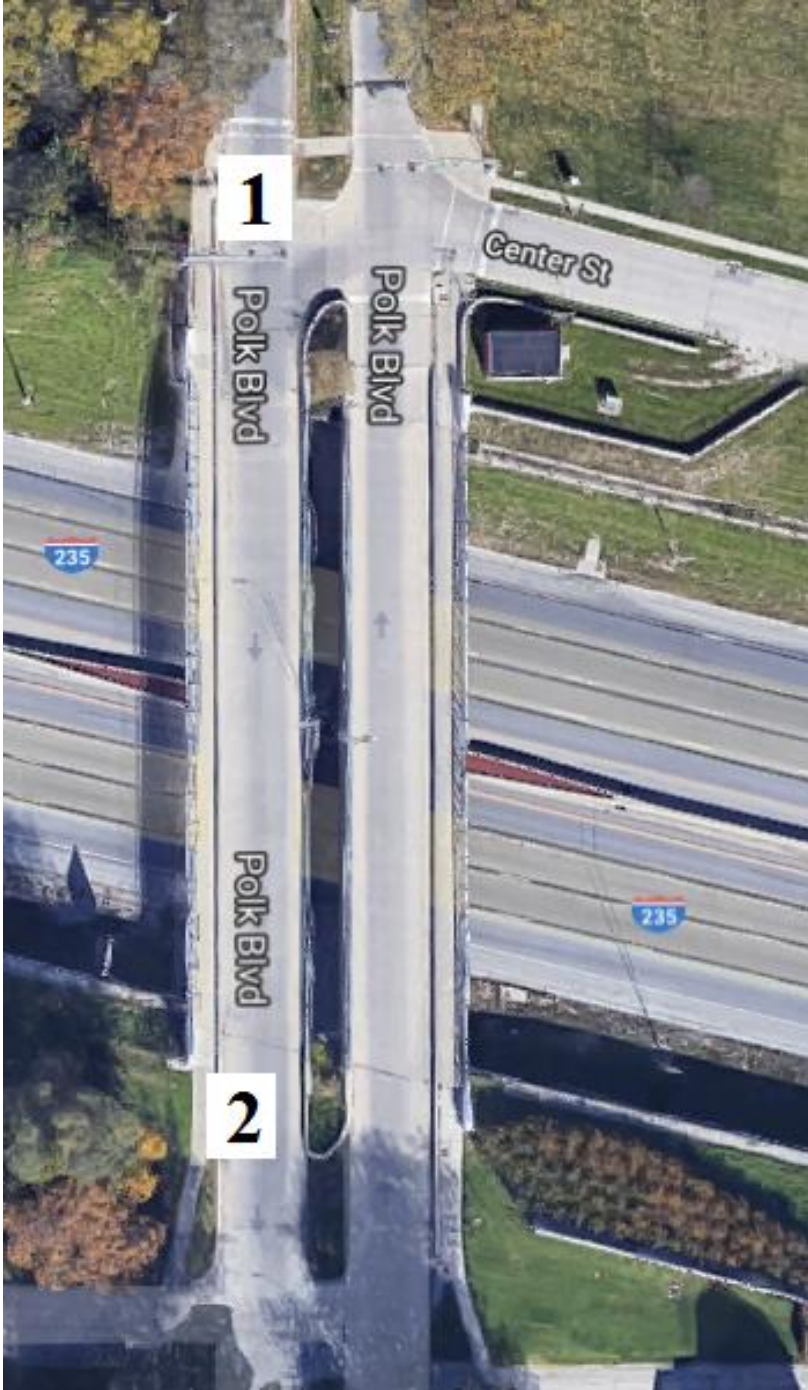
Figure 159. Bridge No. 7705.00235 with Sloped End Treatments Labeled [1]
