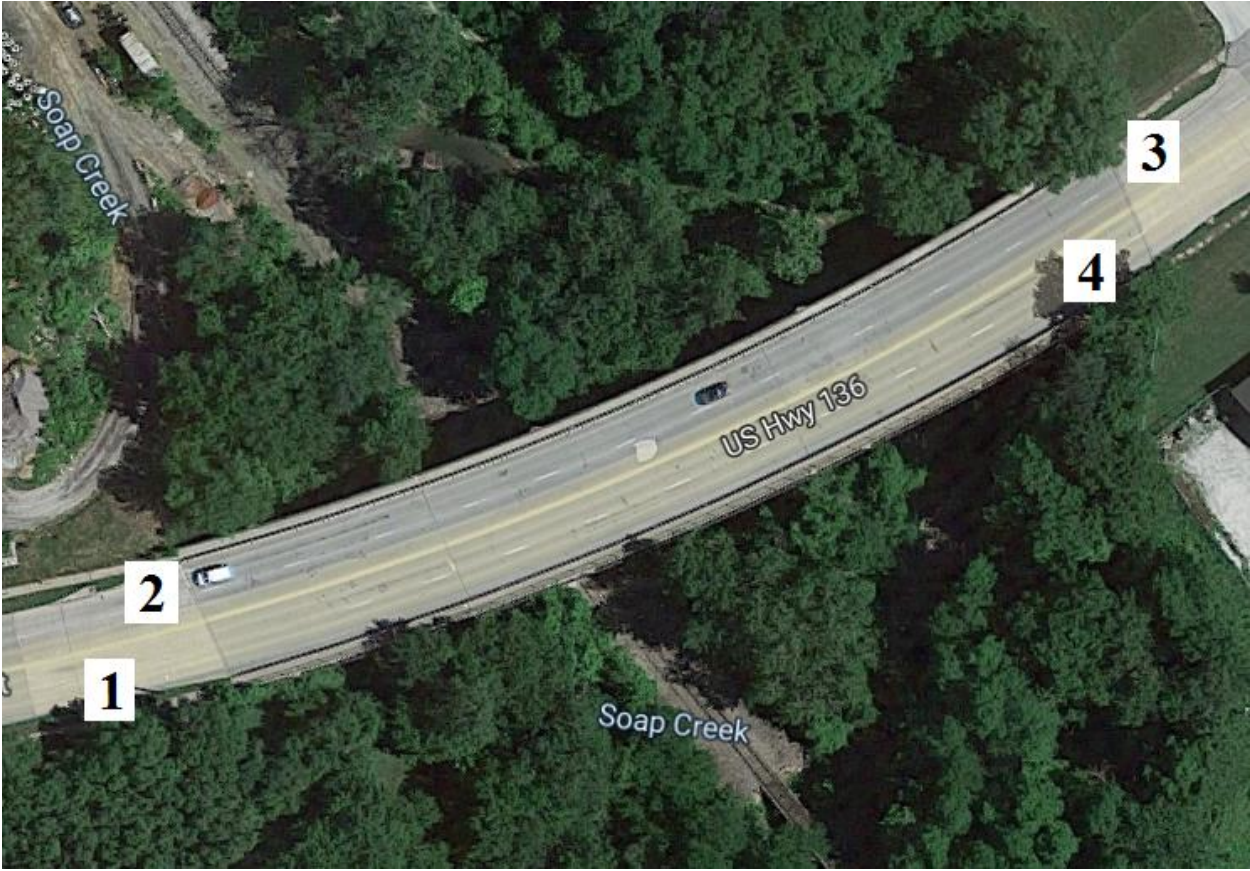
Figure B-89. Bridge No. 5602.4S136 [1]
