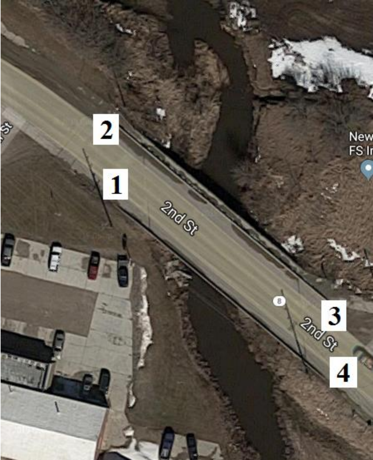
Figure B-164. Bridge No. 8600.5S008 [1]
