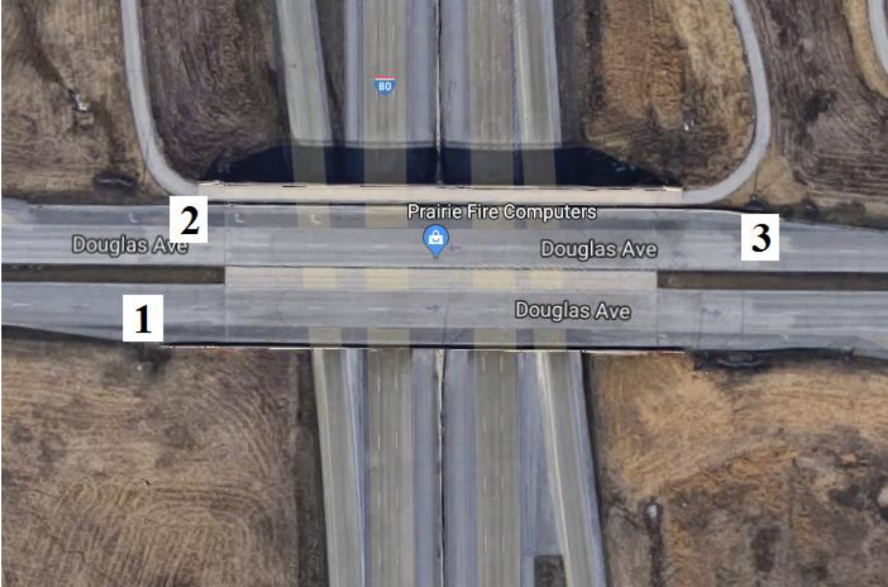
Figure B-141. Bridge No. 7726.1O080 [1]
