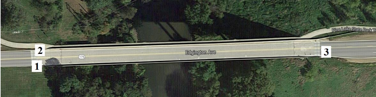
Figure B-68. Bridge No. 4287.7S175 [1]
