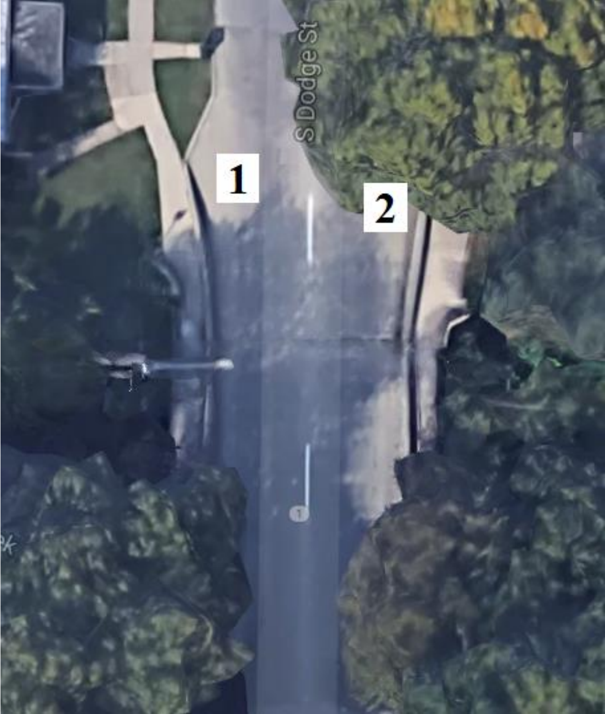
Figure B-83. Bridge No. 5286.9L001 [1]
