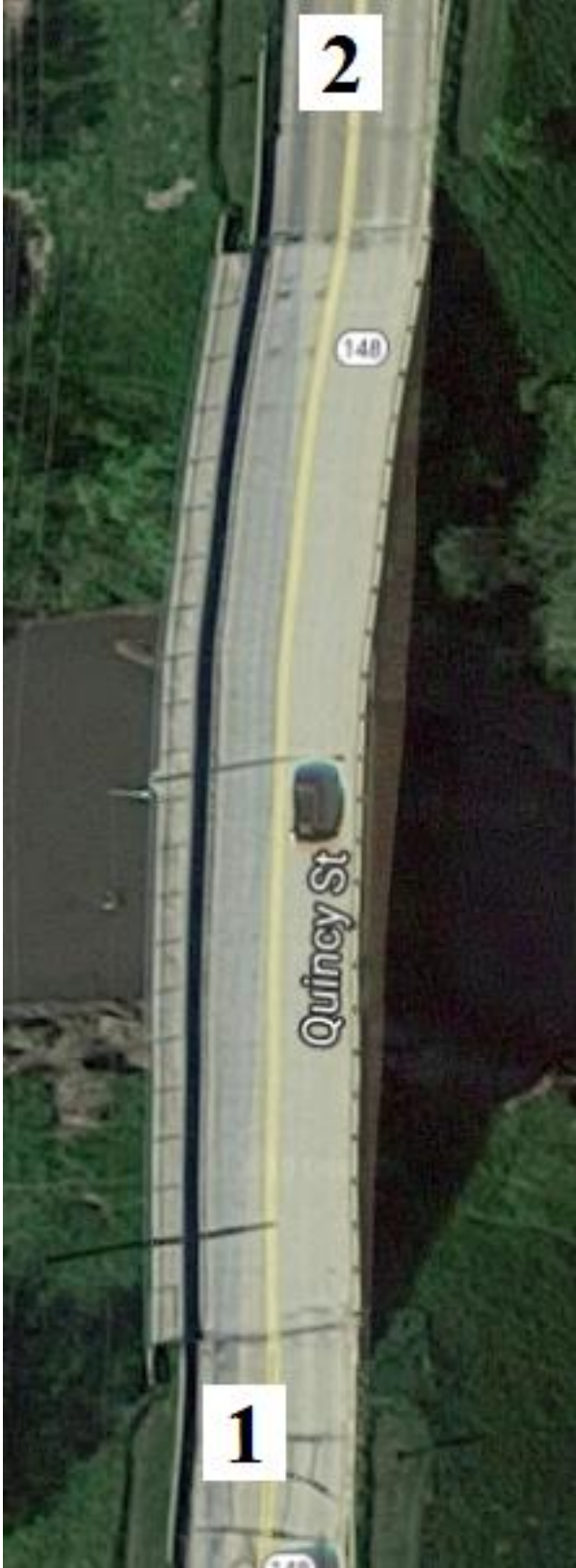
Figure B-1. Bridge No. 0230.3S148 [1]
