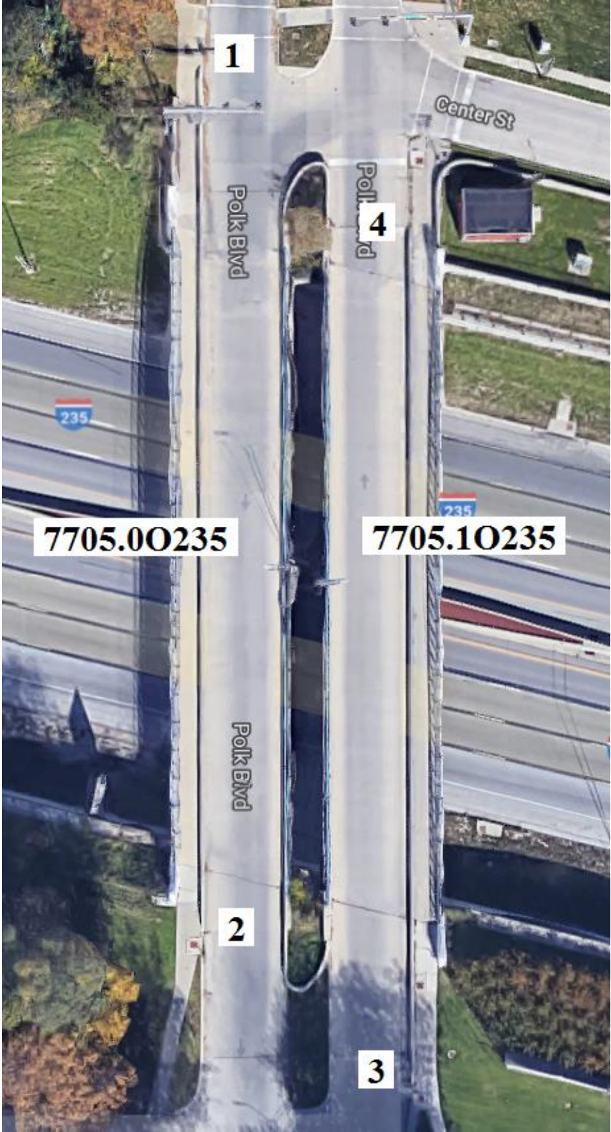
Figure 96. Bridge Nos. 7705.00235 and 7705.10235 [1]
