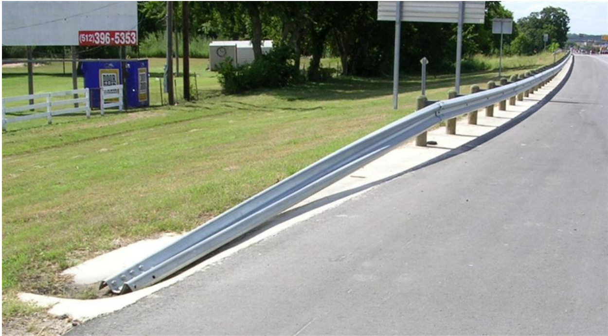
Figure 4. Guardrail Turn-Down [16]
