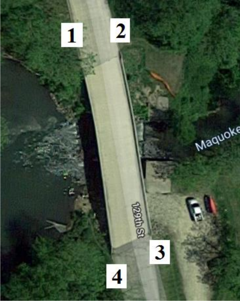
Figure B-37. Bridge No. 2803.8S603 [1]
