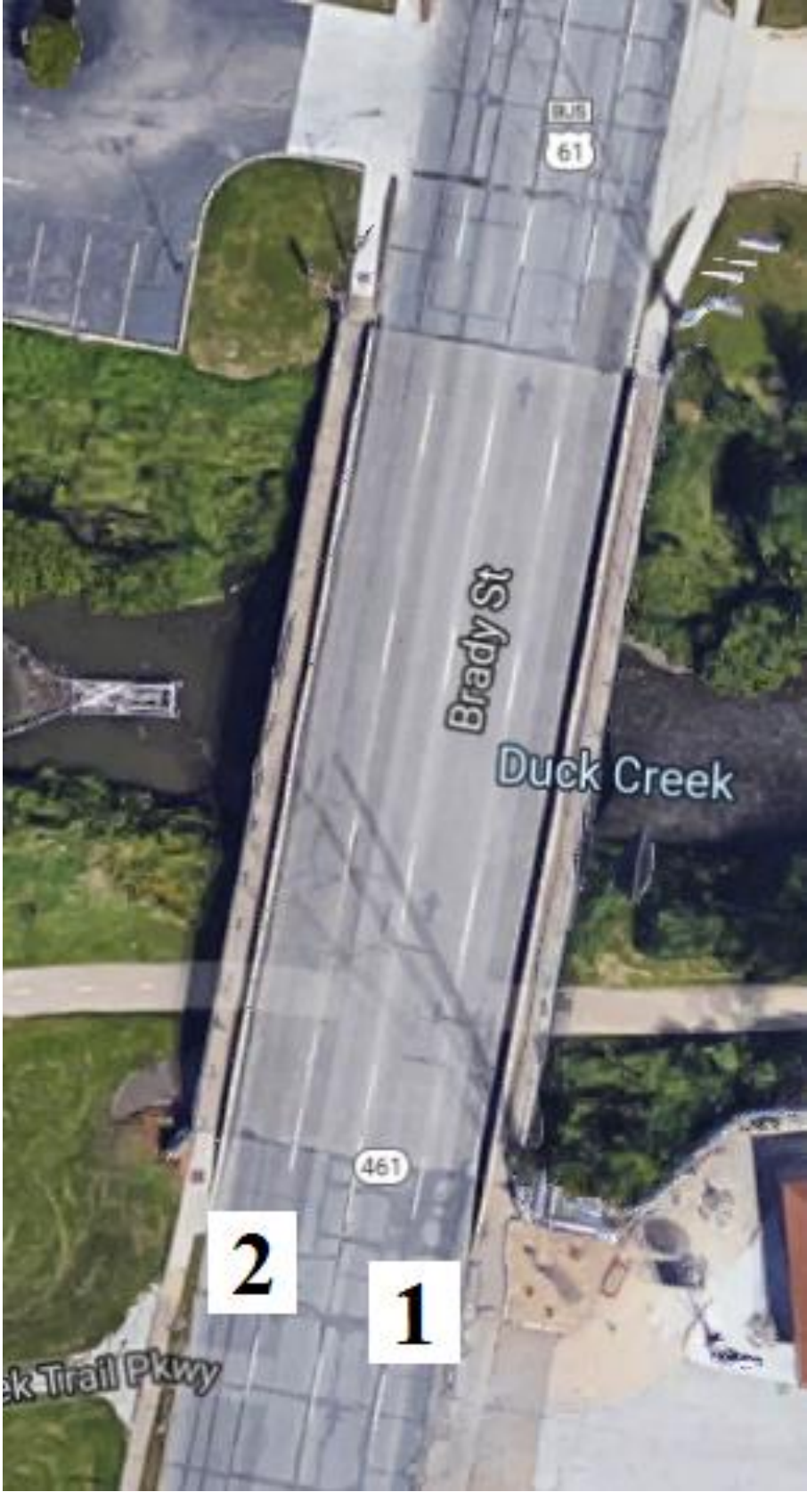
Figure B-156. Bridge No. 8220.1R061 [1]
