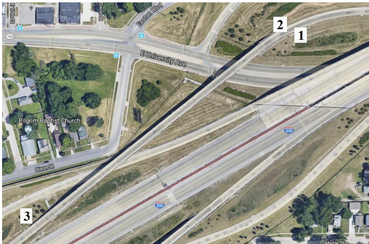
Figure 161. Bridge No. 7710.0A235 with Sloped End Treatments Labeled [1]
