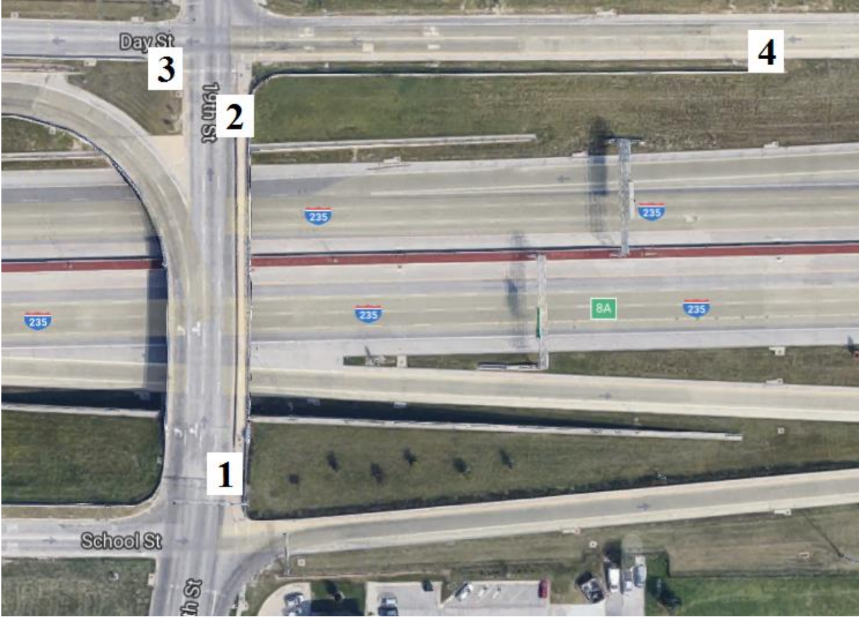
Figure B-125. Bridge No. 7707.2O235 [1]
