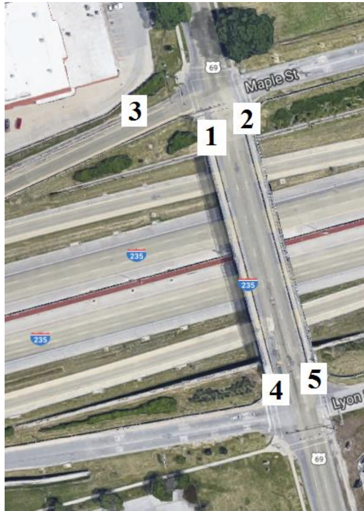
Figure 92. Bridge No. 7785.5S069 [1]
