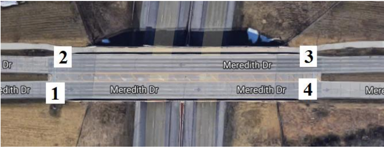
Figure B-142. Bridge No. 7727.1O080 [1]
