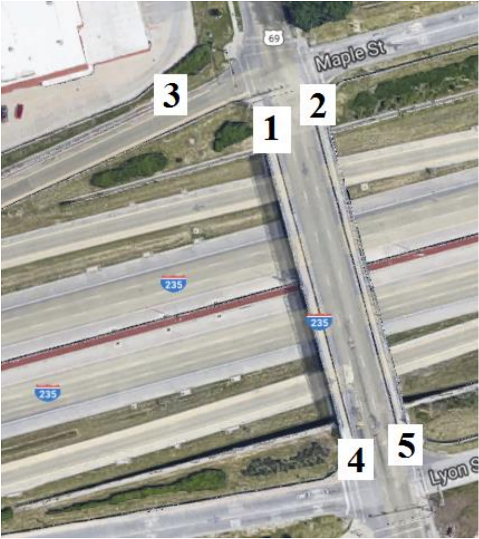
Figure 162. Bridge No. 7785.5S069 with Sloped End Treatments Labeled [1]
