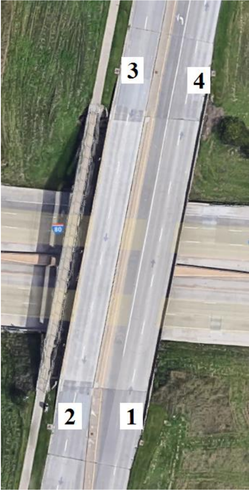
Figure B-77. Bridge No. 5243.00080 [1]
