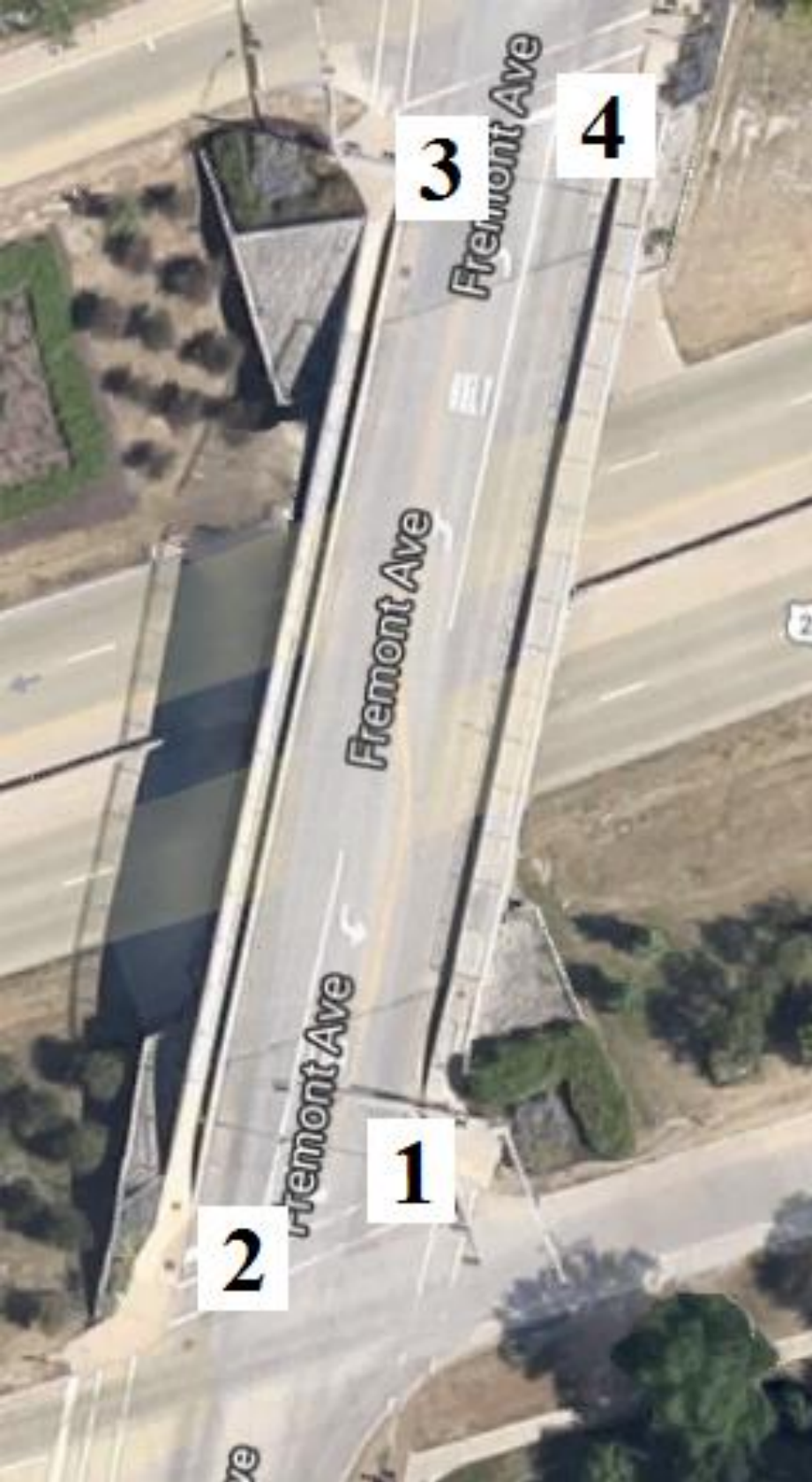
Figure B-49. Bridge No. 3118.4O020 [1]
