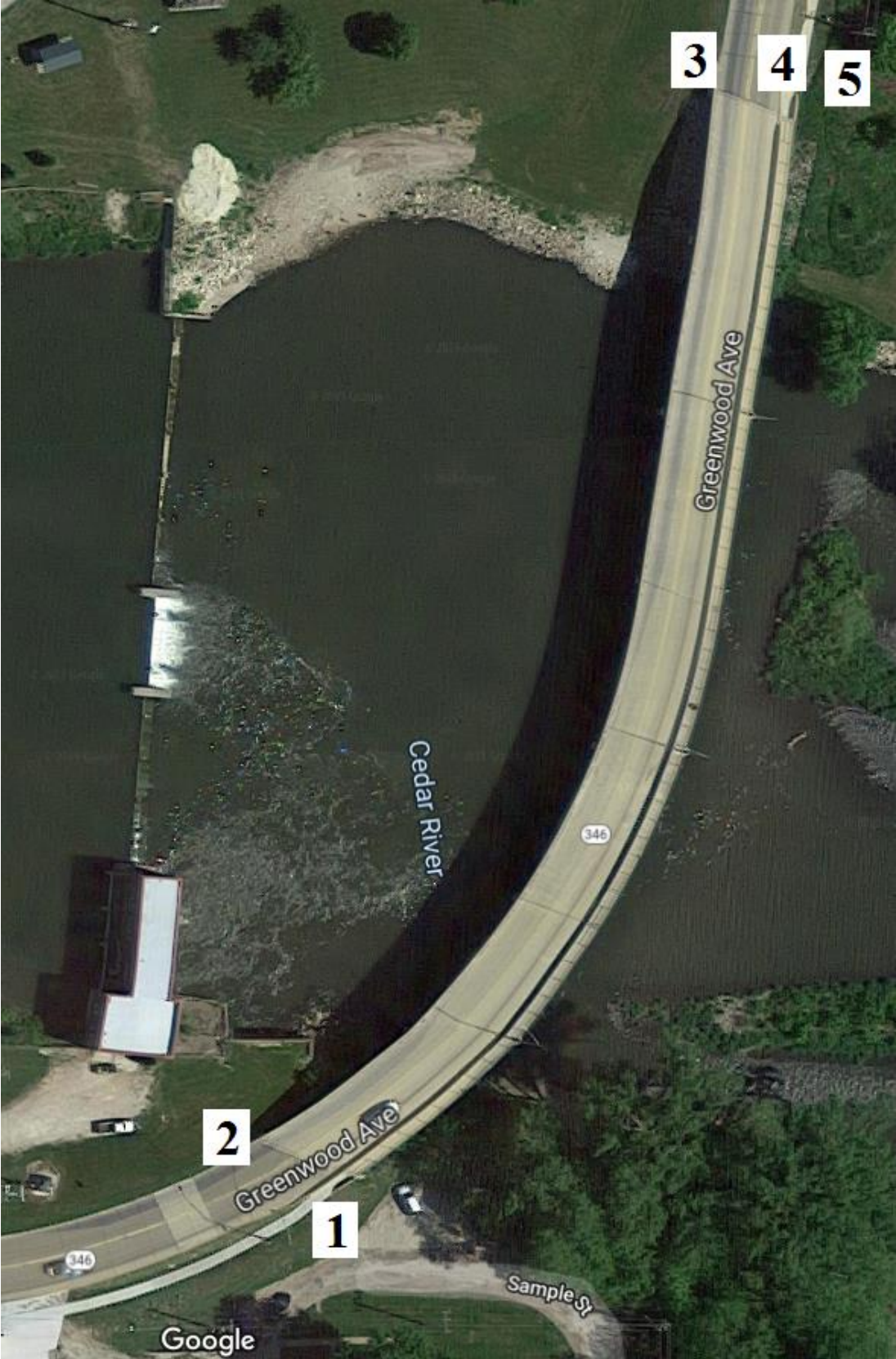
Figure B-27. Bridge No. 1900.5S346 [1]
