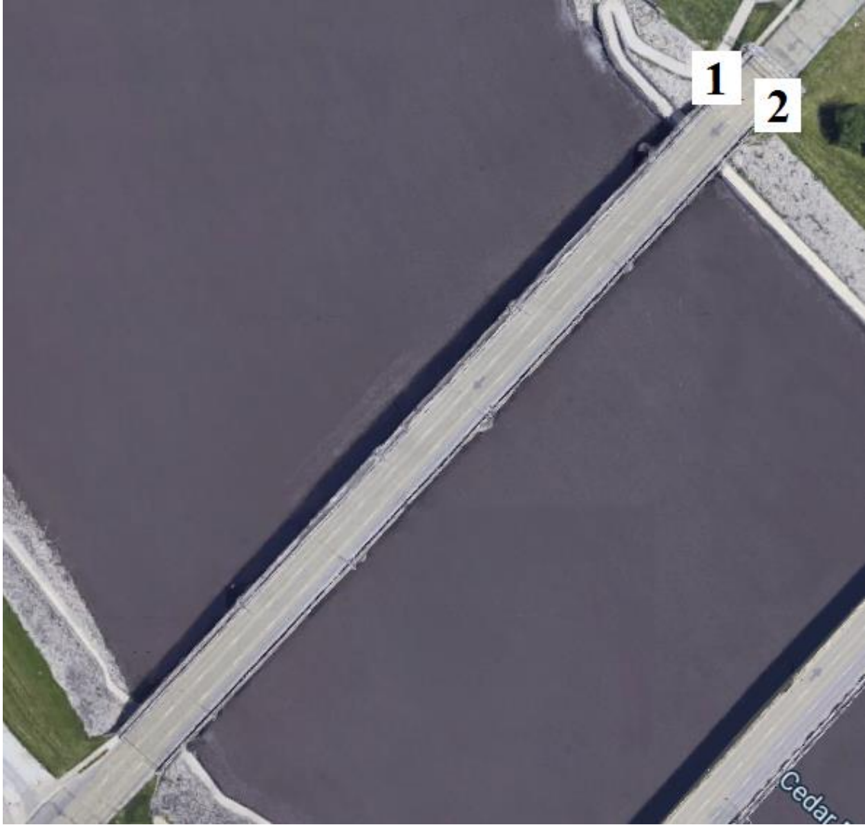
Figure B-11. Bridge No. 0763.1L063 [1]
