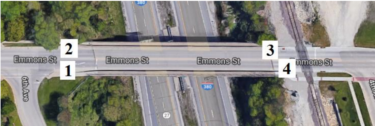
Figure B-97. Bridge No. 5724.7O380 [1]
