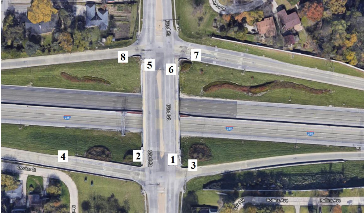
Figure 79. Bridge No. 7718.3S028 [1]
