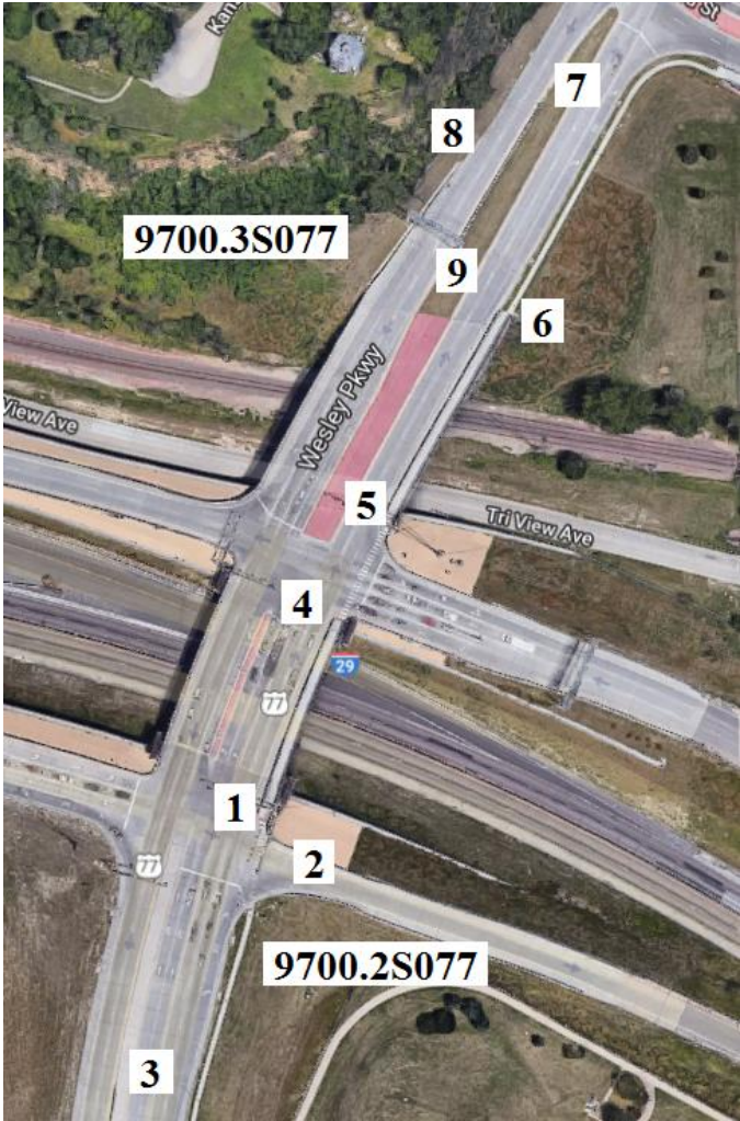
Figure 97. Bridge Nos. 9700.2S077 and 9700.3S077 [1]
