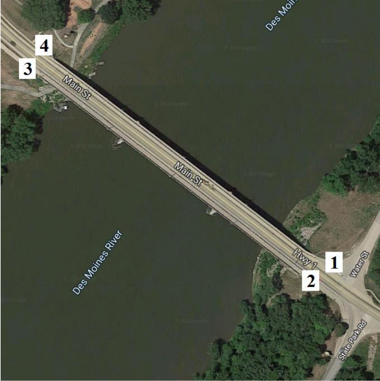
Figure B-168. Bridge No. 8903.8S001 [1]
