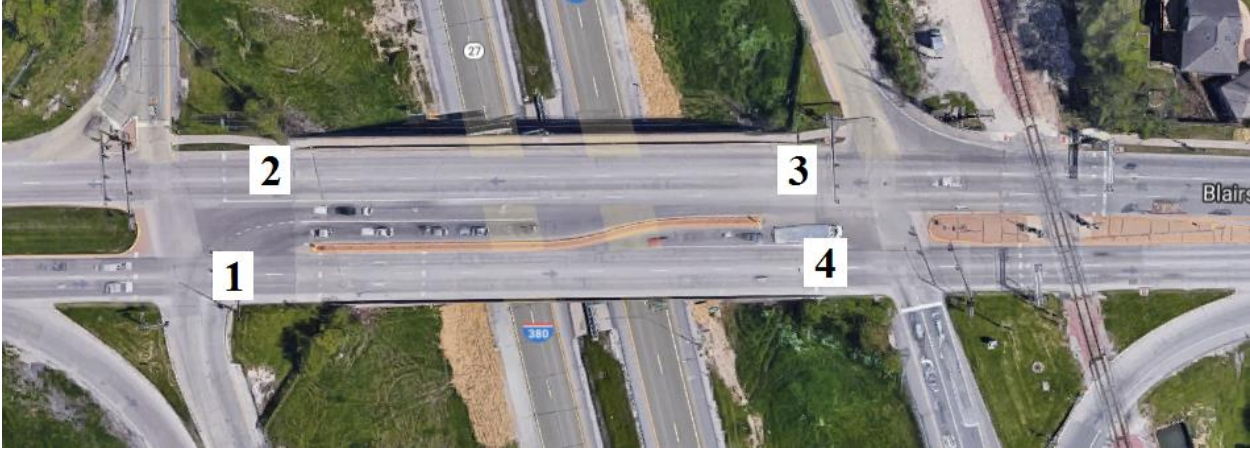
Figure B-96. Bridge No. 5724.4O380 [1]
