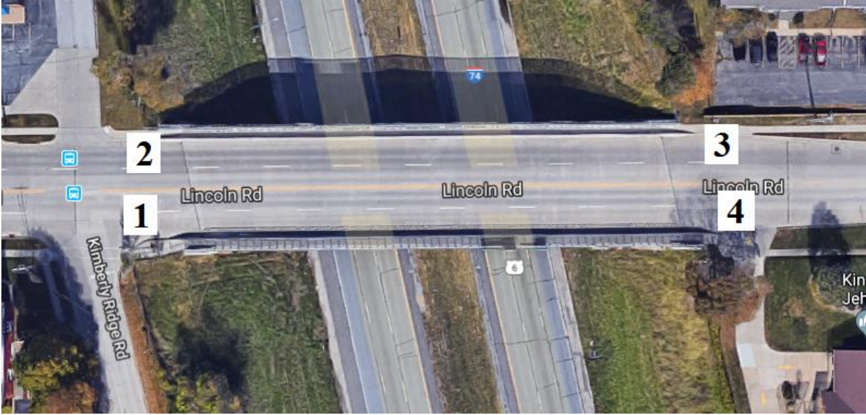
Figure B-151. Bridge No. 8203.8O074 [1]
