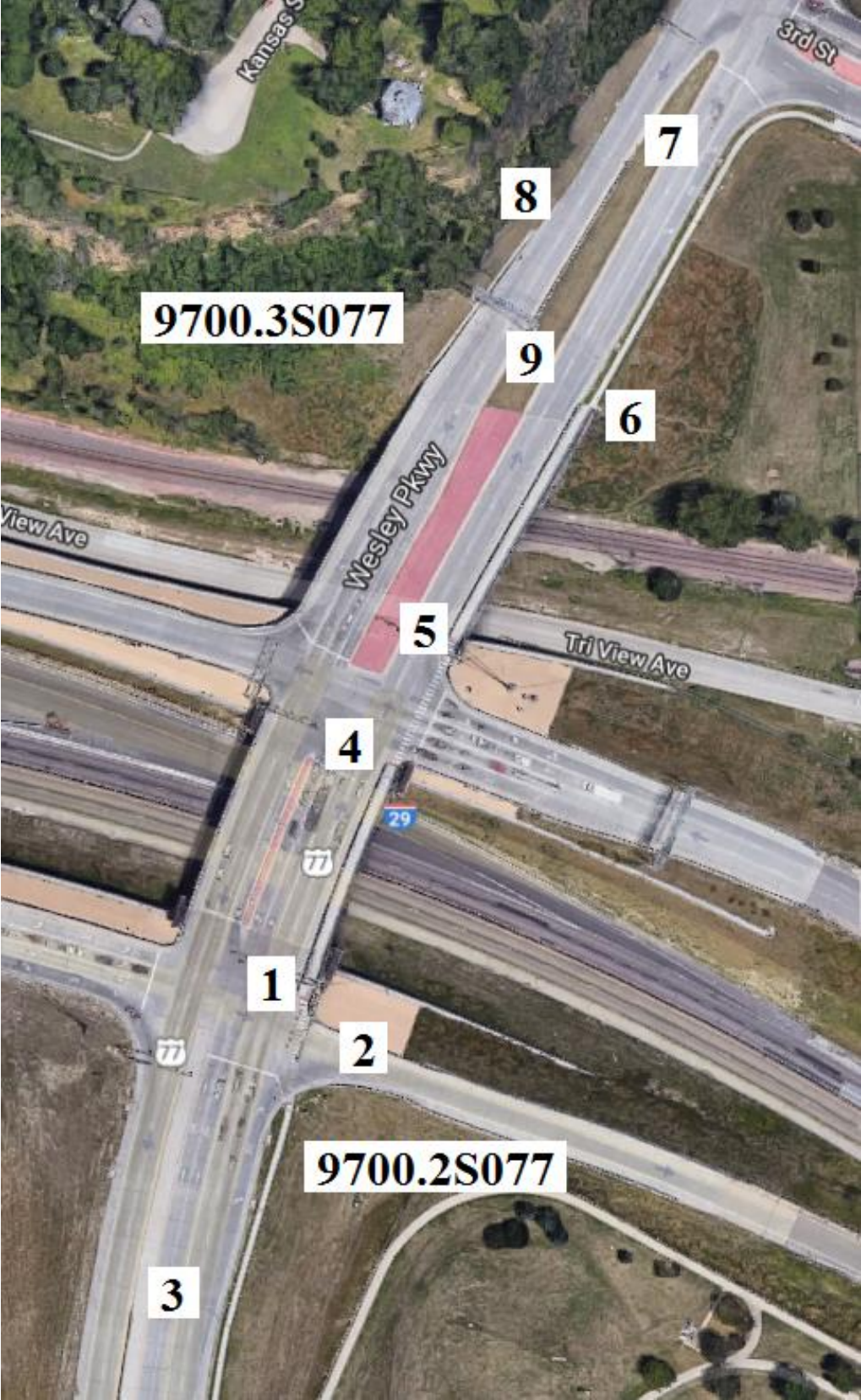
Figure B-178. Bridge Nos. 9700.2S077 and 9700.3S077[1]
