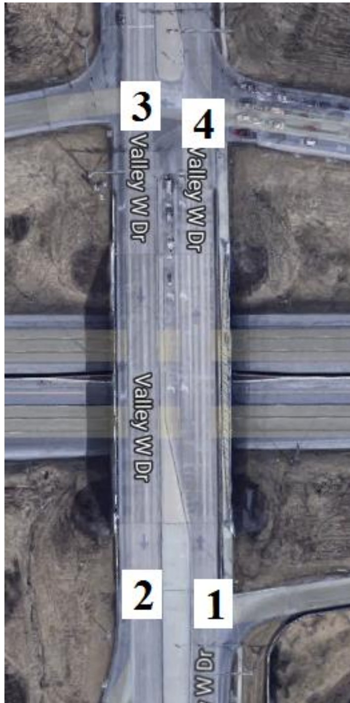
Figure 147. Bridge No. 7701.3O235 with Sloped End Treatments Labeled [1]
