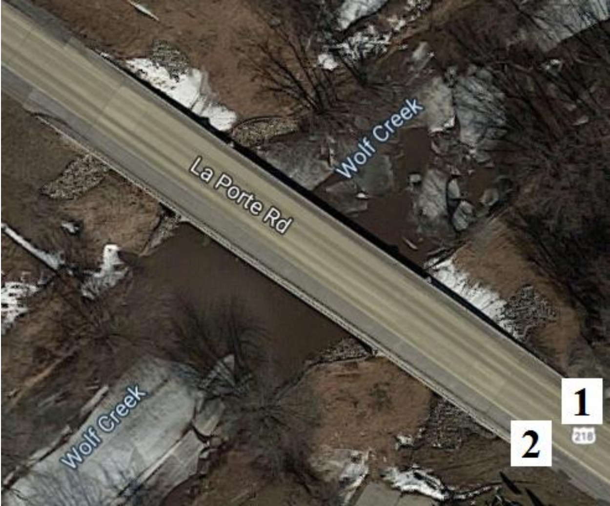
Figure B-13. Bridge No. 0767.1S218 [1]
