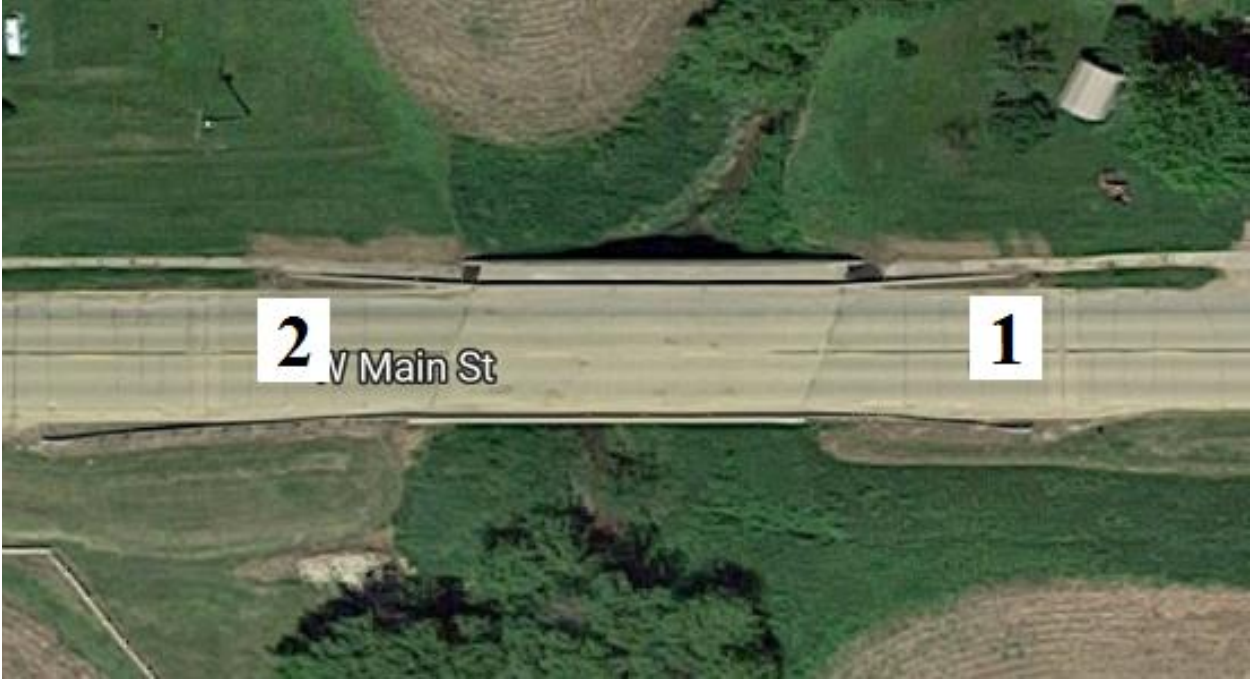
Figure B-72. Bridge No. 4922.0S064 [1]
