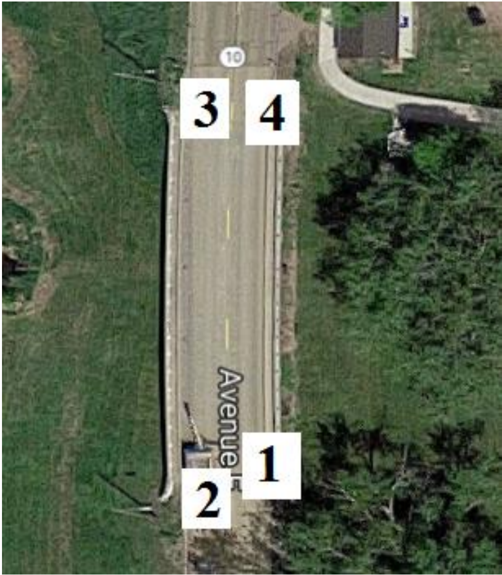
Figure B-158. Bridge No. 8403.4S010 [1]
