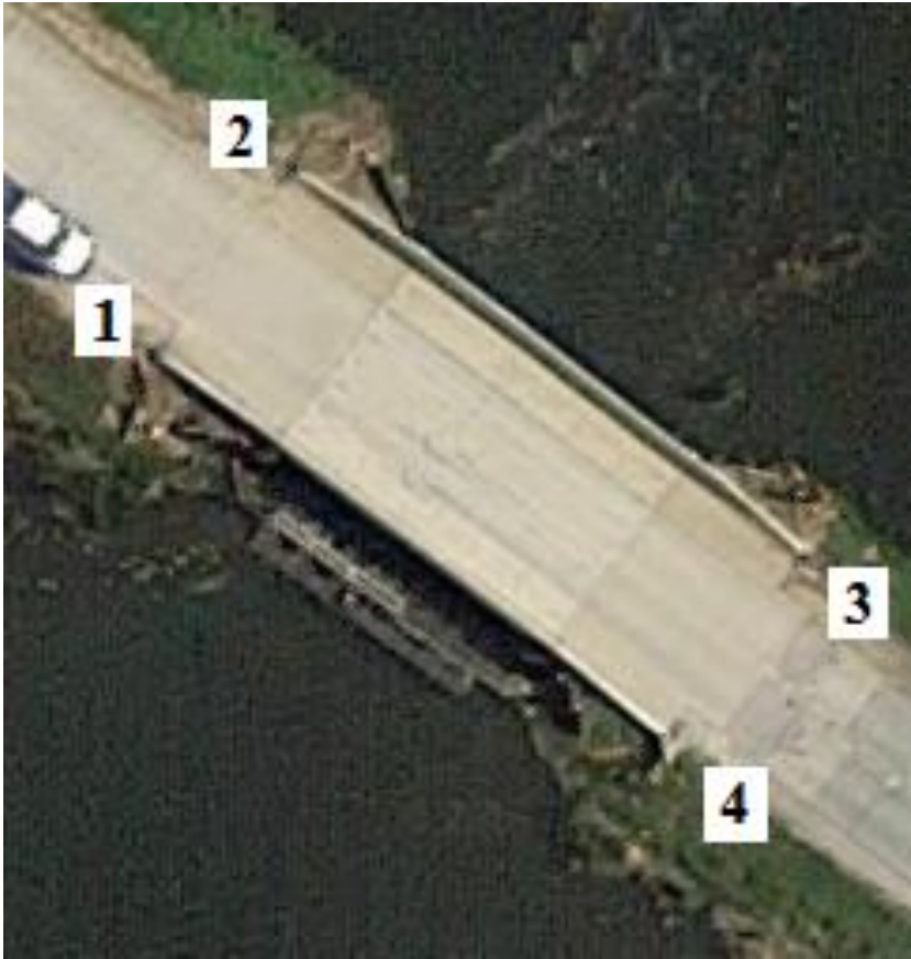
Figure B-150. Bridge No. 8100.3S607 [1]
