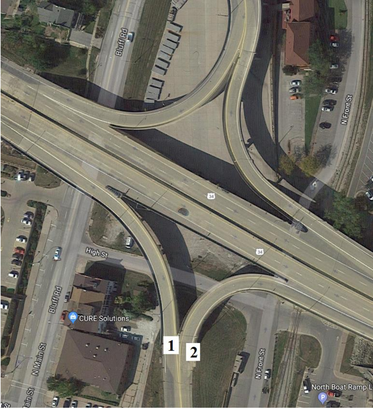
Figure B-46. Bridge No. 2963.7A034 [1]
