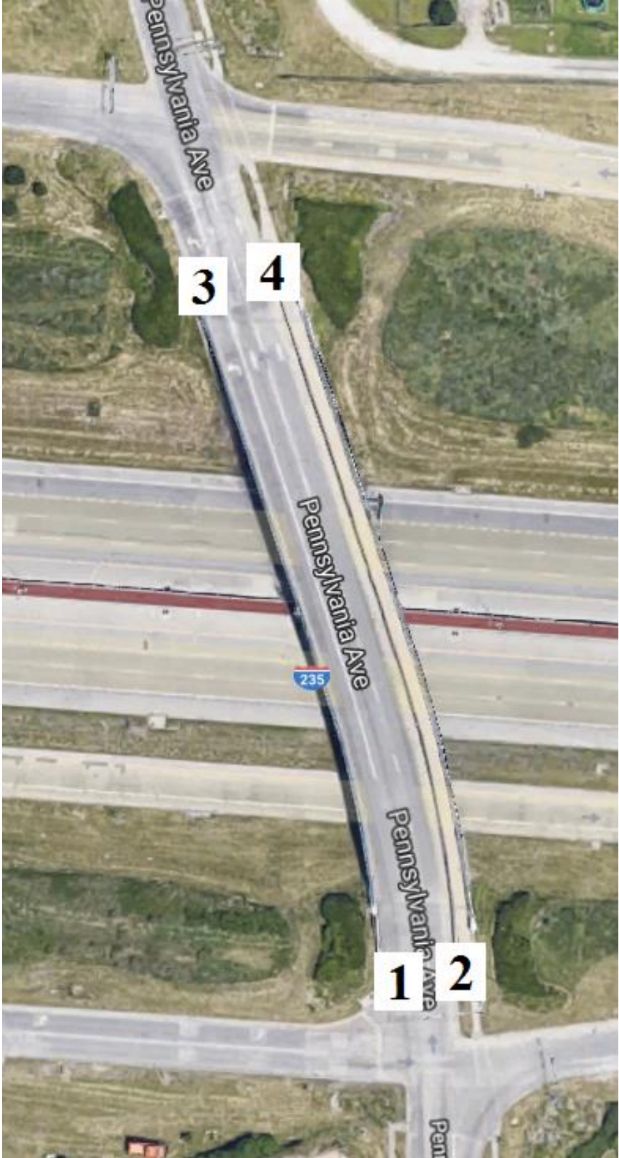
Figure B-132. Bridge No. 7708.9O235 [1]
