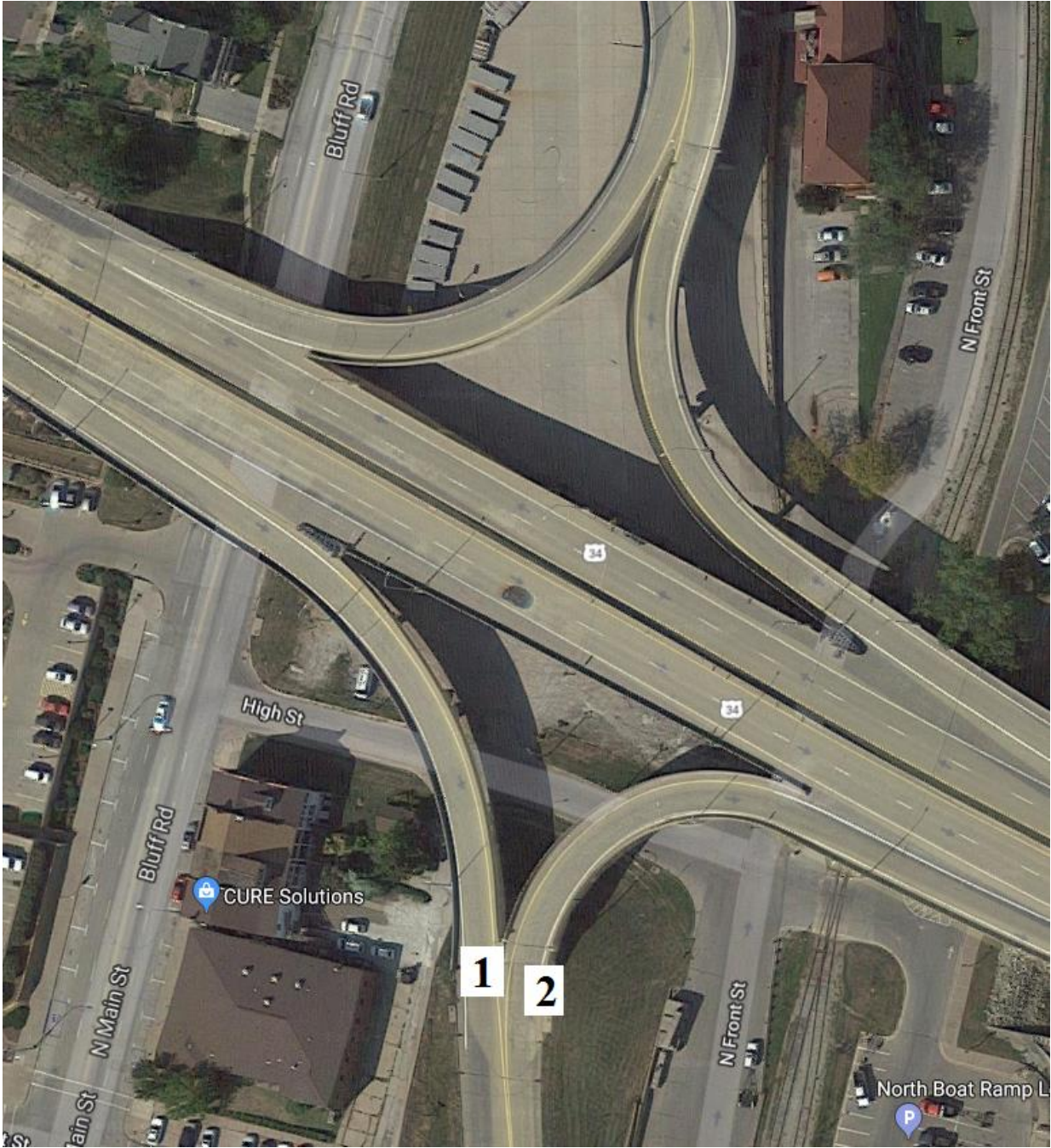
Figure 85. Bridge No. 2963.7A034 [1]
