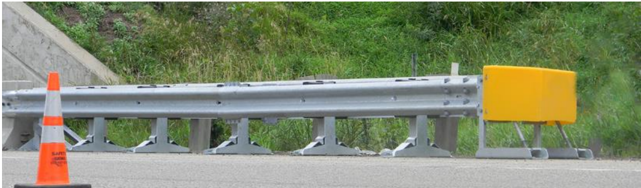
Figure 50. X-TENuator [60]
