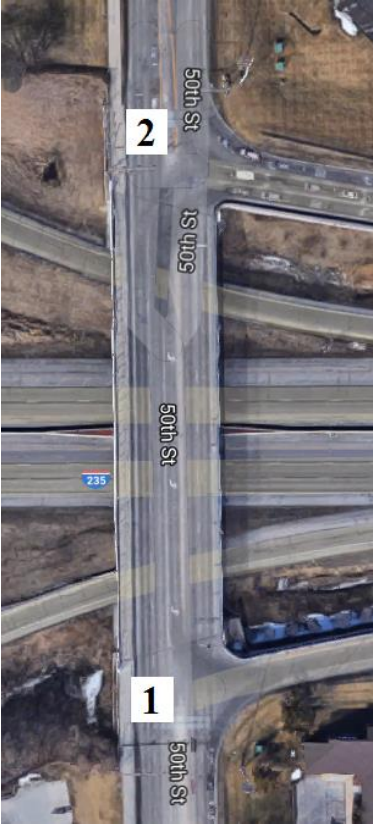
Figure B-114. Bridge No. 7700.3O235 [1]
