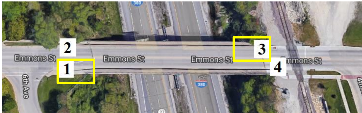
Figure 144. Sloped End Treatments on Bridge with Ramp
