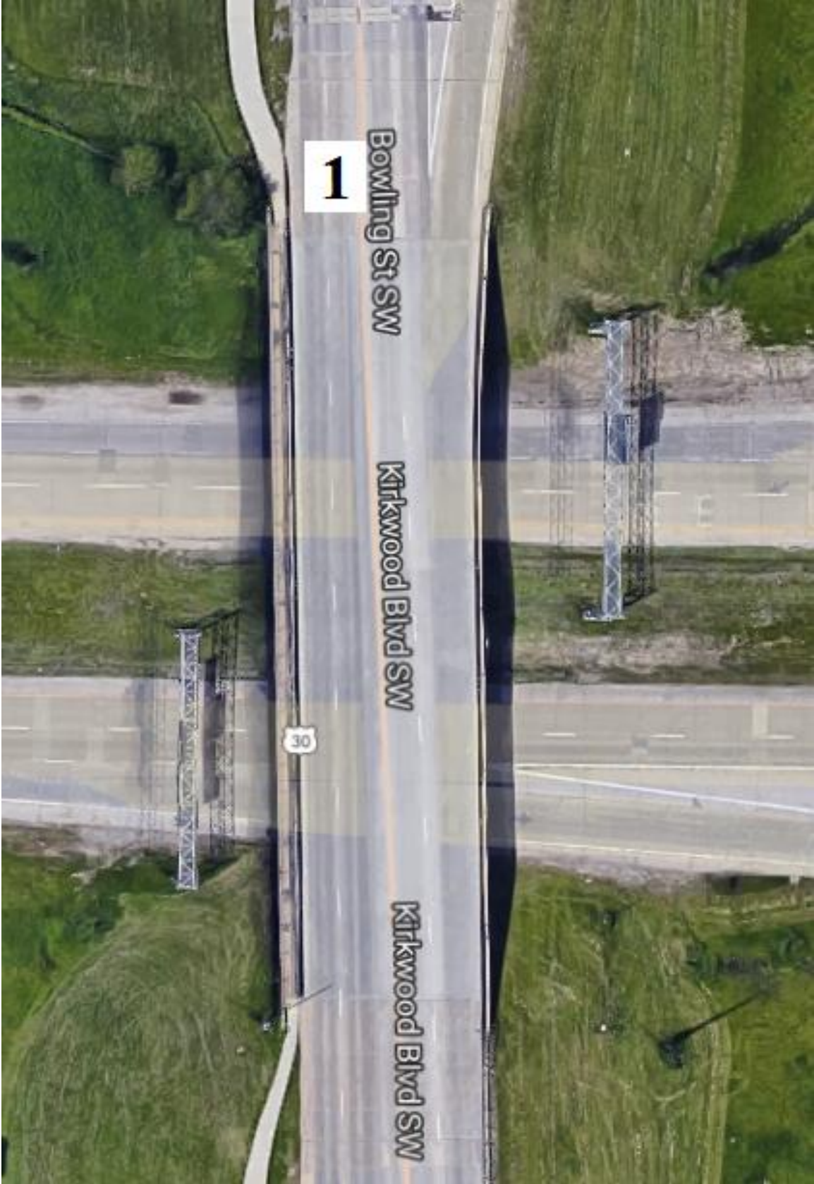
Figure B-100. Bridge No. 5753.4O030 [1]
