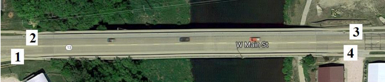
Figure B-38. Bridge No. 2841.6S013 [1]
