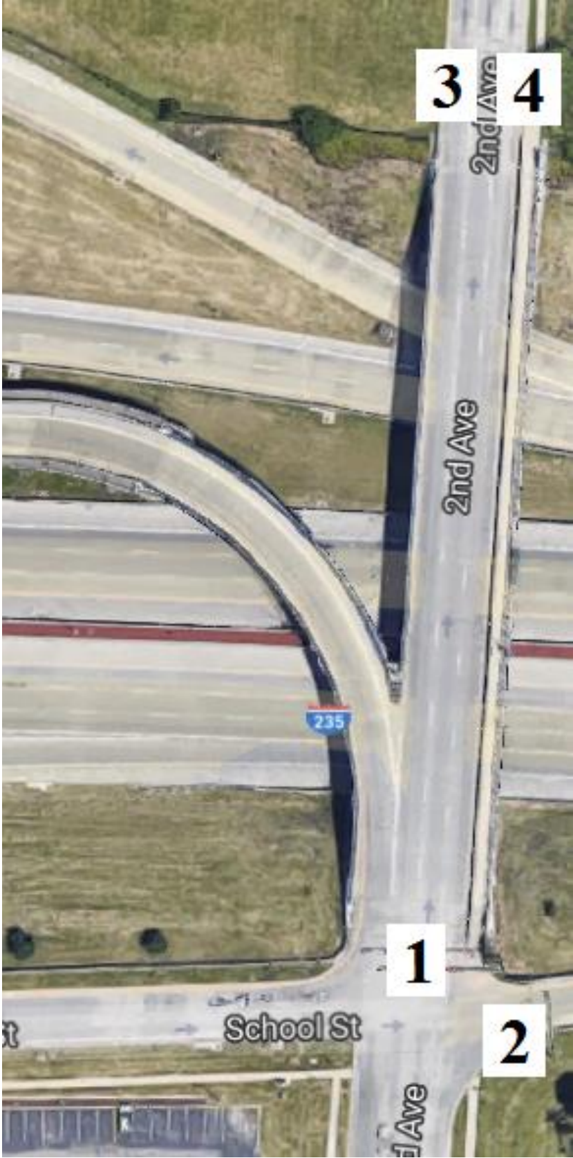
Figure B-130. Bridge No. 7708.3O235 [1]
