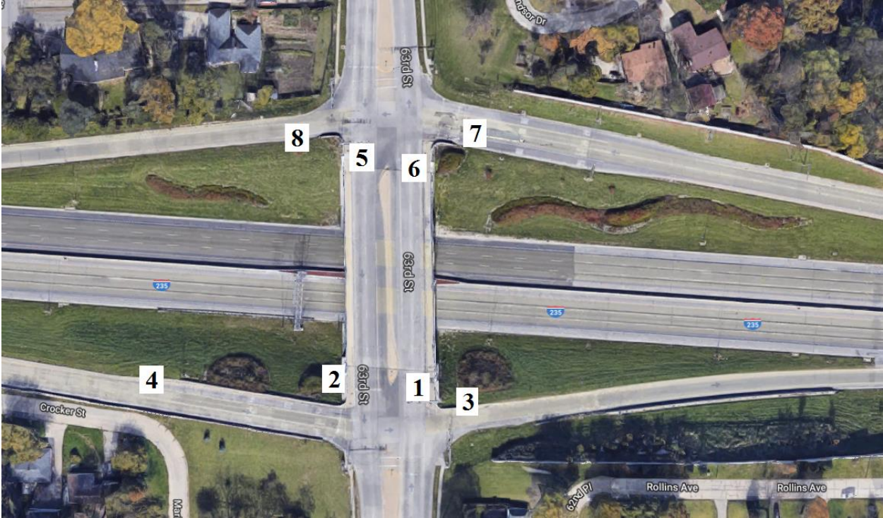
Figure B-137. Bridge No. 7718.3S028 [1]
