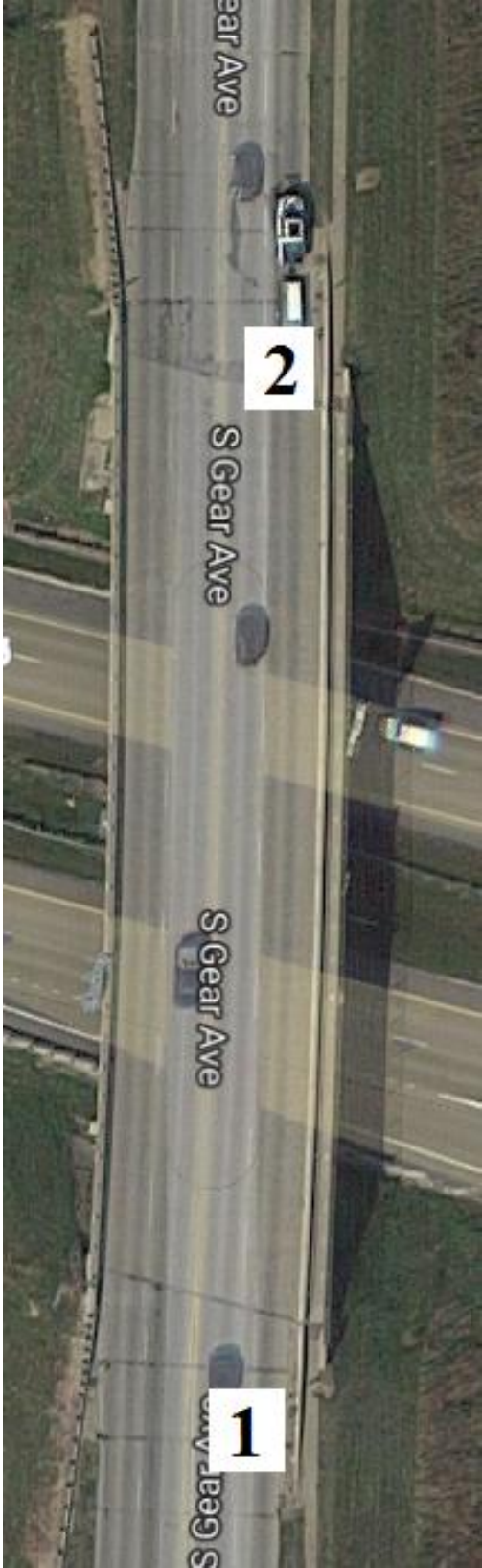
Figure B-40. Bridge No. 2959.6O034 [1]
