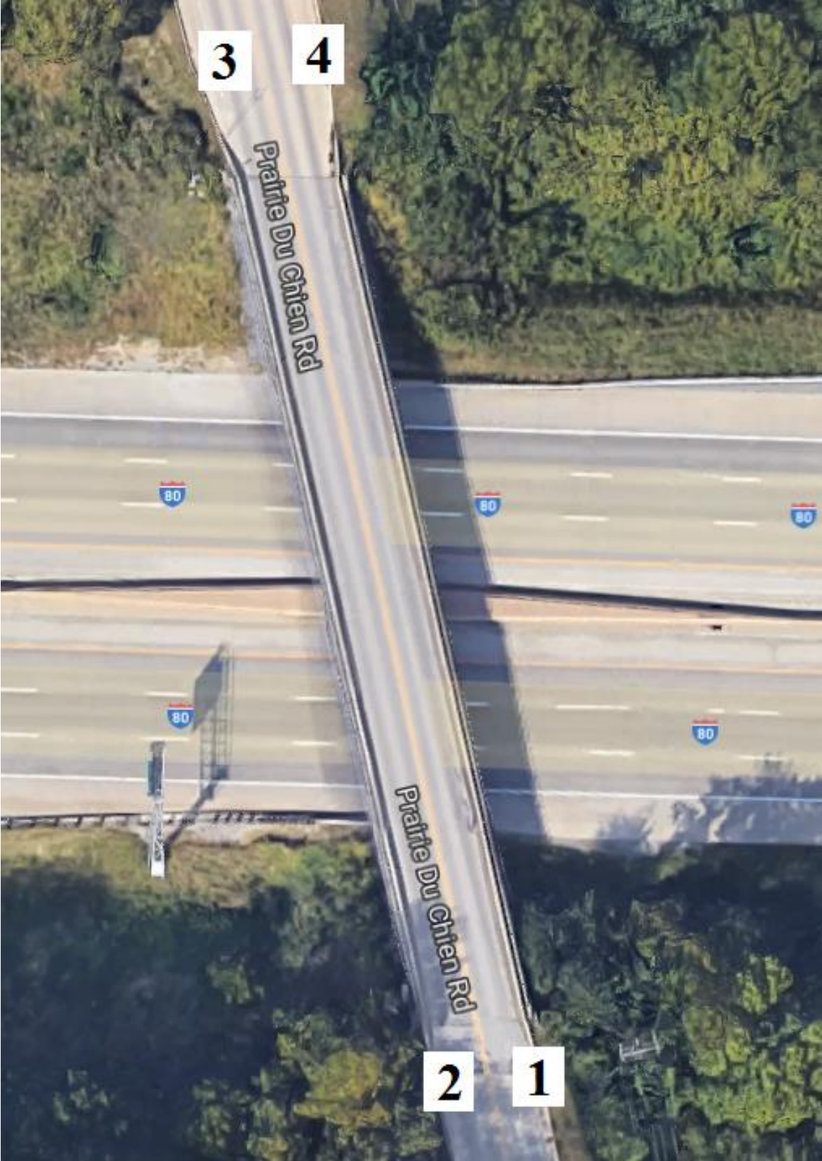
Figure B-79. Bridge No. 5245.1O080 [1]
