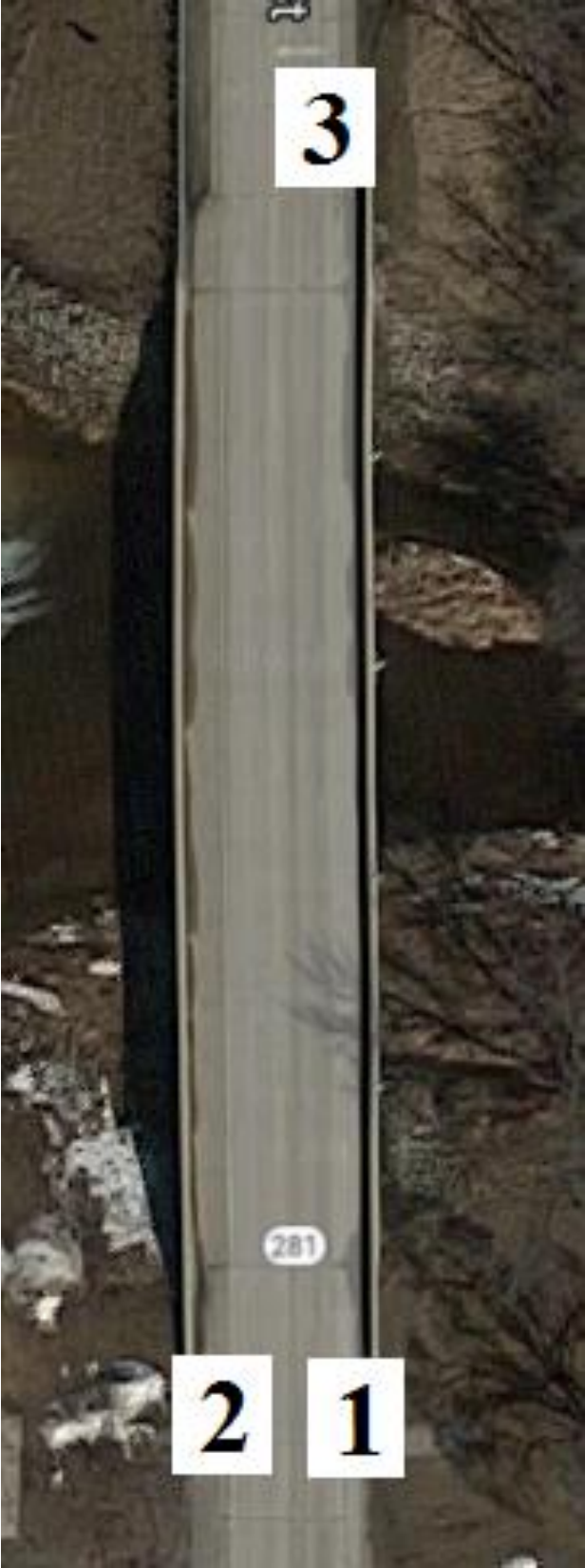
Figure B-5. Bridge No. 0713.9S281 [1]
