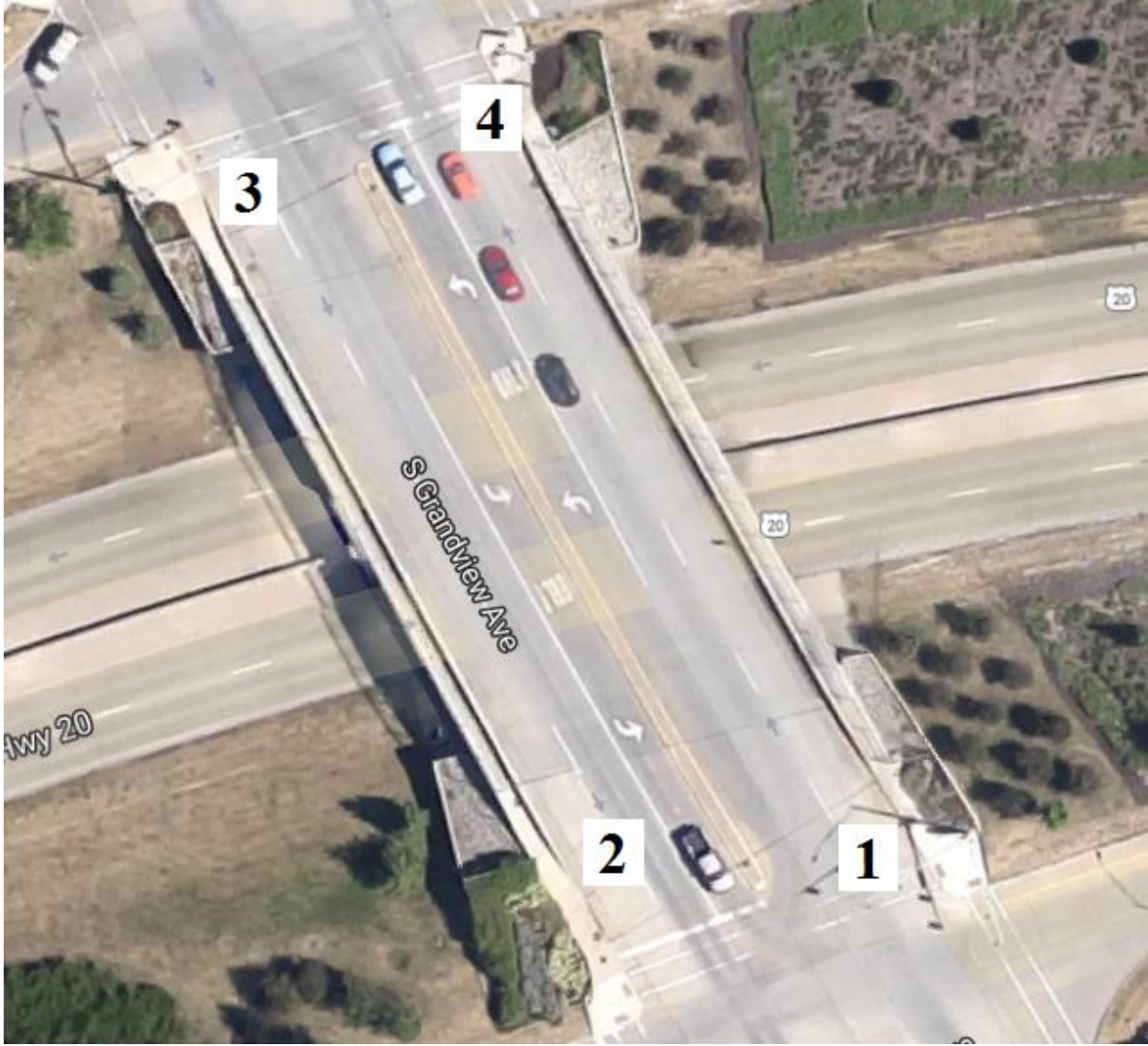
Figure B-50. Bridge No. 3118.50020 [1]
