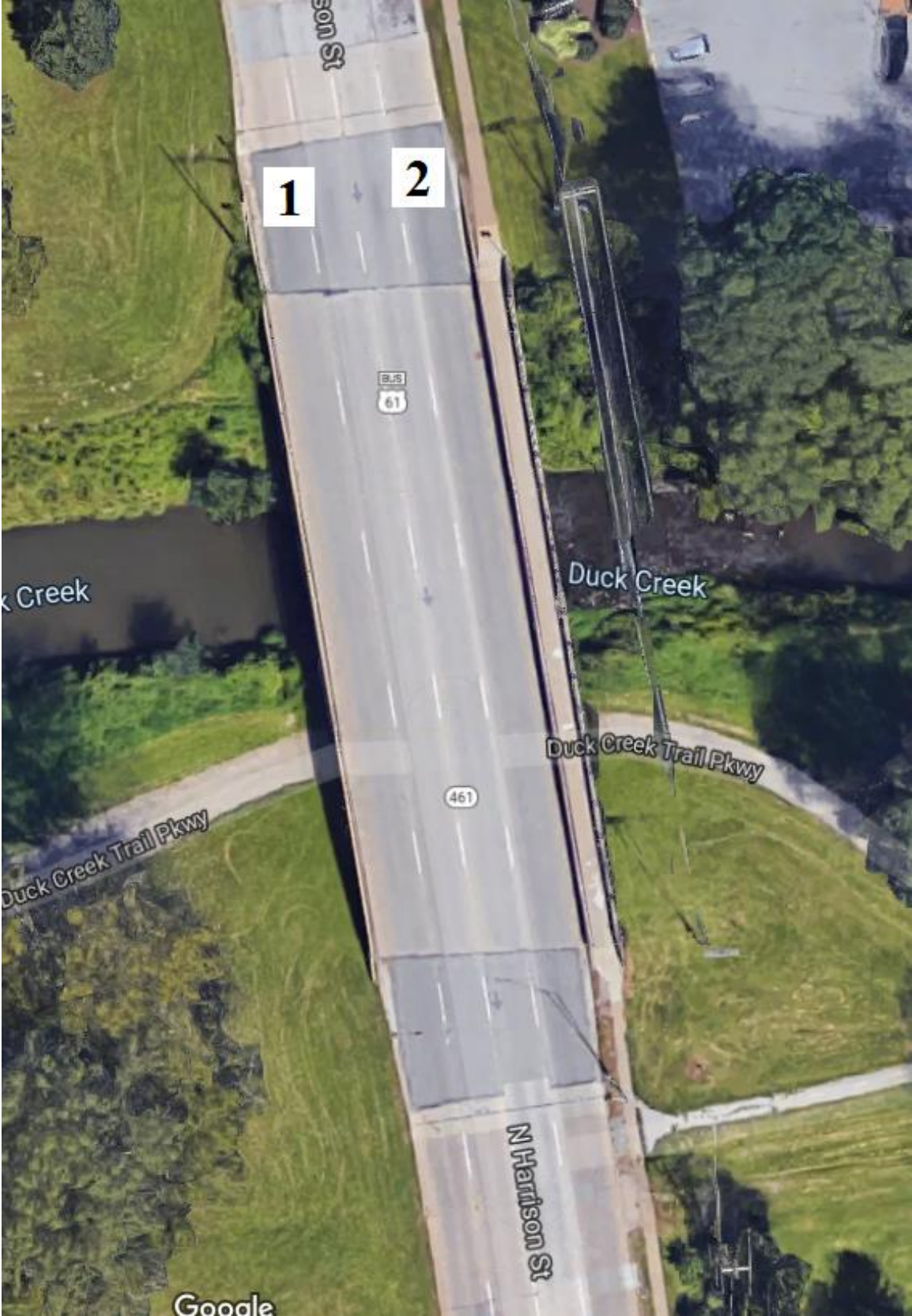
Figure B-155. Bridge No. 8220.1L061 [1]
