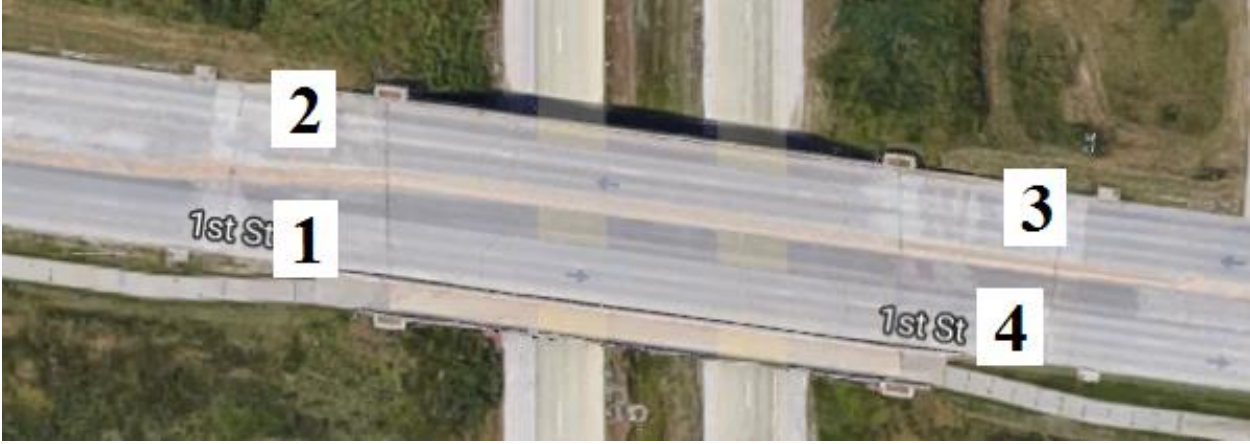
Figure B-183. Bridge No. 9741.2O029 [1]
