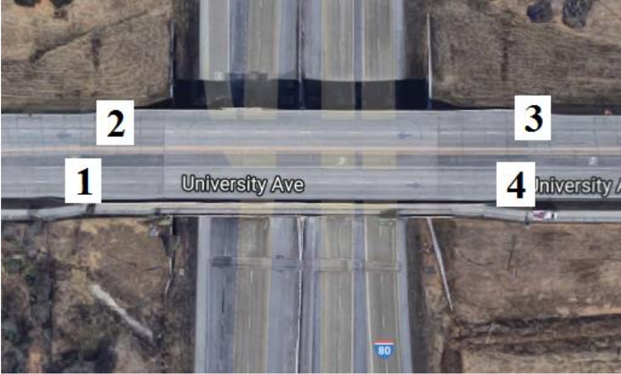
Figure B-140. Bridge No. 7724.1O080 [1]
