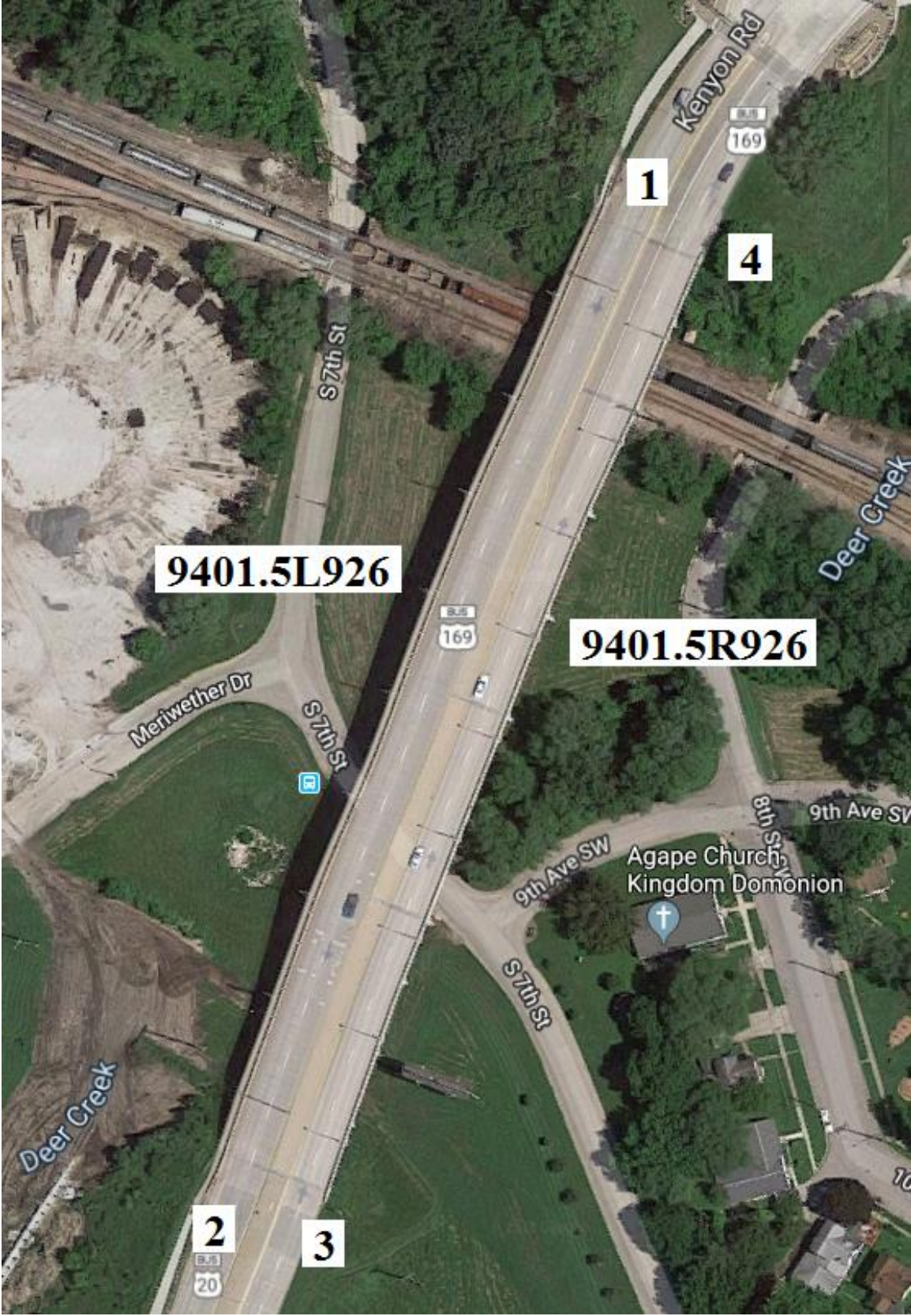
Figure B-174. Bridge Nos. 9401.5L926 and 9401.5R926 [1]
