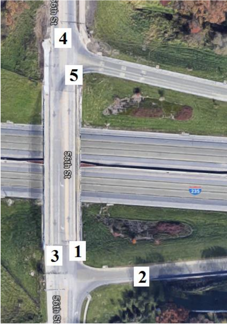
Figure B-119. Bridge No. 7704.4O235 [1]
