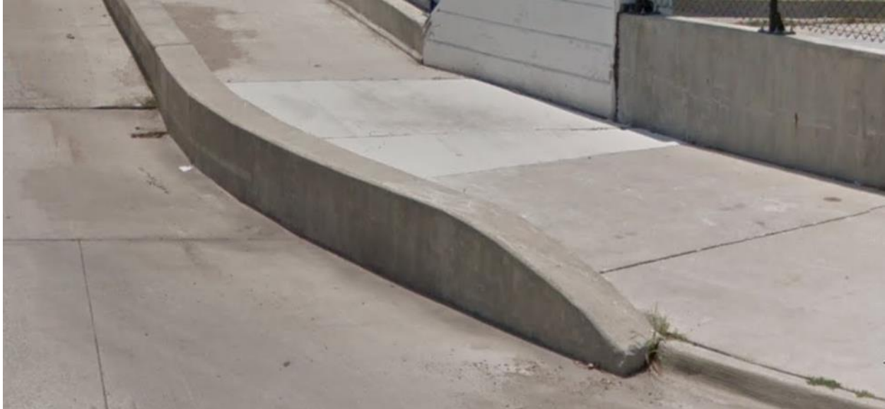
Figure 155. Special Case Sloped End Treatment [1]
