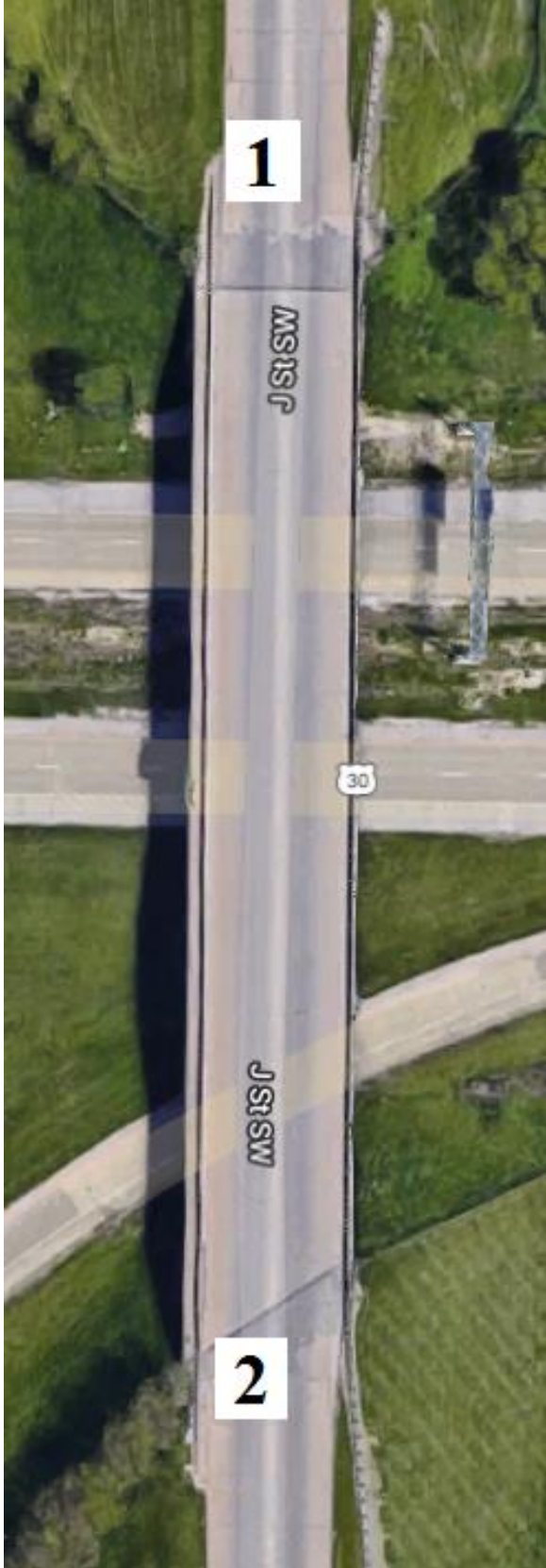
Figure B-99. Bridge No. 5752.9O030 [1]
