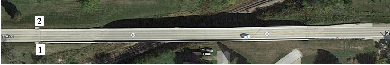
Figure B-65. Bridge No. 4208.0S057 [1]
