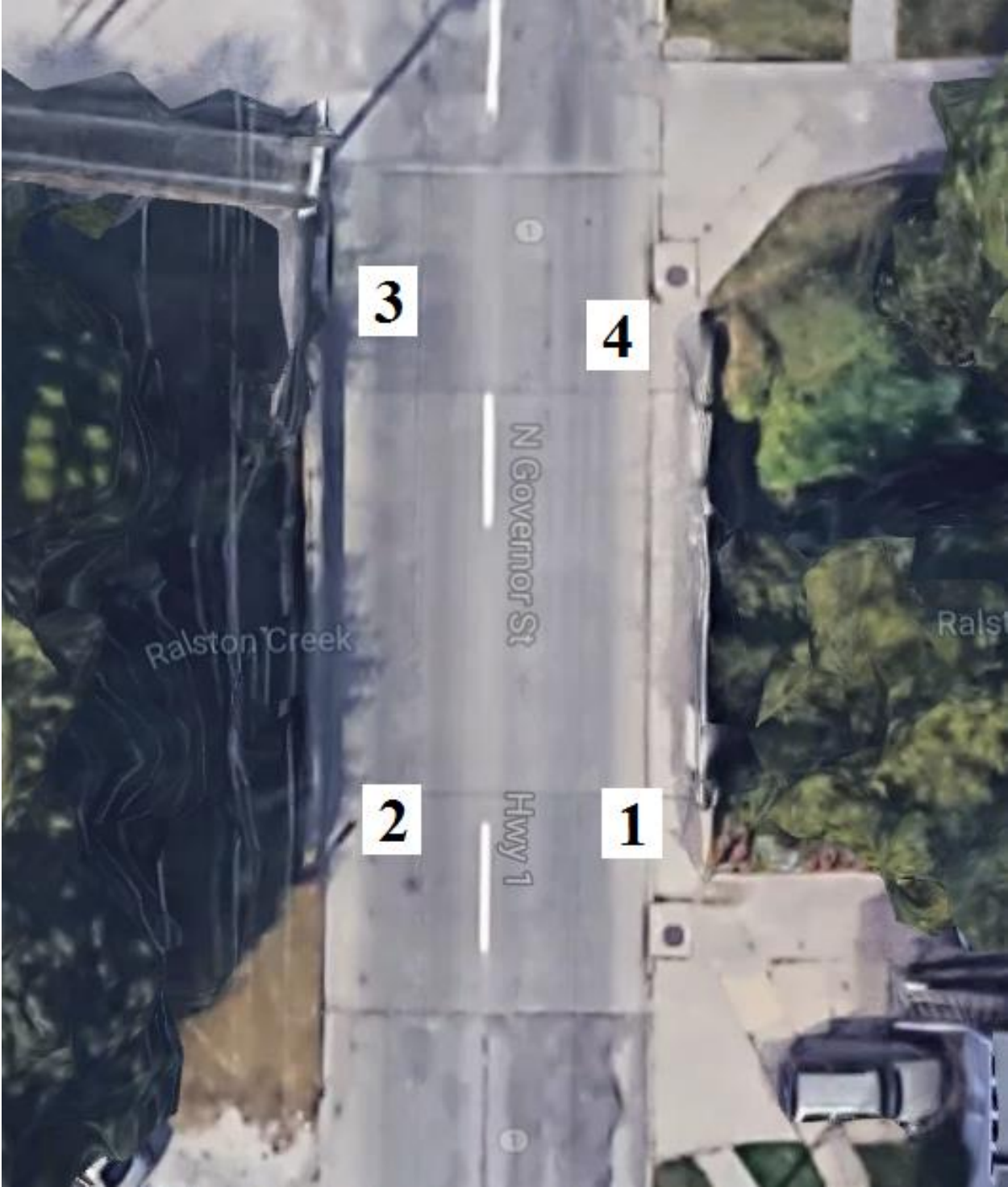
Figure B-84. Bridge No. 5287.2R001 [1]
