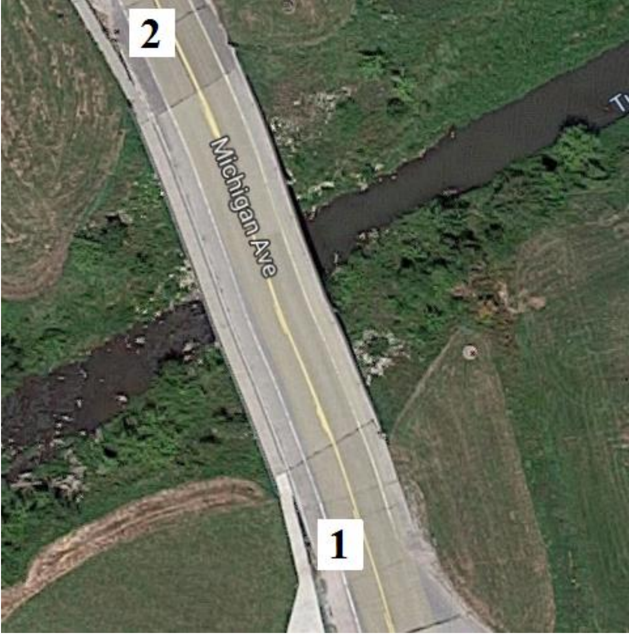
Figure B-21. Bridge No. 1562.9S148 [1]
