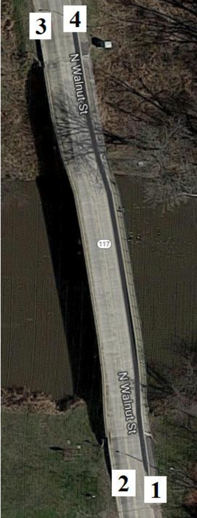
Figure B-75. Bridge No. 5007.7S117 [1]
