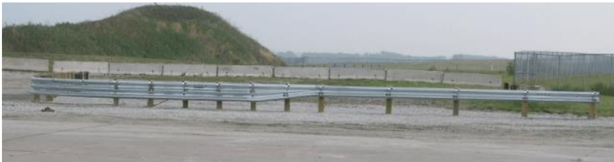
Figure 5. Short Radius Guardrail [26]
