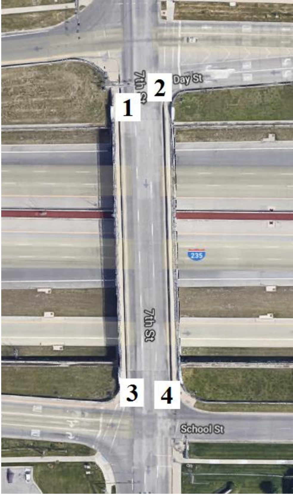
Figure B-126. Bridge No. 7707.9O235 [1]
