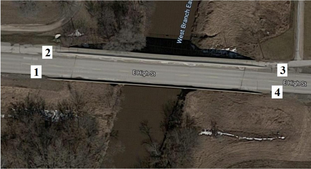
Figure B-149. Bridge No. 7815.0S083 [1]
