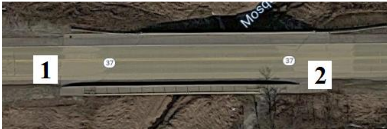
Figure 70. Bridge No. 8336.8S037 [1]
