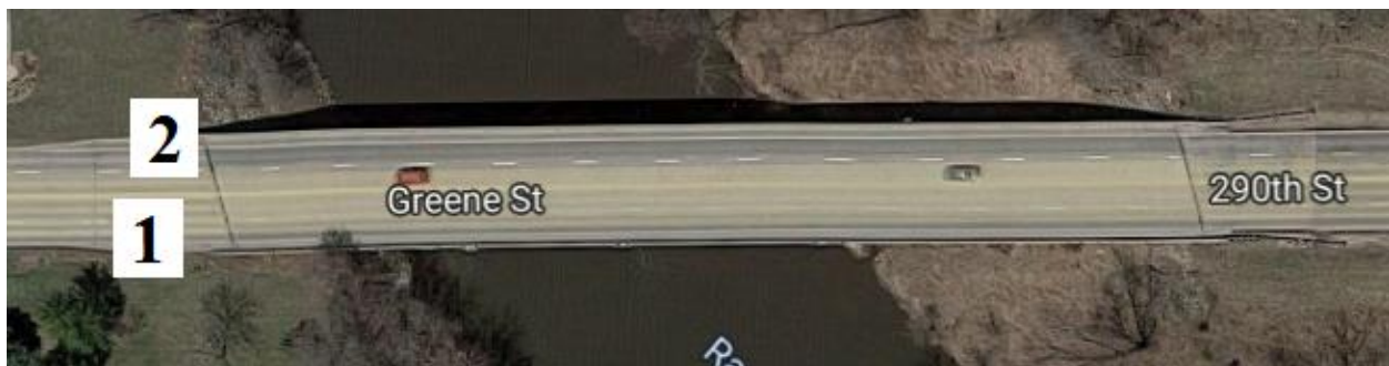
Figure 69. Bridge No. 2515.1S006 [1]
