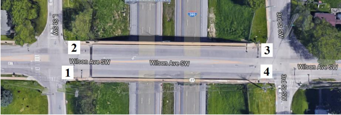
Figure B-91. Bridge No. 5718.40380 [1]
