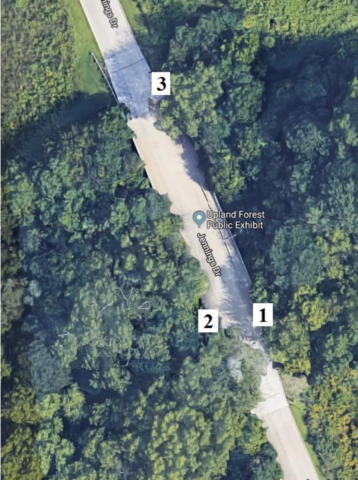
Figure B-4. Bridge No. 0700.4S820 [1]
