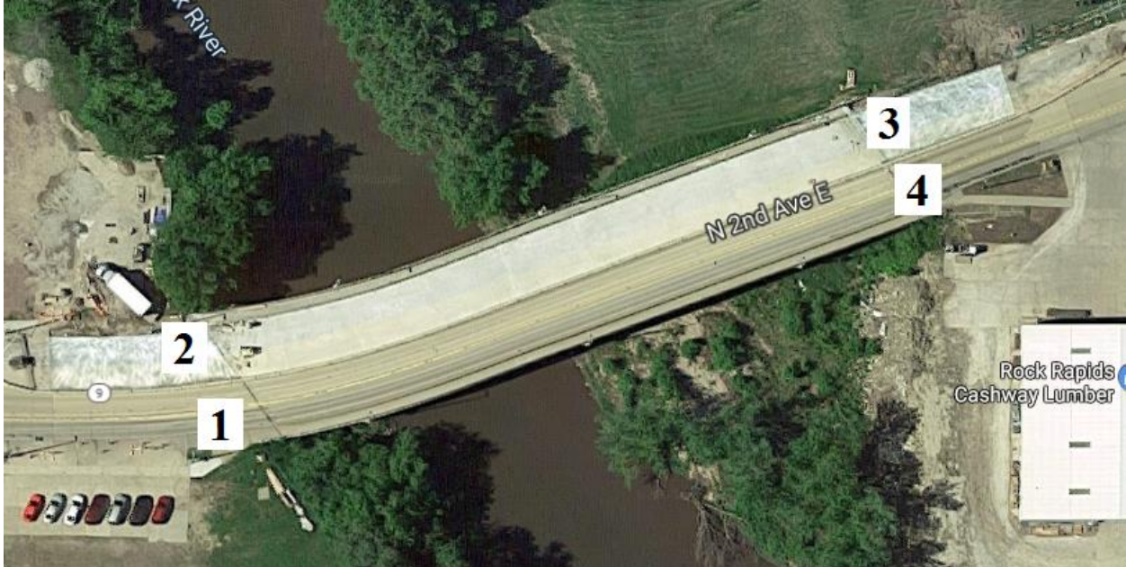
Figure B-102. Bridge No. 6020.4S009 [1]
