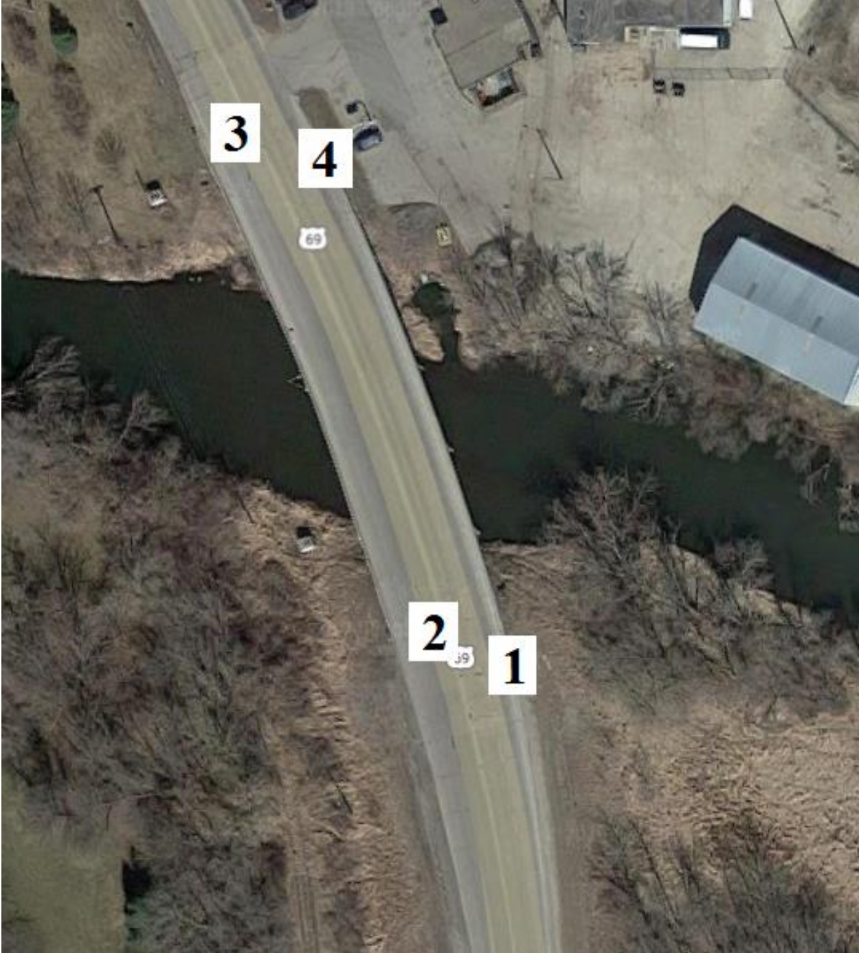
Figure B-175. Bridge No. 9505.0S069 [1]
