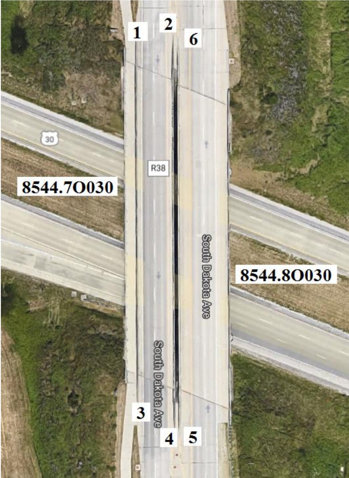
Figure B-161. Bridge Nos. 8544.70030 and 8544.80030 [1]
