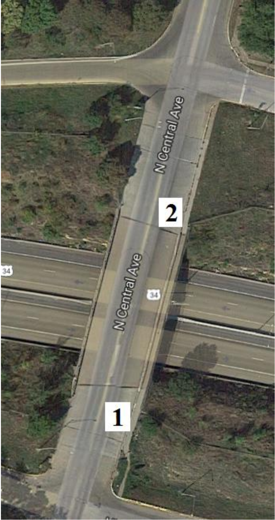
Figure B-42. Bridge No. 2962.9O034 [1]
