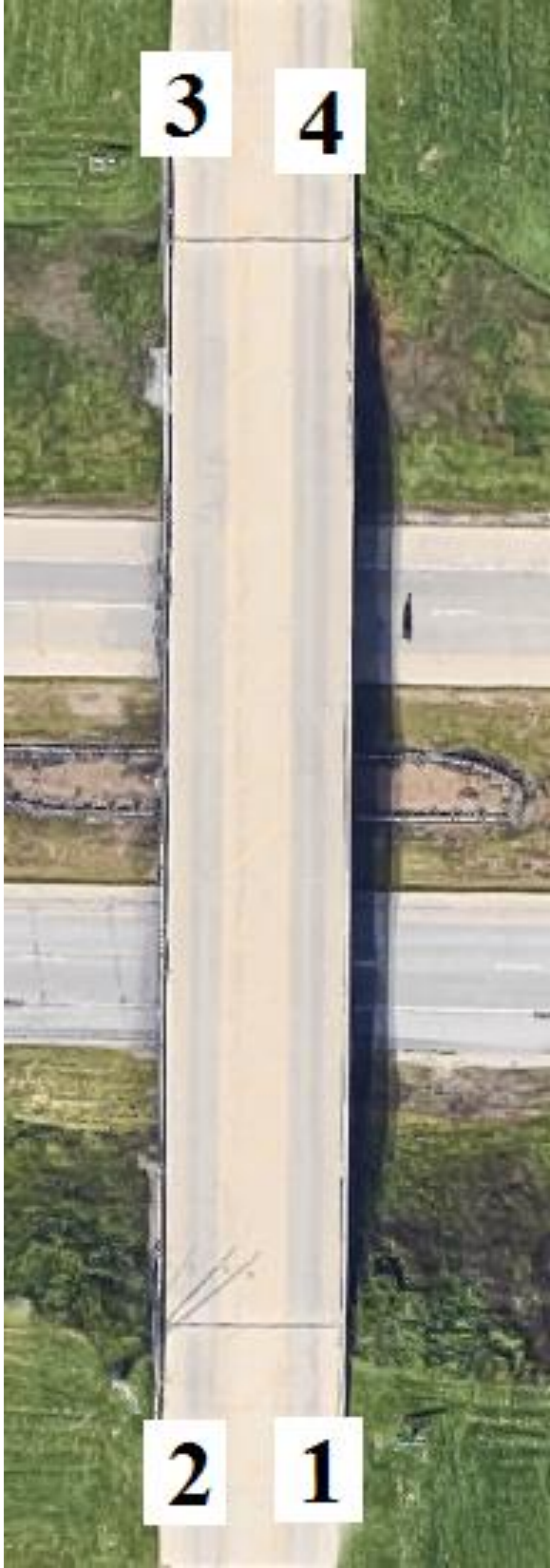
Figure B-7. Bridge No. 0729.00020 [1]
