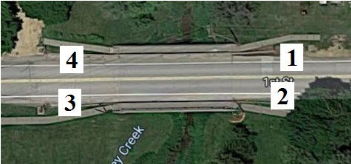
Figure B-30. Bridge No. 2318.8S136 [1]
