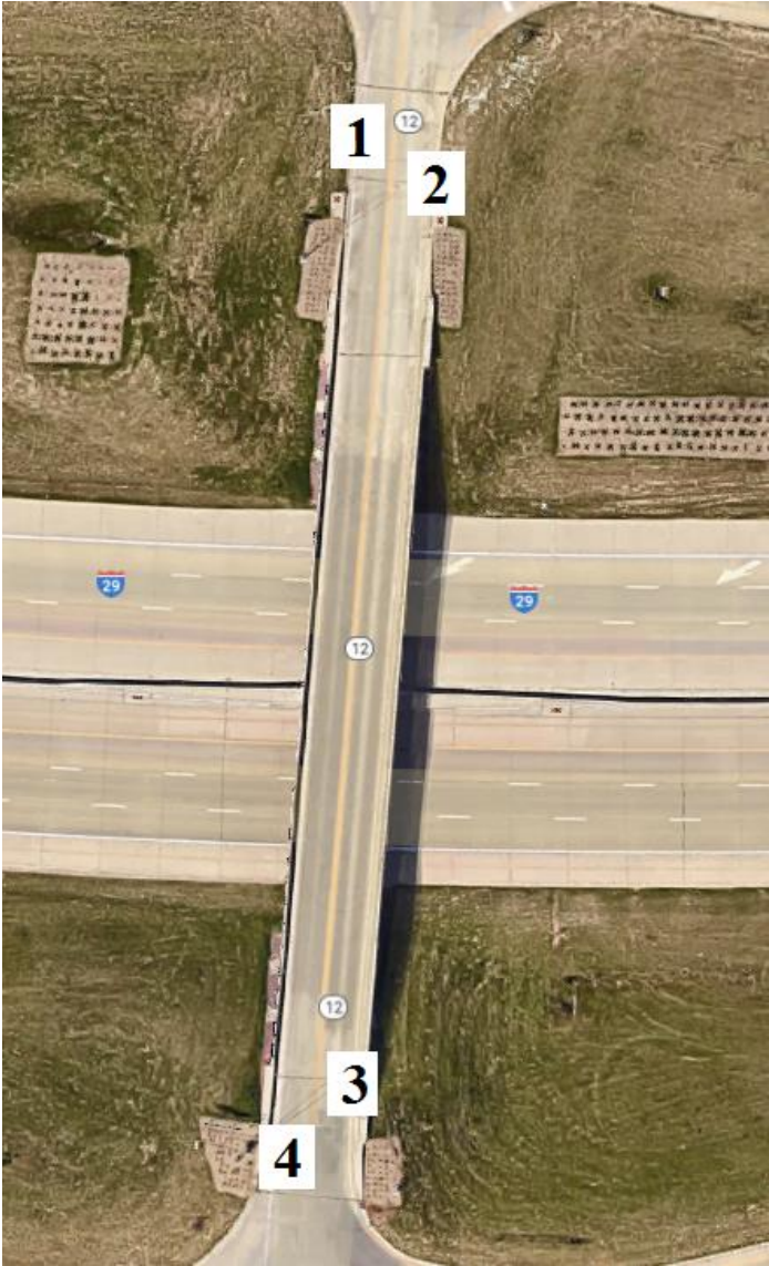
Figure B-182. Bridge No. 9708.1S012 [1]
