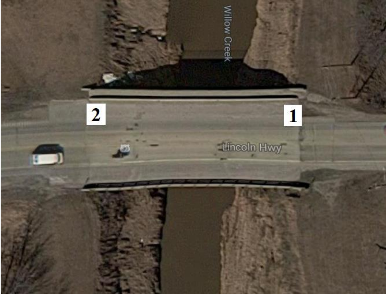
Figure B-66. Bridge No. 4309.8S030 [1]
