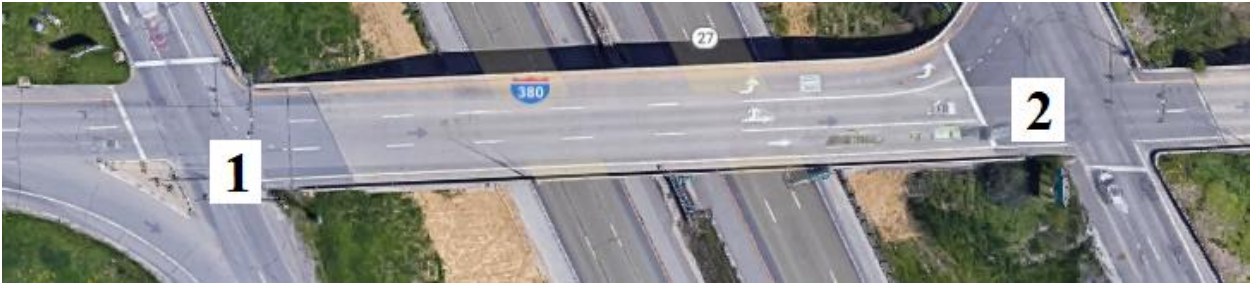
Figure B-95. Bridge No. 5723.80380 [1]
