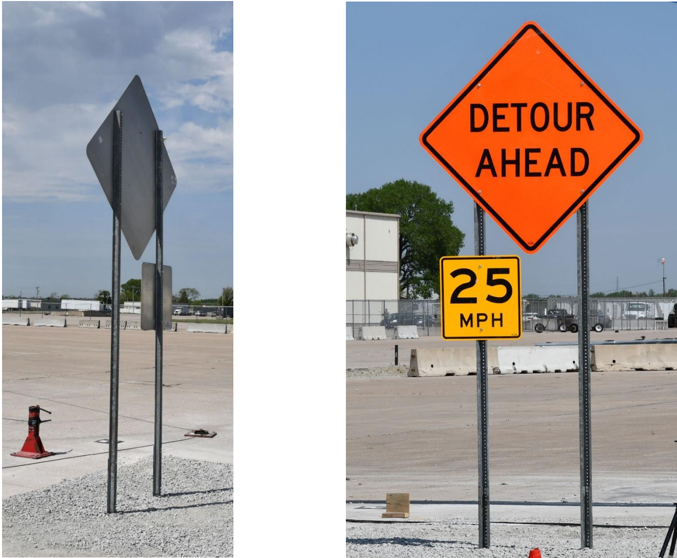
Figure 12. Test Installation Photographs, Test Nos. MOS-5 through MOS-7
