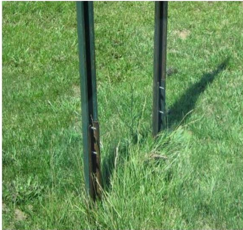
Figure 1. Ground-Mounted, Dual-Post, U-channel Sign System
