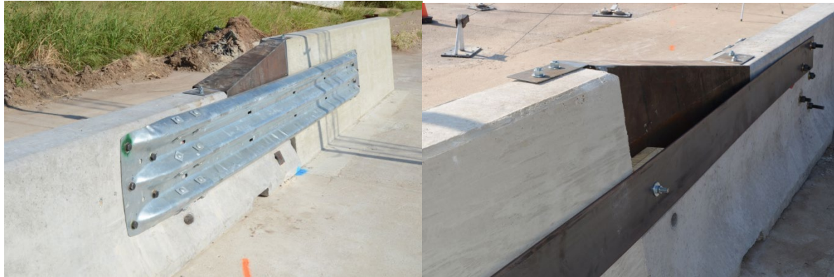
Figure 1 – Photos of the Height Transition for MASH Test Level 3 (Test 3-21)
