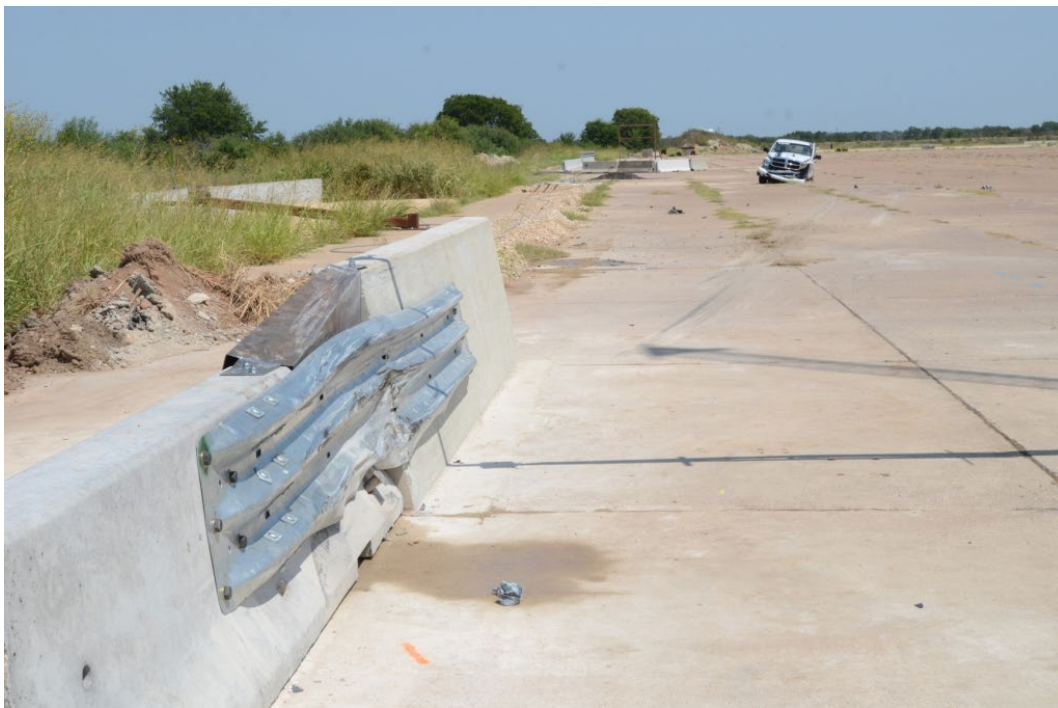
Figure 2 – Photos of the Height Transition After MASH Test 3-21
