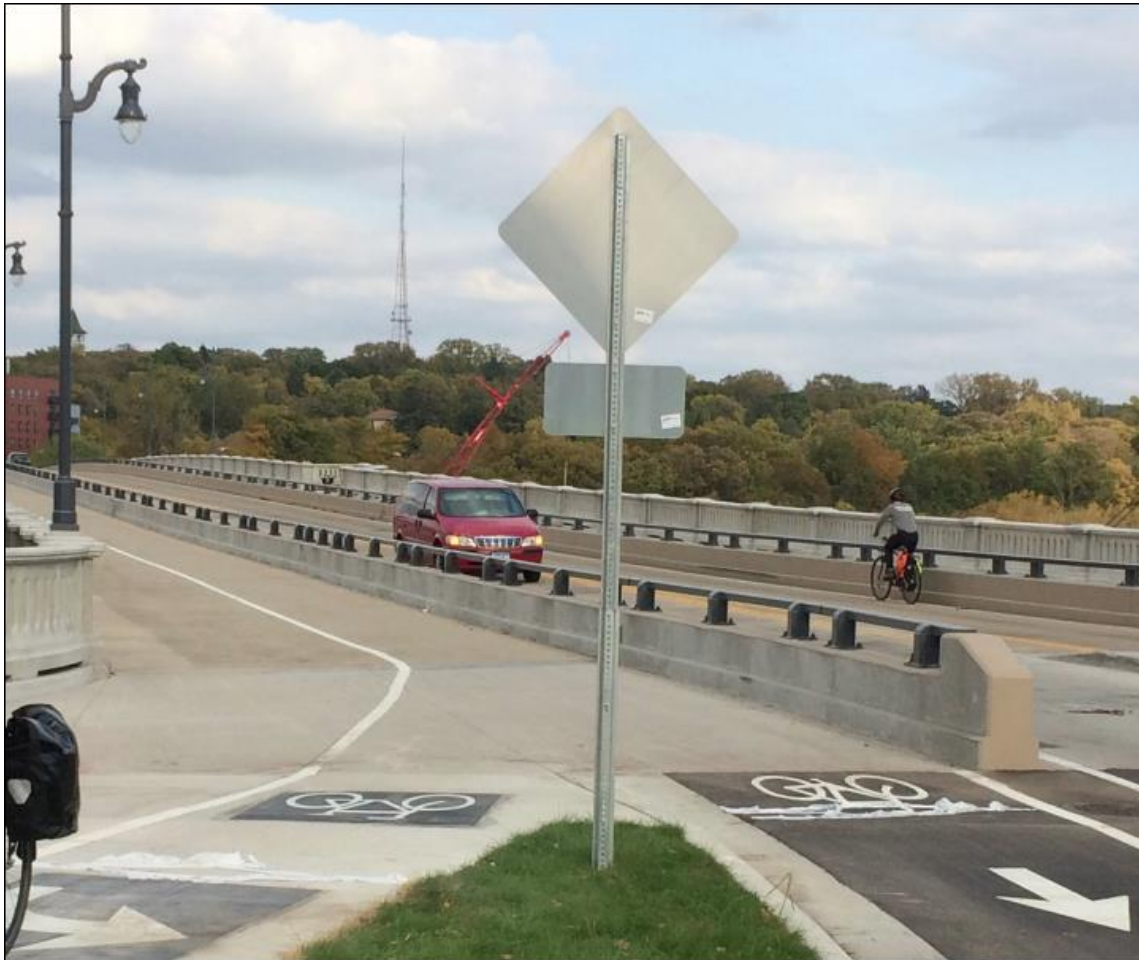
Figure 1. Typical Concrete Parapet with Brush Curb and Upper Beam and Post Rail
