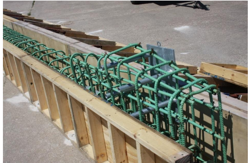
Figure 37. New Concrete Tapered End Rebar Installation, Test Nos. MNCBR-1, MNCBR-2, and MNCBR-3
