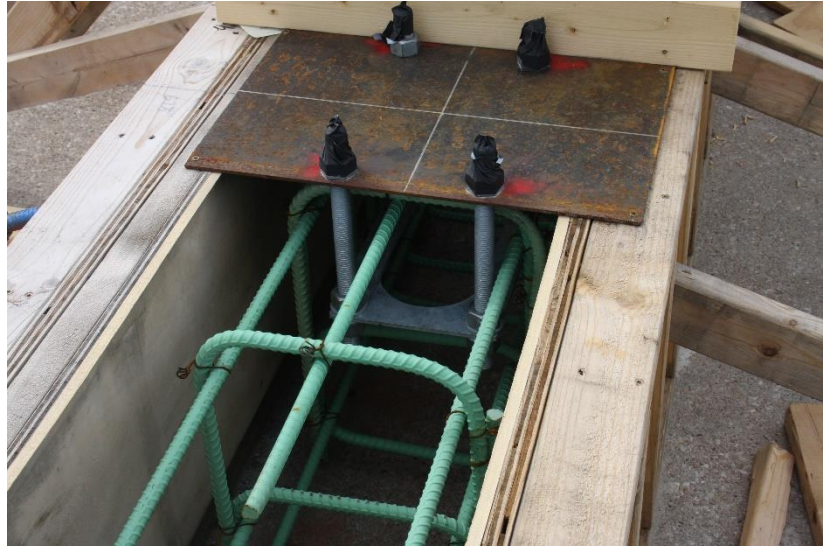
Figure 38. New Concrete Tapered End Rebar Installation, Test Nos. MNCBR-1, MNCBR-2, and MNCBR-3
