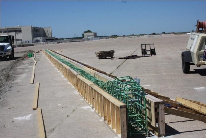
Figure 37. New Concrete Tapered End Rebar Installation, Test Nos. MNCBR-1, MNCBR-2, and MNCBR-3
