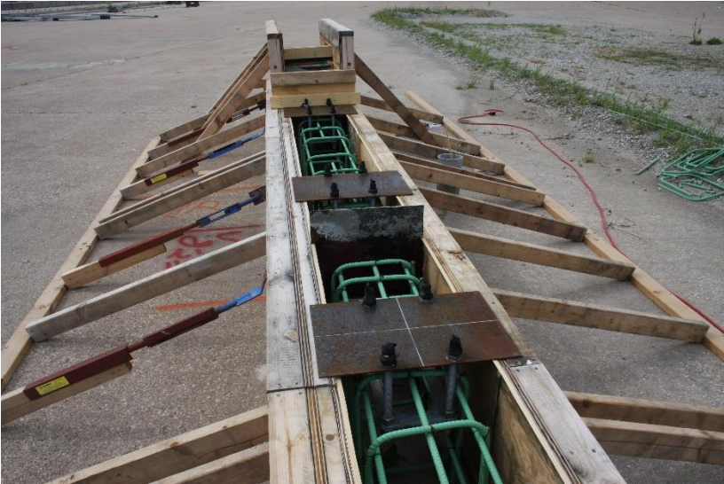
Figure 38. New Concrete Tapered End Rebar Installation, Test Nos. MNCBR-1, MNCBR-2, and MNCBR-3
