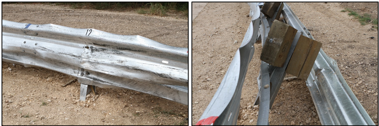
Figure 6.5. Post 12 after Test No. 611971-03-2.
