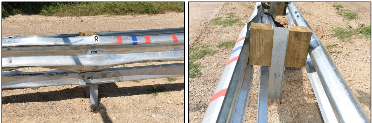
Figure 5.4. Post 8 after Test No. 611971-03-1.
