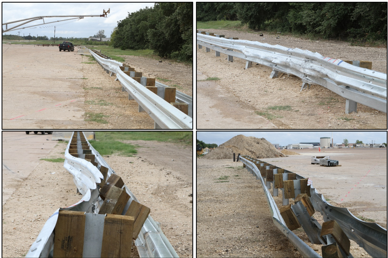
Figure 6.3. Median Barrier after Test No. 611971-03-2.
