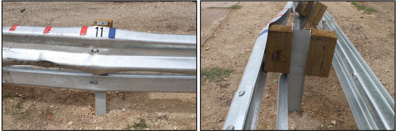
Figure 6.4. Post 11 after Test No. 611971-03-2.
