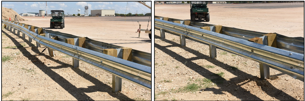
Figure 5.7. Field Side of Median Barrier after Test No. 611971-03-1.
