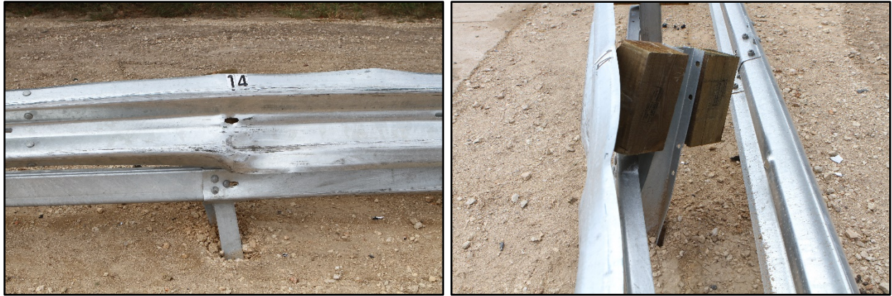
Figure 6.7. Median Barrier after Test No. 611971-03-2.
