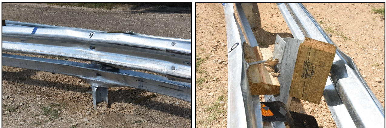
Figure 5.5. Post 9 after Test No. 611971-03-1.
