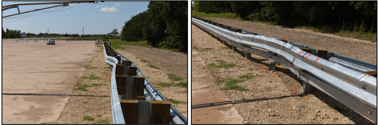
Figure 5.3. Median Barrier after Test No. 611971-03-1.
