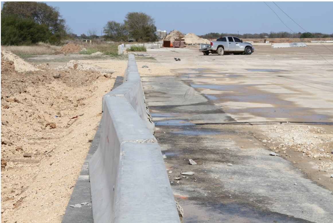
Figure 17. Pinned barrier installed on asphalt after MASH test 3-11.
