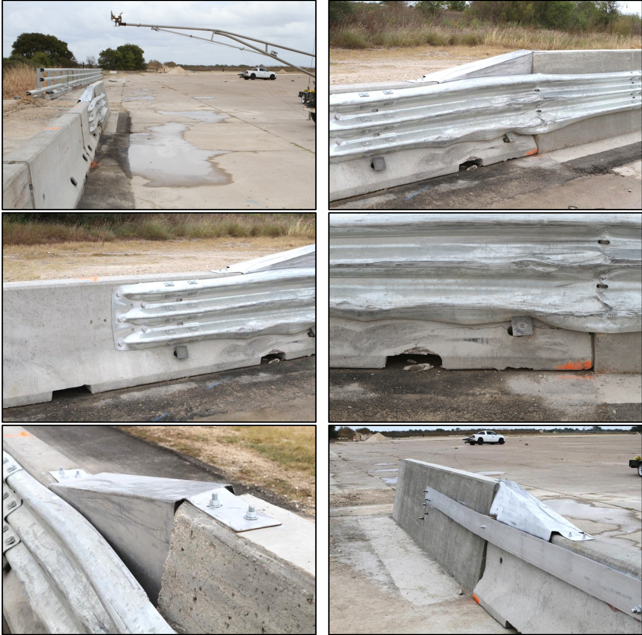
Figure 28. Test installation after full-scale crash testing.
