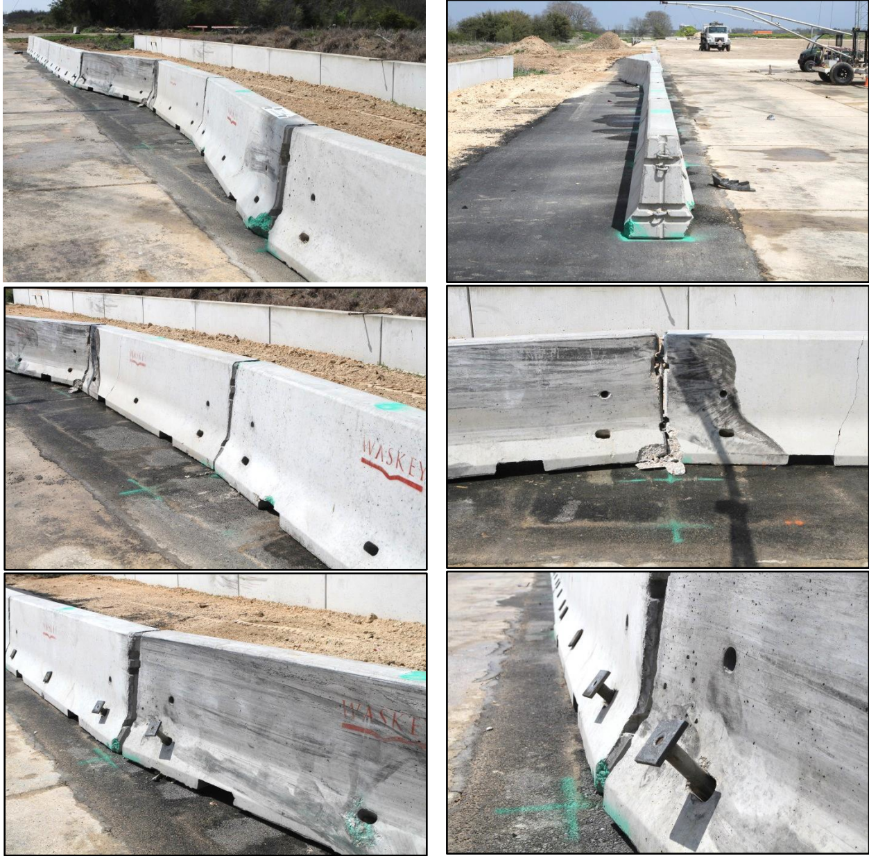
Figure 23. Test installation after full-scale crash testing.
