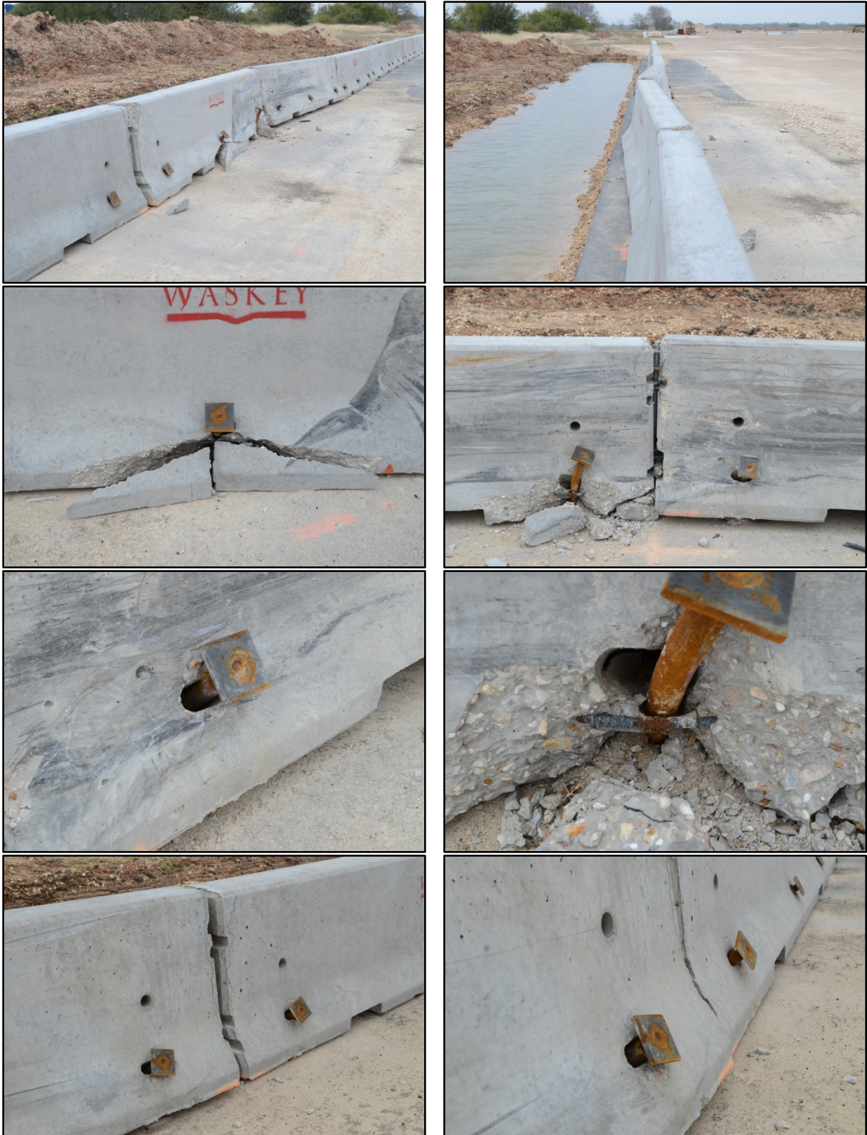
Figure 18. Barrier deflection and damage after full-scale crash testing.
