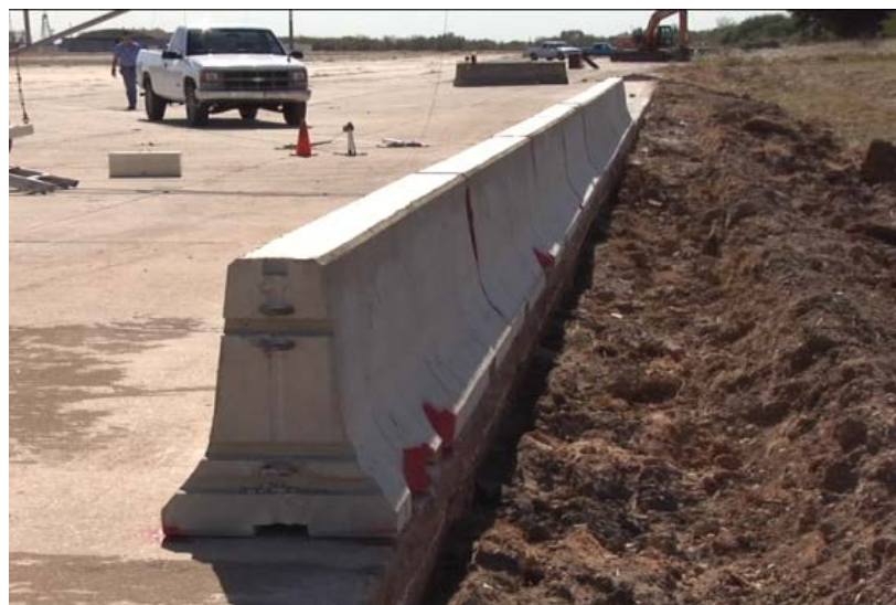
Figure 11. Test installation of the pinned-down barrier on concrete.
