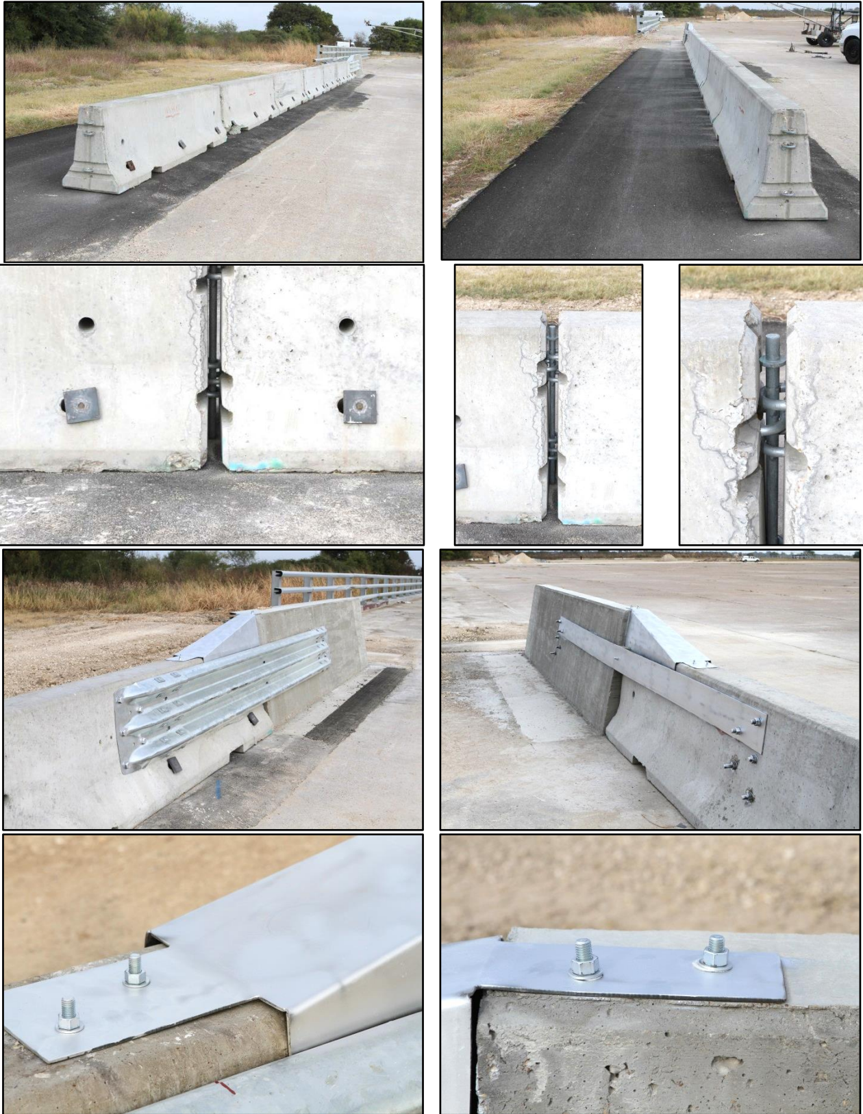
Figure 27. Installation of transition from pinned-down to permanent single slope concrete barrier.
