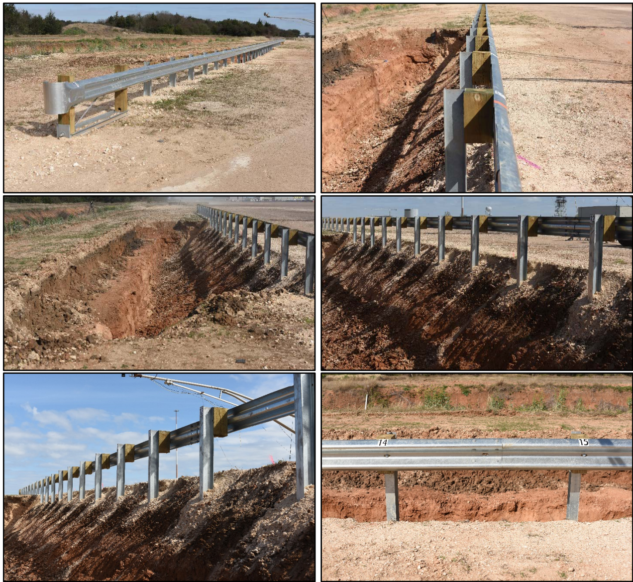
Figure 2.1. Guardrail on 1H:1V Slope prior to Test No. 609301-01-1.
