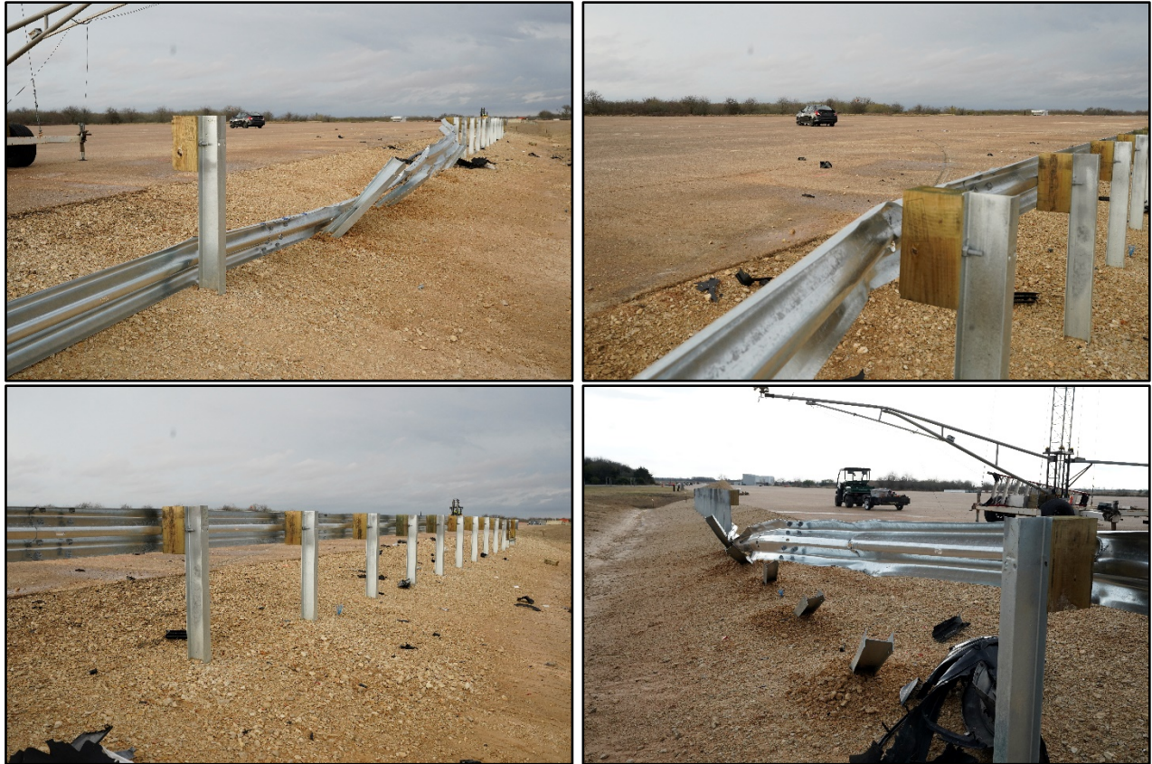
Figure 7.5. Field Side after Test No. 613011-01-1.
