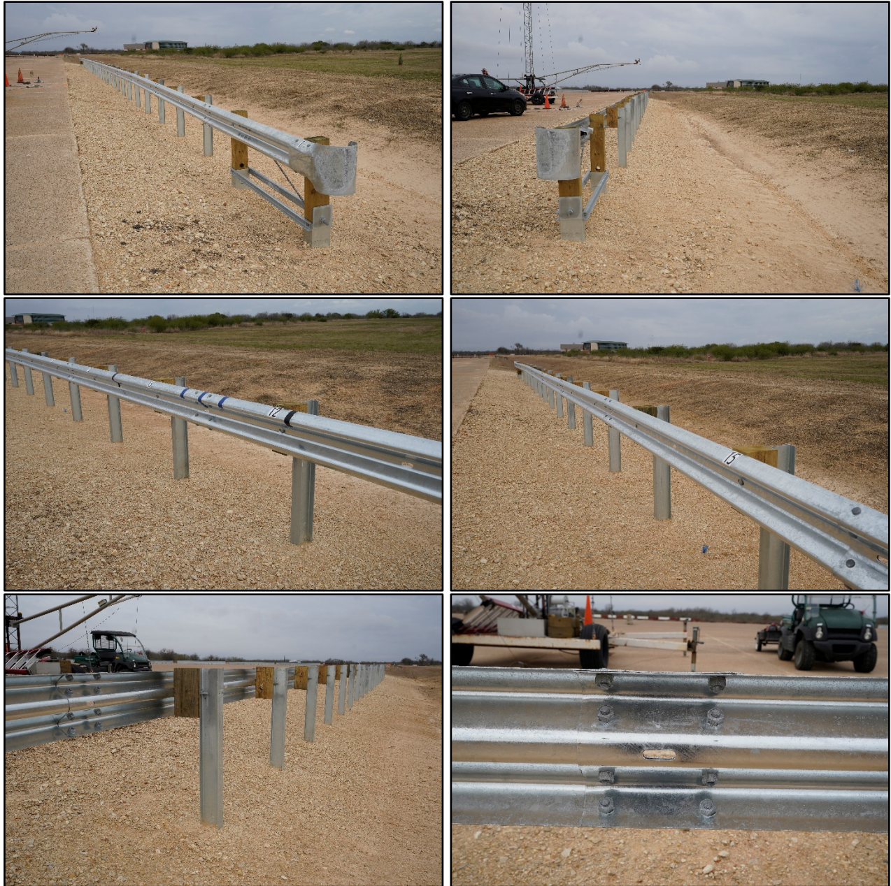
Figure 4.2. Guardrail on 6H:1V Slope prior to Testing.
