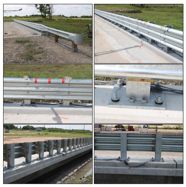
Figure 2.2. Thrie Beam Bridge Rail Retrofit prior to Testing.
