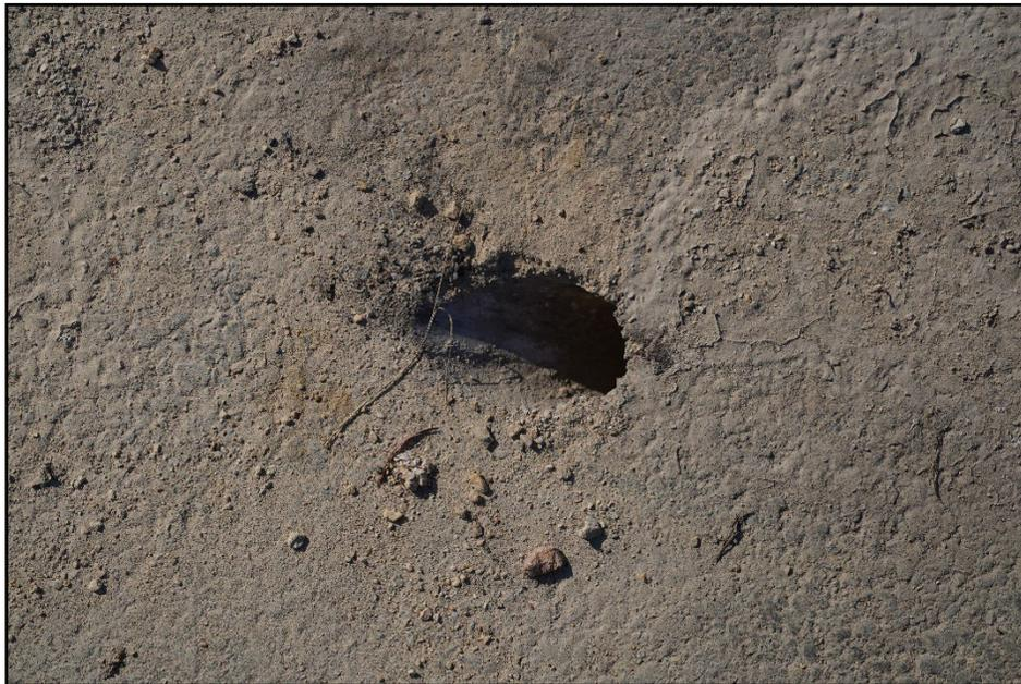
**Figure 7.12. Asphalt Damage at the Downstream Anchor Pin Location 616391-01-2.**
