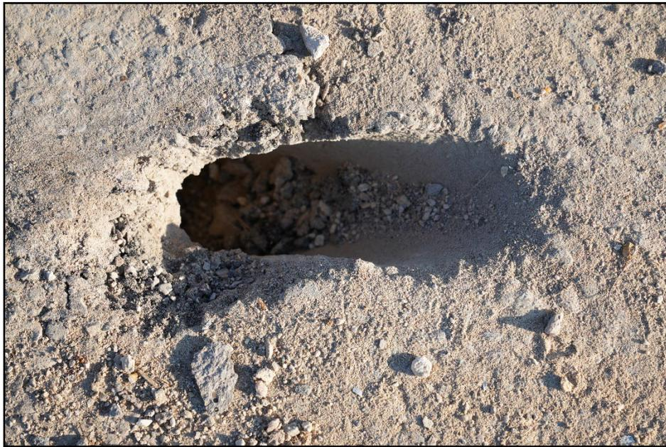
**Figure 6.8. Asphalt Damage at the Upstream Anchor Pin Location 616391-01-1.**
