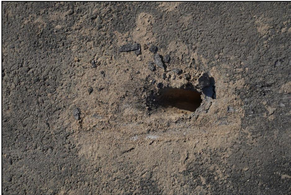
**Figure 7.10. Asphalt Damage at the Middle Anchor Pin Location 616391-01-2.**
