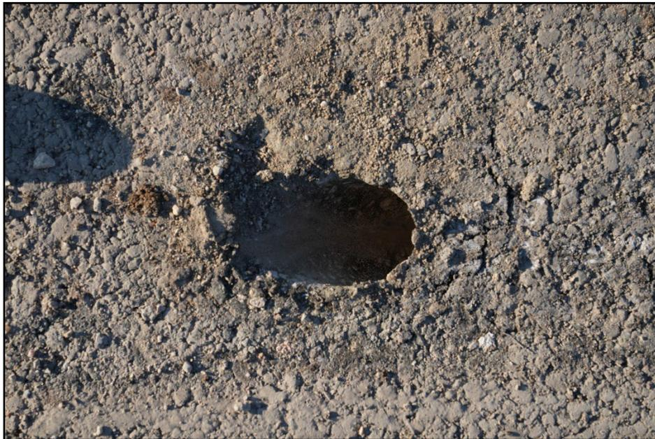
**Figure 6.10. Asphalt Damage at the Middle Anchor Pin Location 616391-01-1.**
