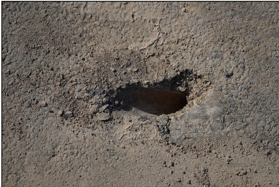
**Figure 7.8. Asphalt Damage at the Upstream Anchor Pin Location 616391-01-2.**
