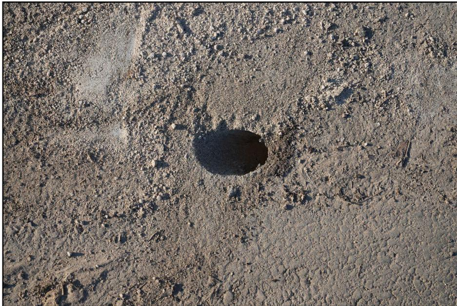
**Figure 6.12. Asphalt Damage at the Downstream Anchor Pin Location 616391-01-1.**
