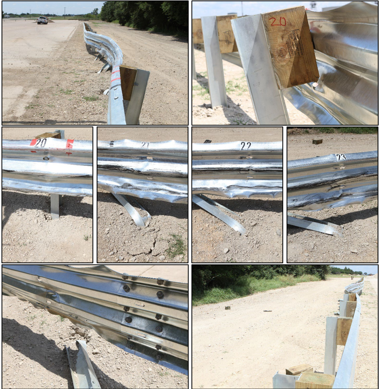
Figure 6.5. Roadside Thrie-beam System after Test No. 614341-01-1.
