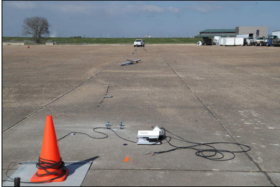
Figure 6.5. Crashworthy Enhanced Highway Sign Assemblies after Test at Impact Location 616161-01-2.
