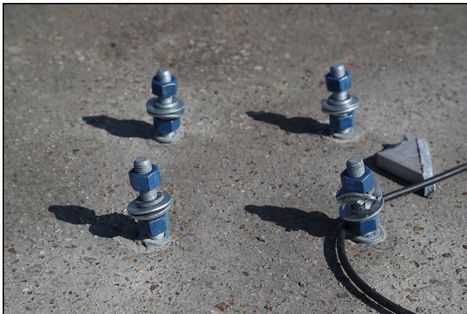
Figure 6.6. Crashworthy Enhanced Highway Sign Assemblies after Test at the Anchor Bolts 616161-01-2.
