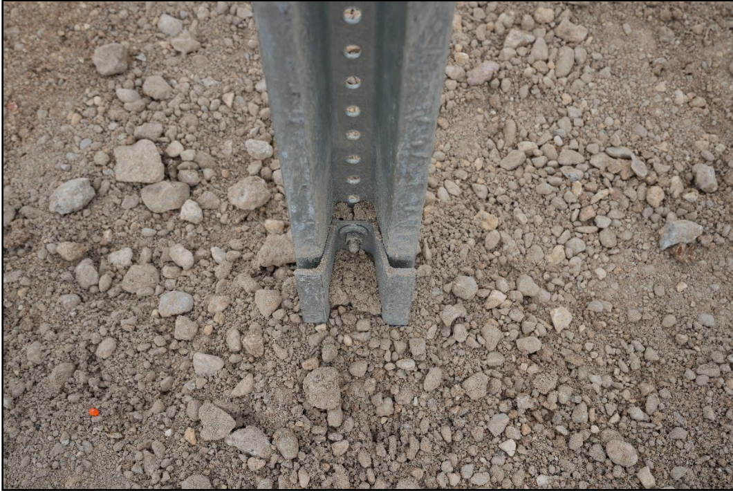
Figure 2.6. Lower Section of the U-Channel Sign Support System prior to Testing.
