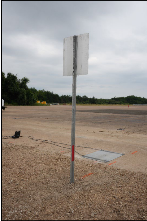
Figure 2.4. Rear of the U-Channel Sign Support System prior to Testing.
