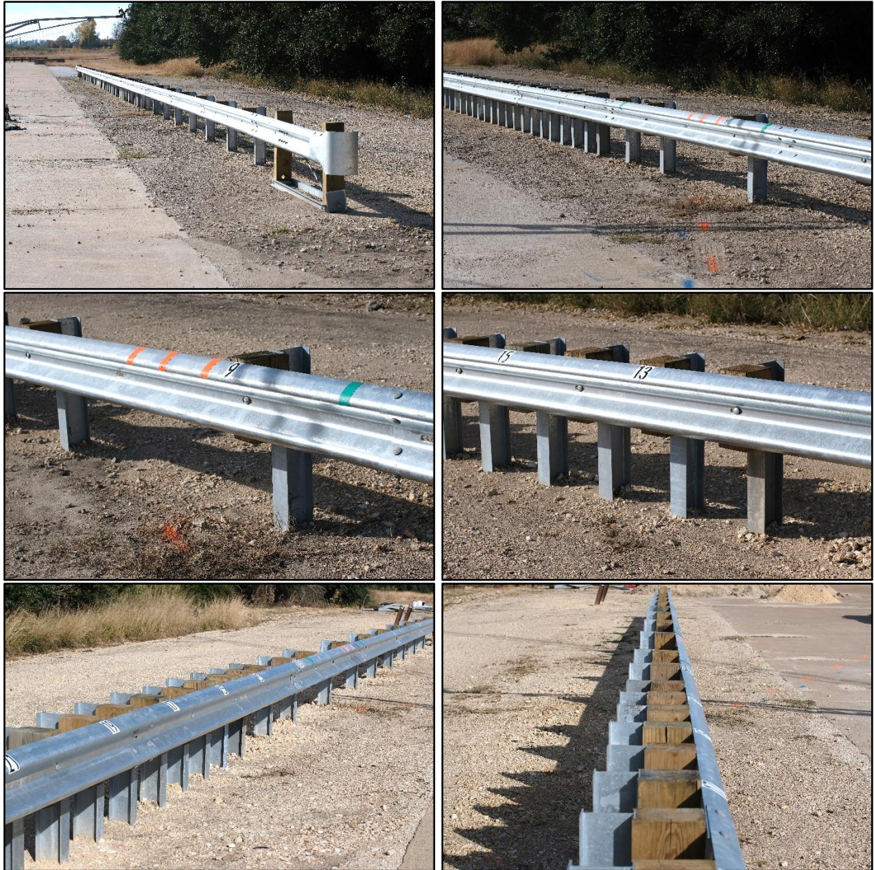
Figure 6.2. Transition from Full to Quarter Post Spacing prior to Testing.
