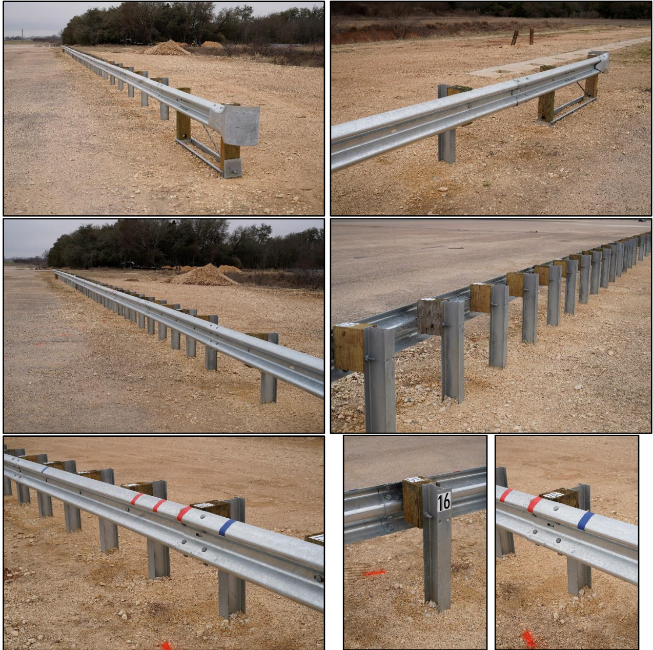
Figure 5.18. MGS with Half Post Spacing and Shortened Blockouts prior to Testing.
