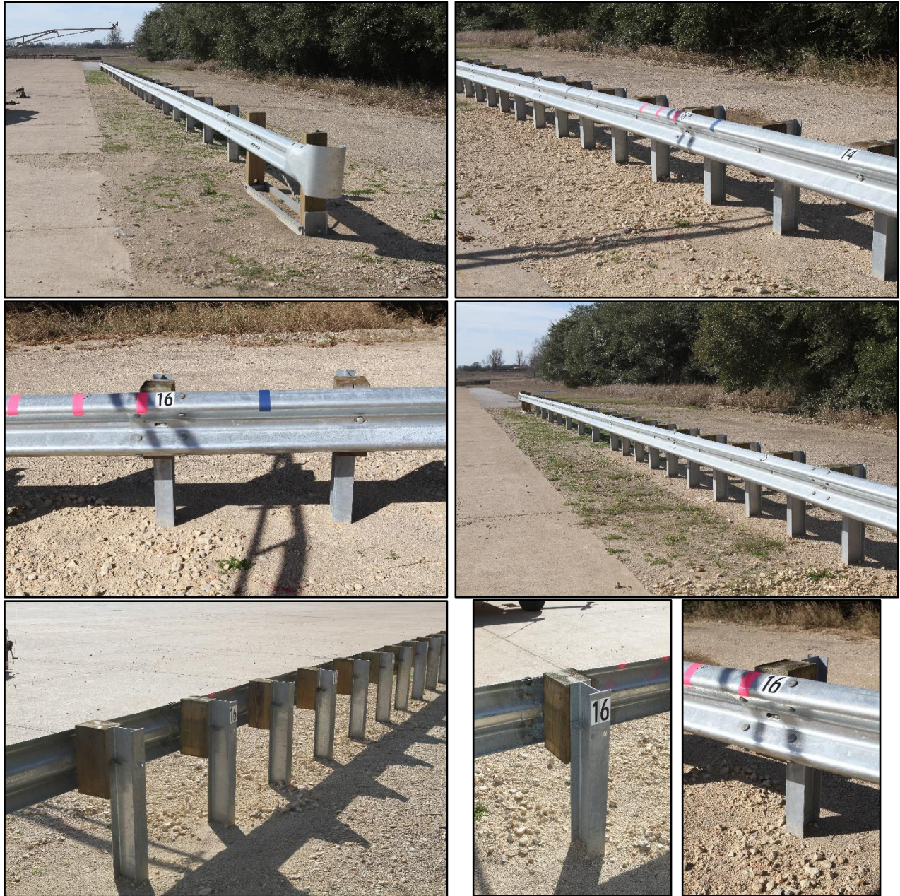
Figure 5.2. MGS with Half Post Spacing prior to Testing.
