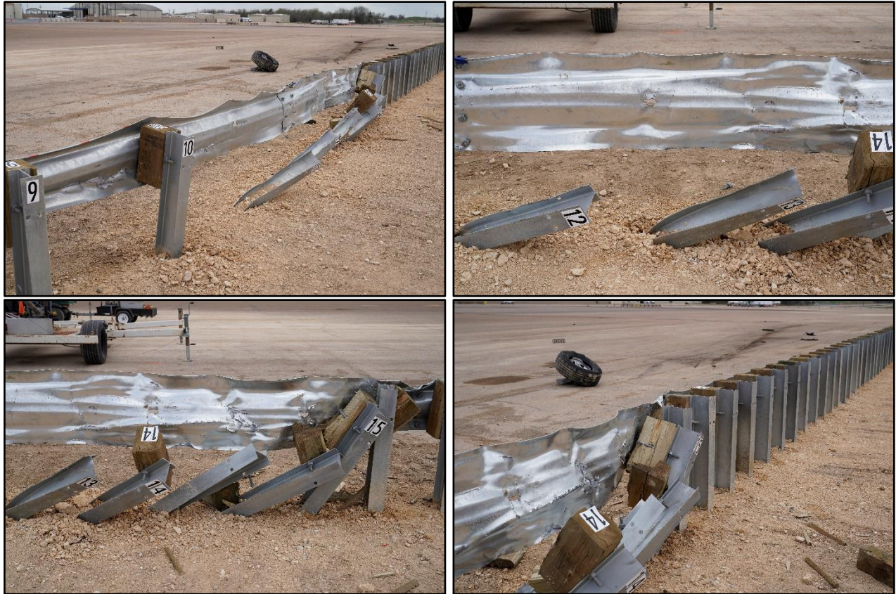
Figure 6.21. Field Side of Longer Transition from Full to Quarter Post Spacing after Test No. 610211-01-5.
