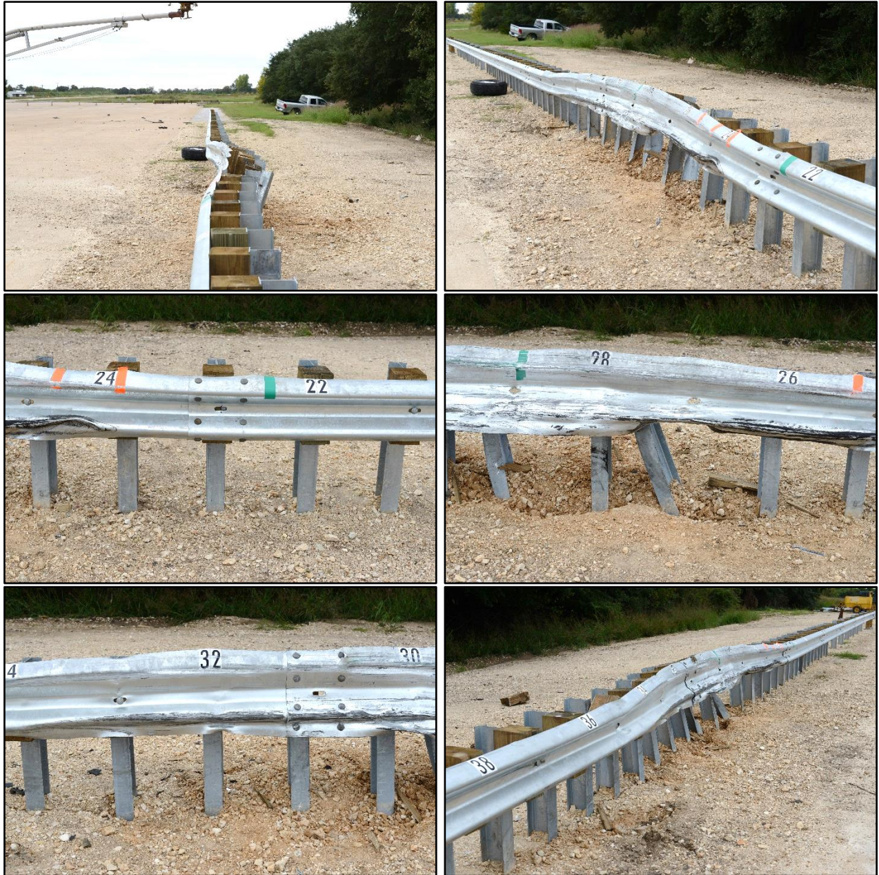
Figure 4.11. MGS System with Quarter Post Spacing after Test No. 610211-01-2.
