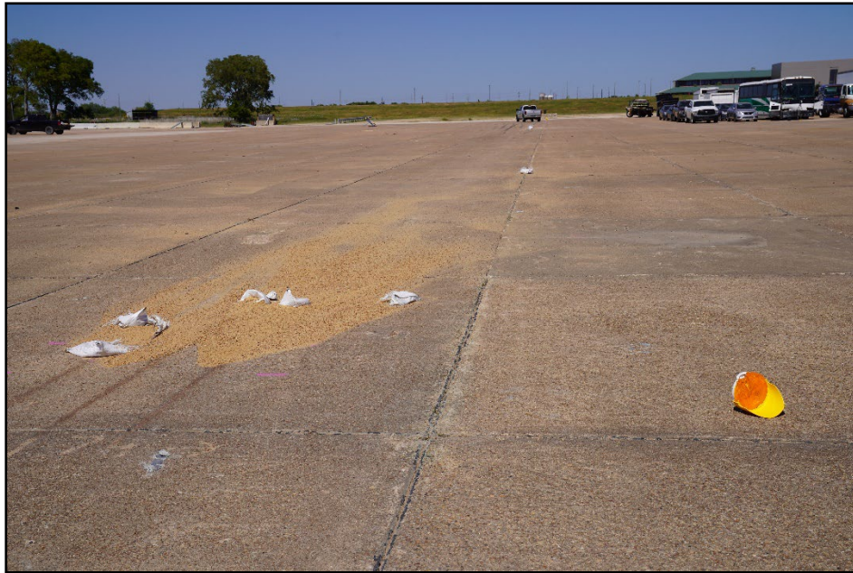
Figure 9.5. Type III Barricade with Mounted Sign after Test at Impact Location 616411-01-3.
