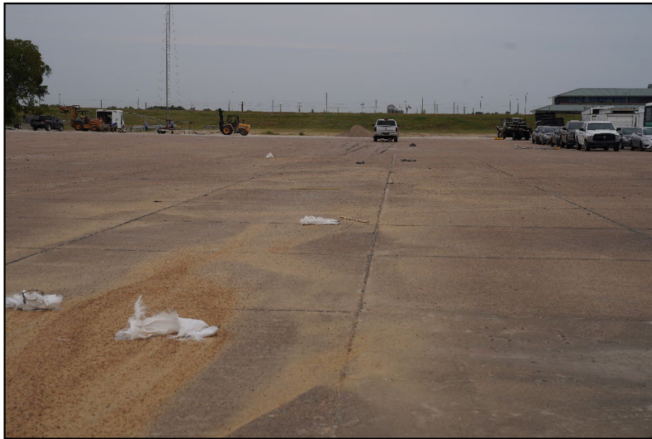
Figure 10.5. Type III Barricade with Mounted Sign after Test at Impact Location 616411-01-4.
