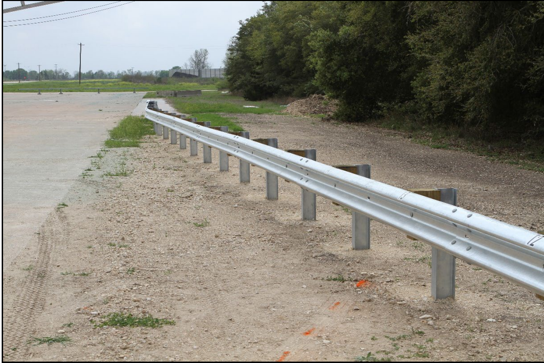
Figure 2.14. MGS Guardrail with Shortened 11:1 Flare at Impact prior to Testing.
