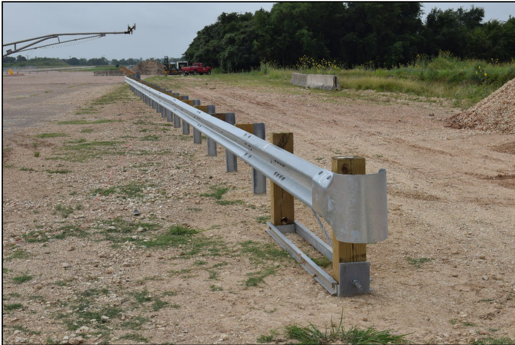
Figure 2.7. MGS Guardrail with 11:1 Flare prior to Testing.
