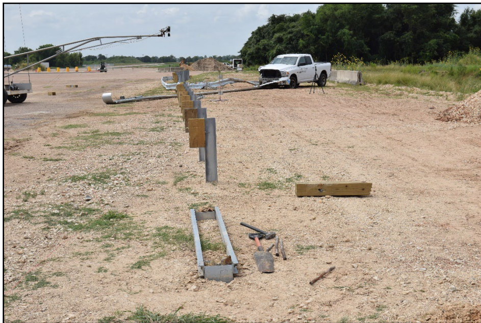
Figure 6.6. MGS Guardrail with Flare after Test 609971-03-1.
