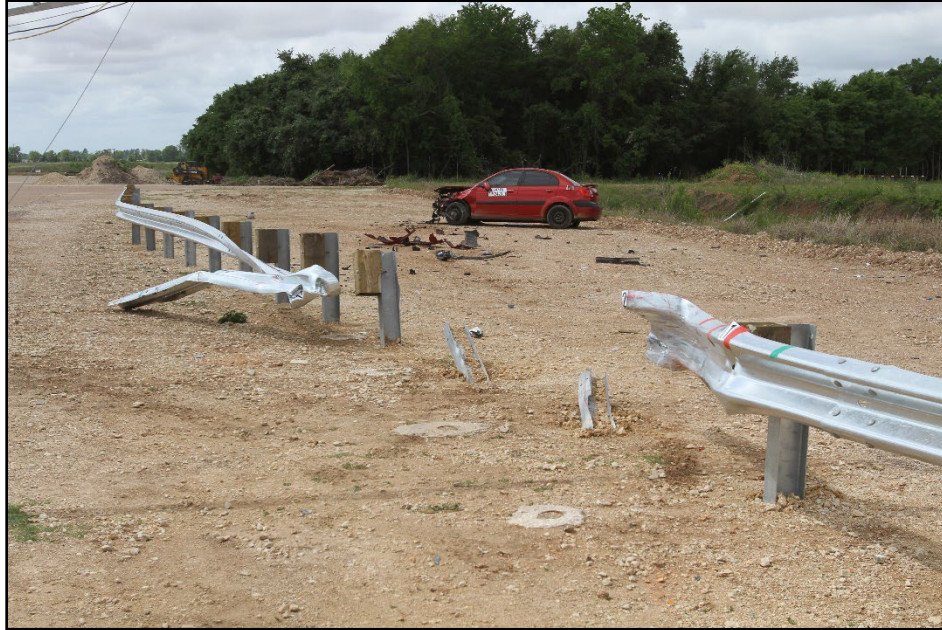
Figure 5.5. MGS Guardrail with Flare after Test at Impact Location for Test 609971-01-1.
