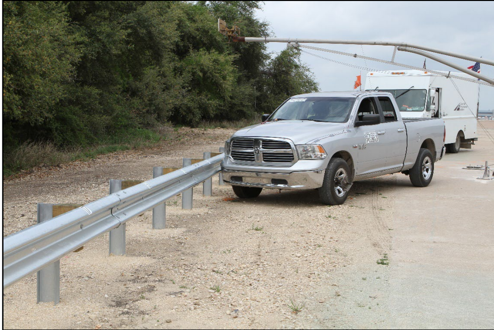
Figure 7.1. MGS Guardrail with Flare/Test Vehicle Geometrics for Test 609971-03-2.
