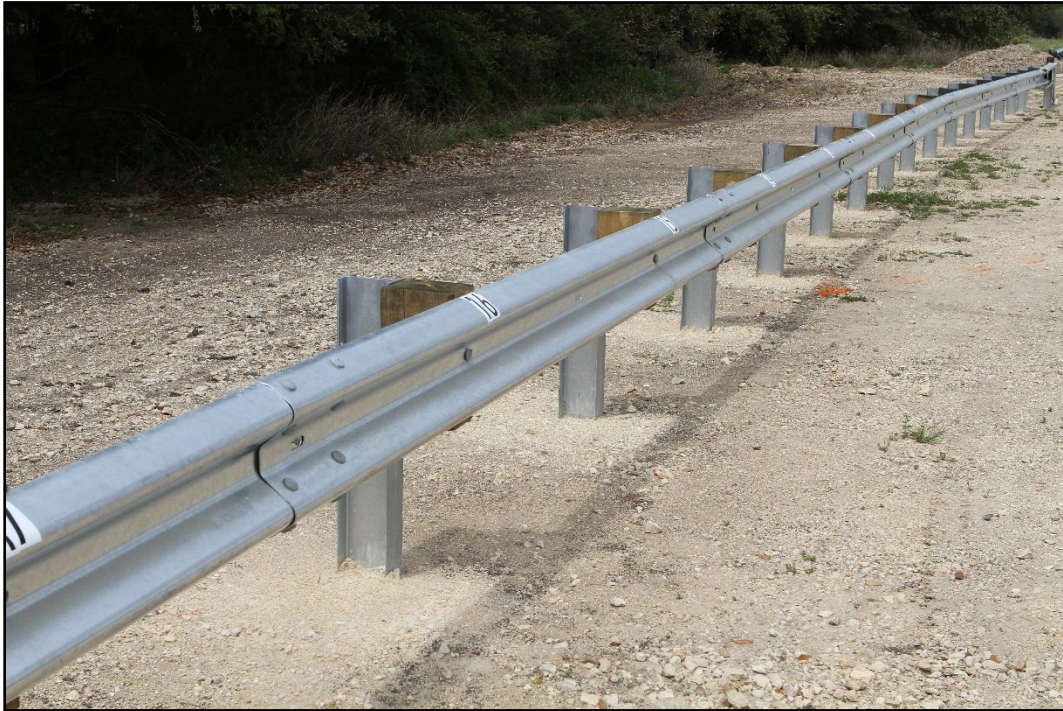
Figure 2.15. Downstream View of MGS Guardrail with Shortened 11:1 Flare prior to Testing.
