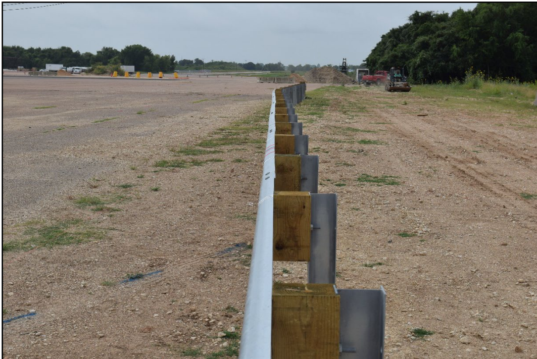
Figure 2.10. In-line View of the MGS Guardrail with 11:1 Flare prior to Testing.
