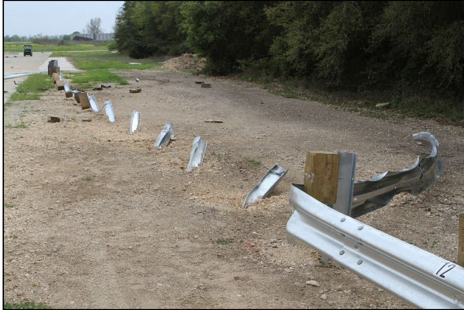
Figure 7.5. MGS Guardrail with Flare after Test at Impact Location for Test 609971-03-2.
