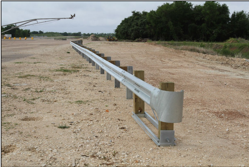
Figure 2.2. MGS Guardrail with 7:1 Flare prior to Testing.
