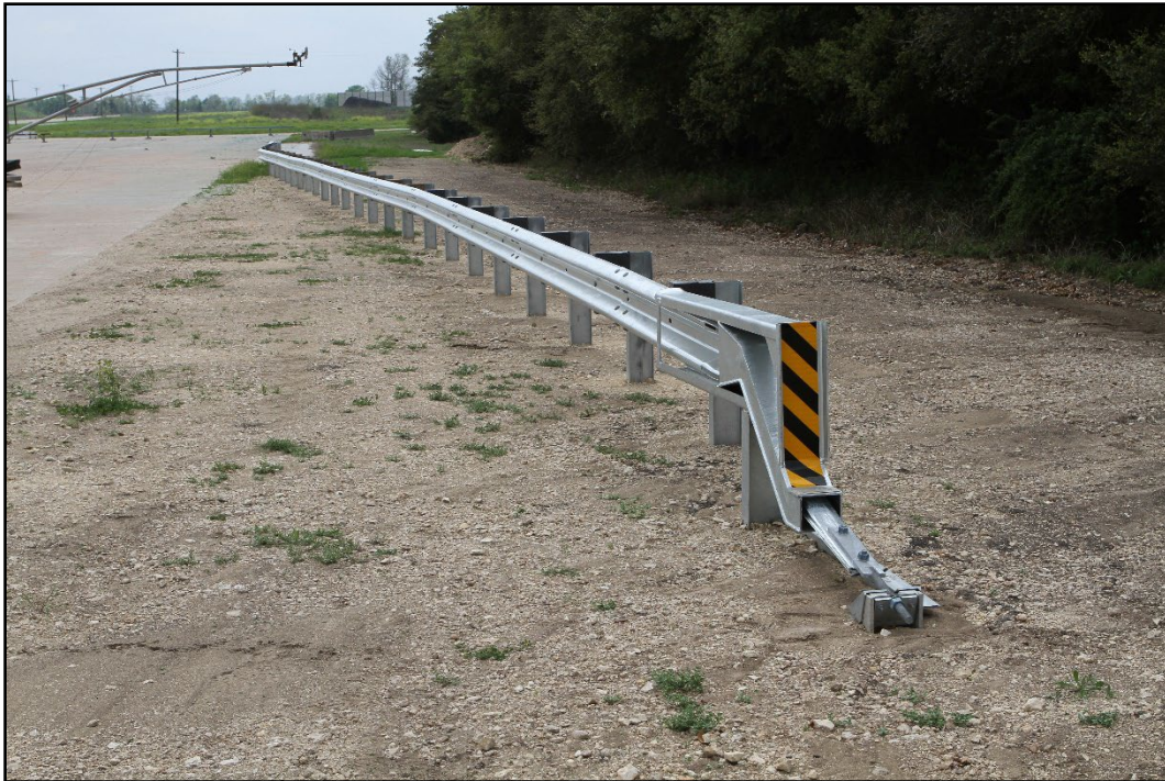
Figure 2.12. MGS Guardrail with Shortened 11:1 Flare prior to Testing.
