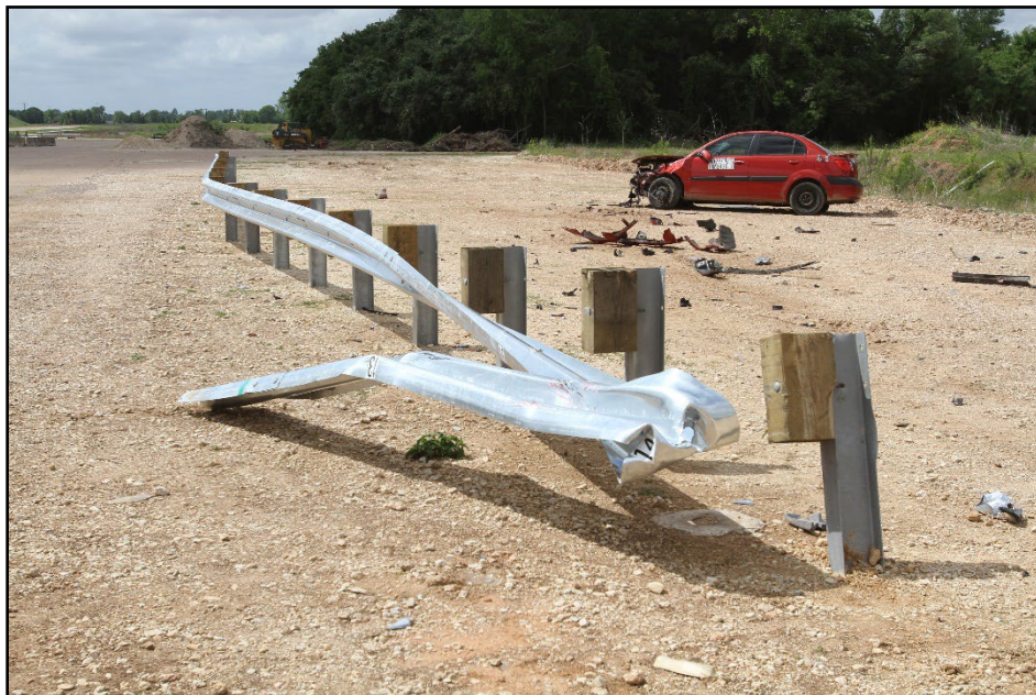
Figure 5.6. MGS Guardrail with Flare after Impact for Test 609971-01-1.
