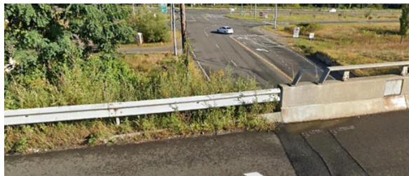
Figure 1. Trailing End Connection on Downstream End of Bridge Parapet
