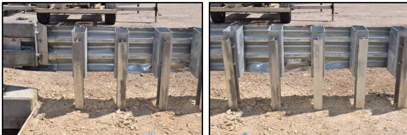
Figure 5. MASH Test 3-21 (Test NO. 608331-01-5)
