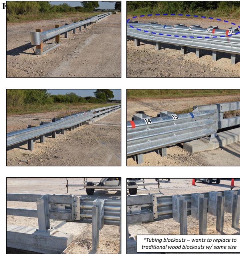
Figure 3. Alaska 2-Tube Bridge Rail Thrie Beam Transition prior to Testing
