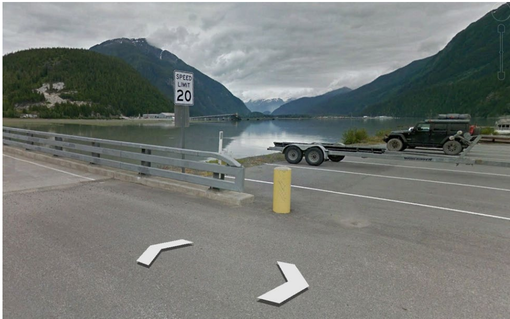
Figure 3: Bollard end treatment; low-speed parking lot application.
