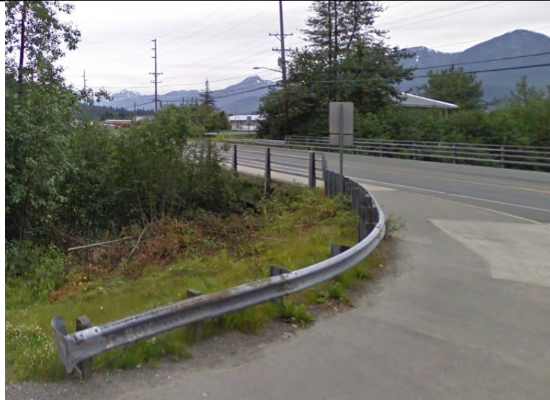
Figure 2: Steep slopes and short-radius turn resulted in improvised transition.
