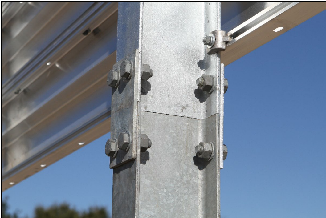
Figure 2.12. Hinge Plate of the Large Sign Slip Base Support Prior to Testing 612261-04-1.
