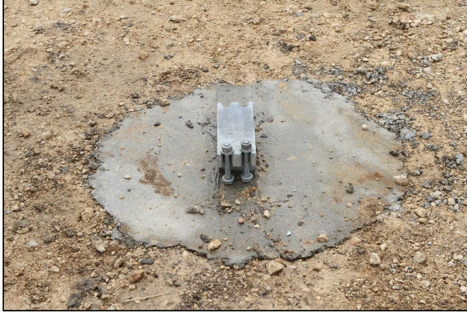
Figure 5.6. Left/Driver Large Sign Slip Base Support after Test at the Left Support Base 6122561-05-1.
