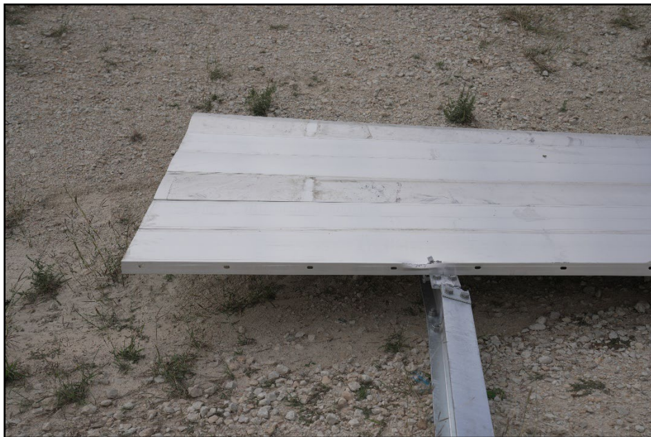
Figure 7.6. Large Sign Slip Base Support after Test at the Impacted Support 612261-05-2.
