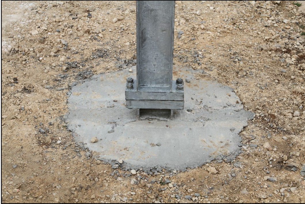
Figure 2.6. Base of the Large Sign Slip Base Support Prior to Testing 612261-05-1.
