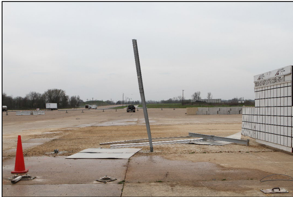
Figure 5.5. Large Sign Slip Base Support after Test at Impact Location 6122561-05-1.
