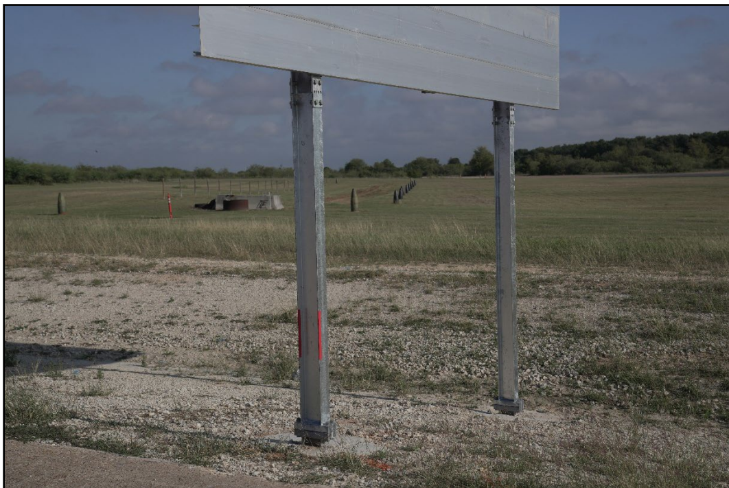
Figure 2.17. Large Sign Slip Base Support on a Slope In-line with the Impact Path Prior to Testing 612261-05-2.
