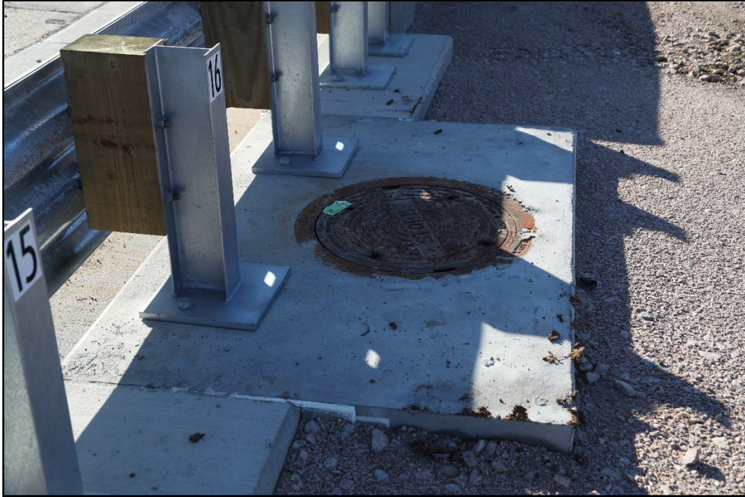
Figure 5.6. Storm Drain Inlet Location Prior to Testing.
