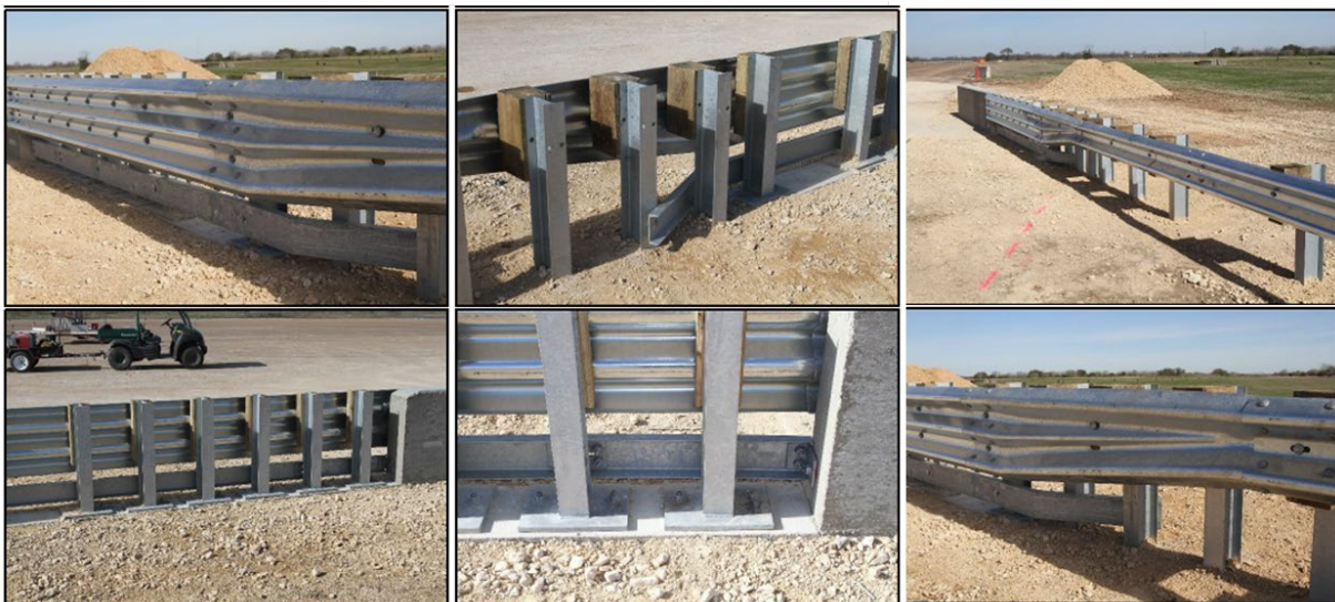
Figure 3.1. Wingwall Transition System (5).
