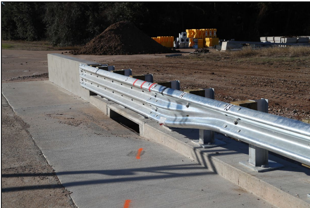
Figure 5.3. Transition with Storm Drain Inlet Prior to Testing.
