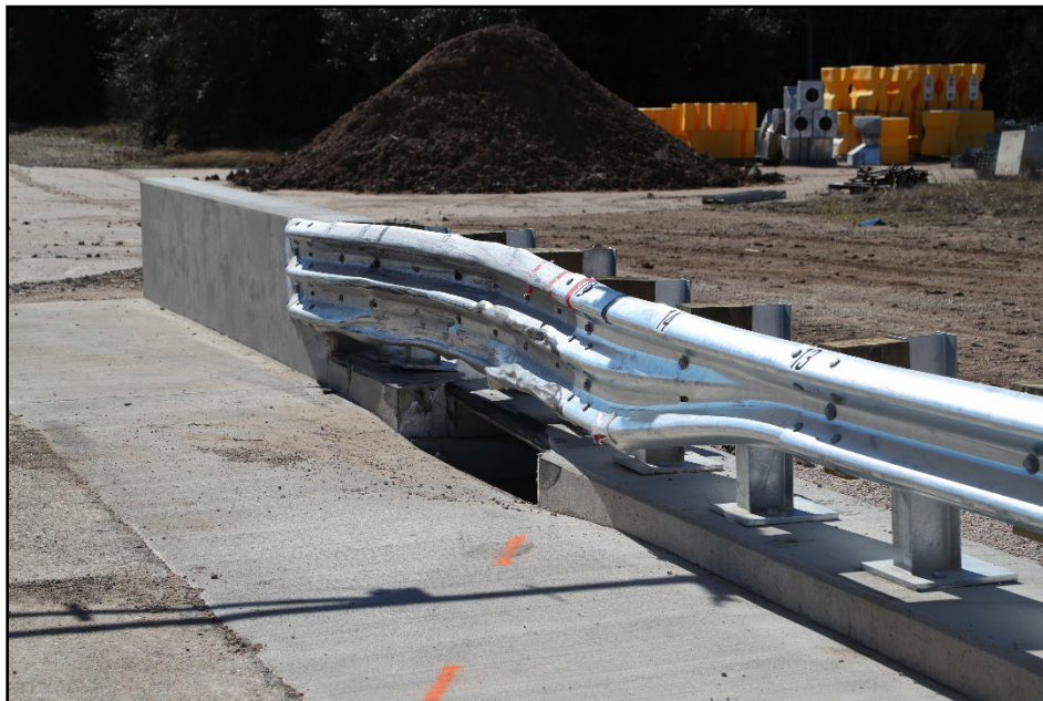
Figure 8.5. Transition with Storm Drain Inlet at Impact Location after Test 615251-01-1.
