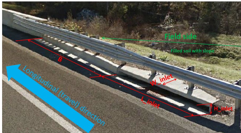
Figure 2.1. Key Parameters for Placing Storm Drain Inlet.
