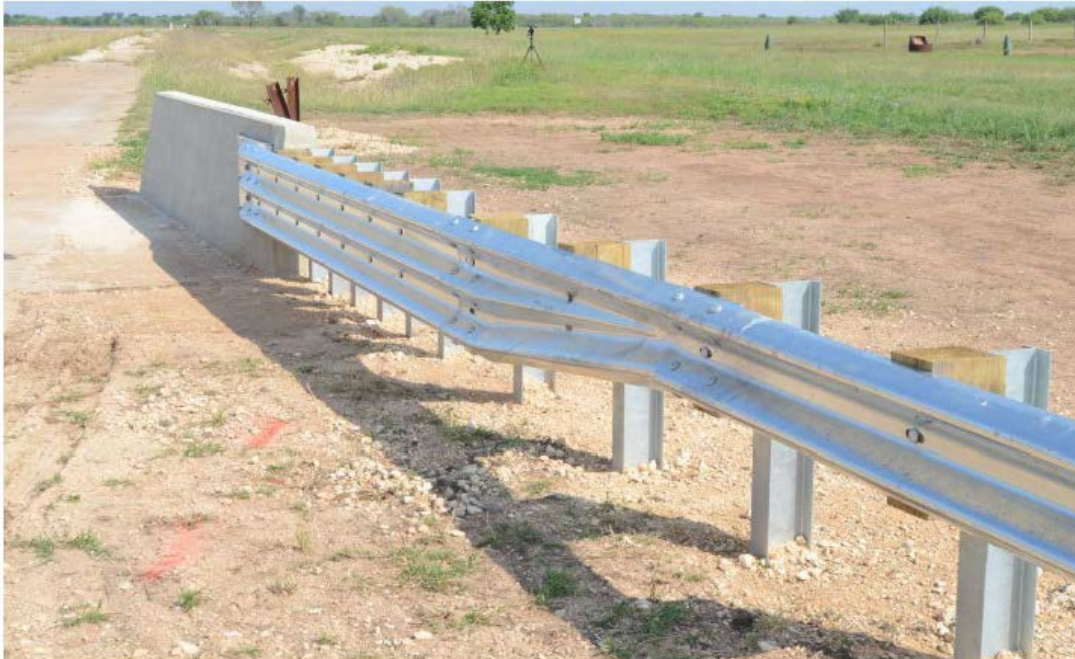
Figure 2.8. Thrie-Beam Transition without Curb or Rubrail [13].
