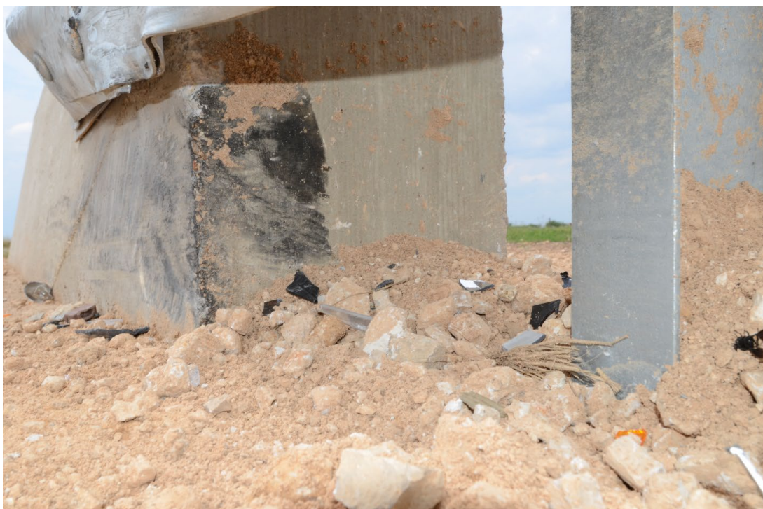
Figure 2.9. Tire Snagging on End of Single-Slope Concrete Transition Parapet [13].
