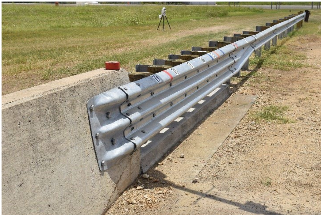
Figure 2.10. Thrie-Beam Transition without End Shoe Block [14].
