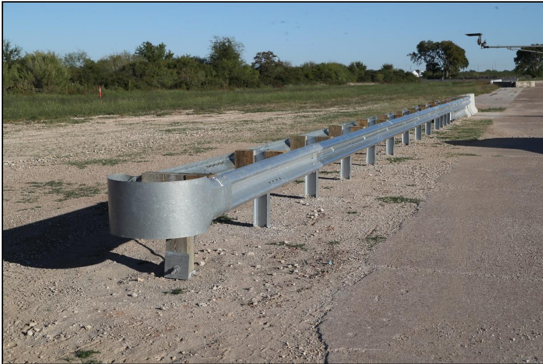
Figure 3.2. Median Guardrail Transition to Median F-Shape Barrier prior to Testing.
