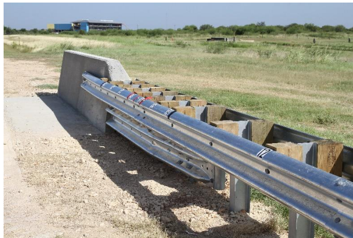
Figure 1.1. MASH TL-3 Median Guardrail Transition to Median Single Slope Barrier. (2)
