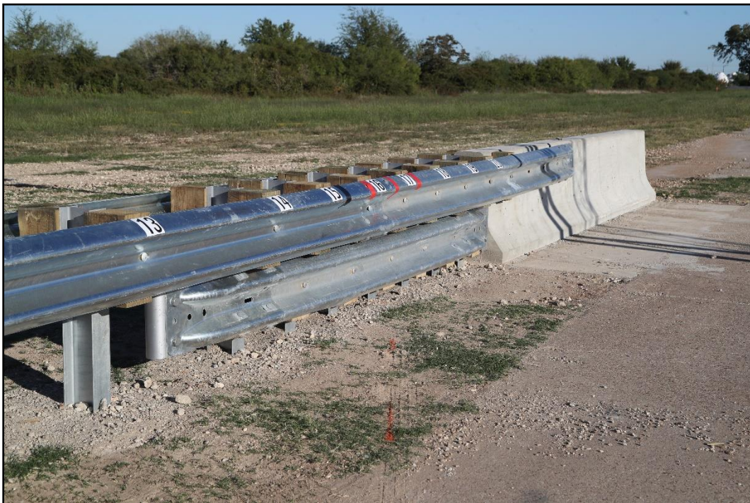
Figure 3.3. Median Guardrail Transition to Median F-Shape Barrier at Impact prior to Testing.
