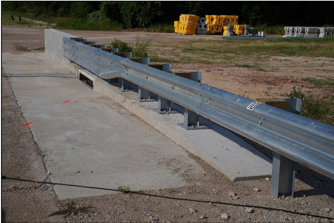
Figure 2.2. TL-3 Transition with a Storm Drain Inlet prior to Testing.
