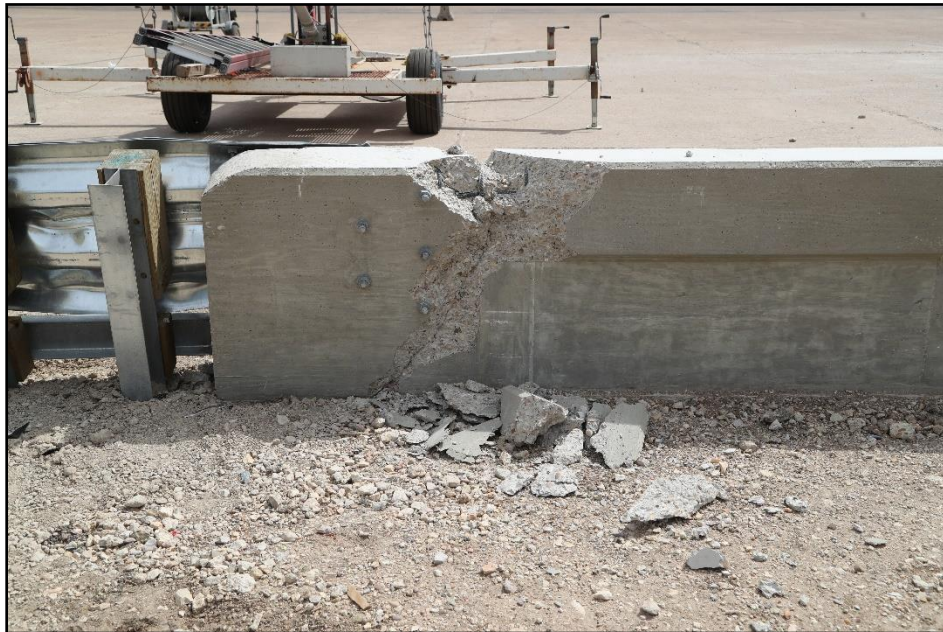
Figure 6.6. Field Side View of Shortened Transition of Concrete Parapet after Test 618981-01-1.
