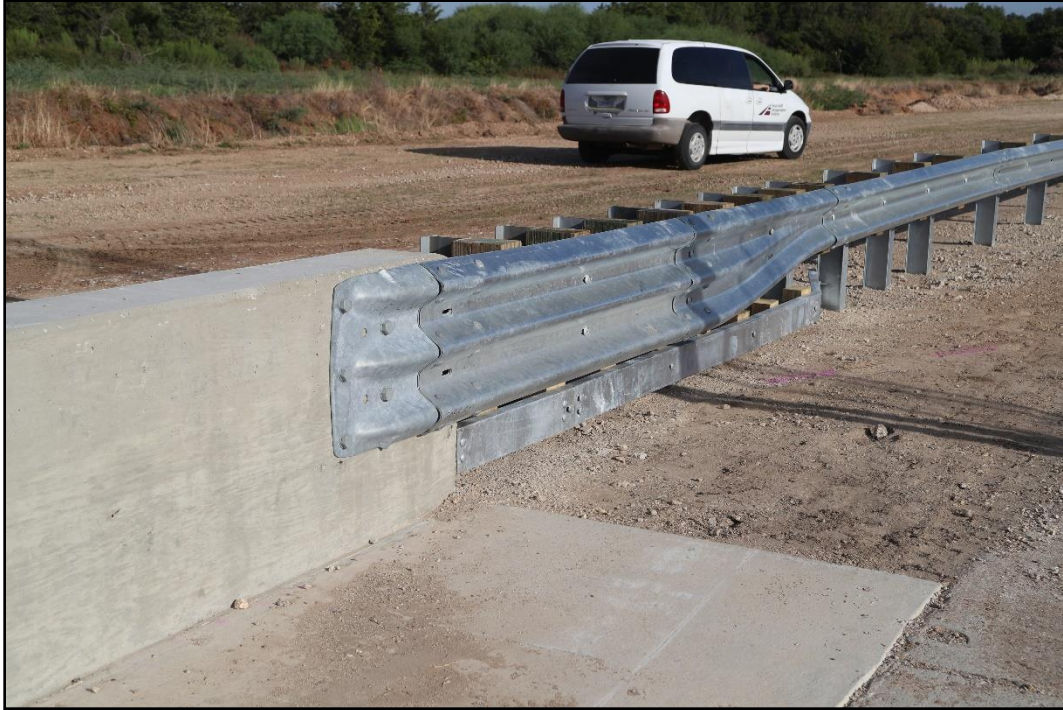
Figure 3.4. View of Shortened Transition from Downstream prior to Testing.
