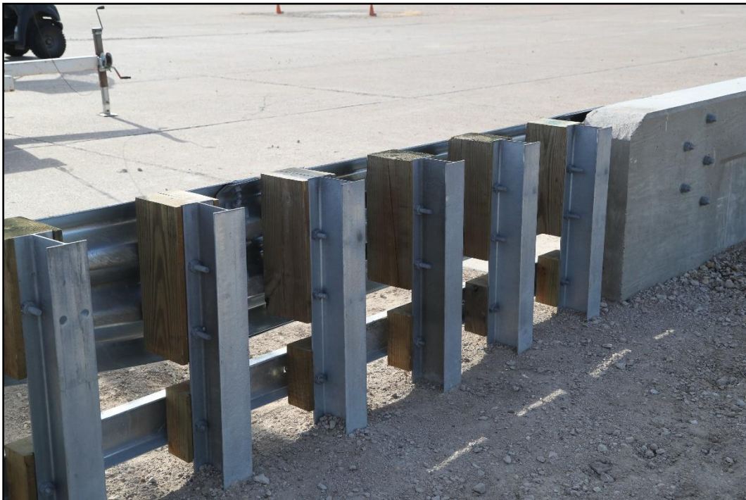
Figure 3.7. Field Side View of Shortened Transition prior to Testing.
