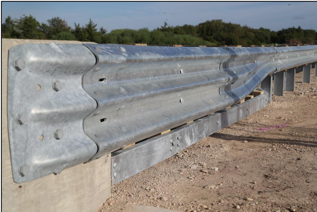
Figure 3.5. View of Shortened Transition from Downstream prior to Testing.
