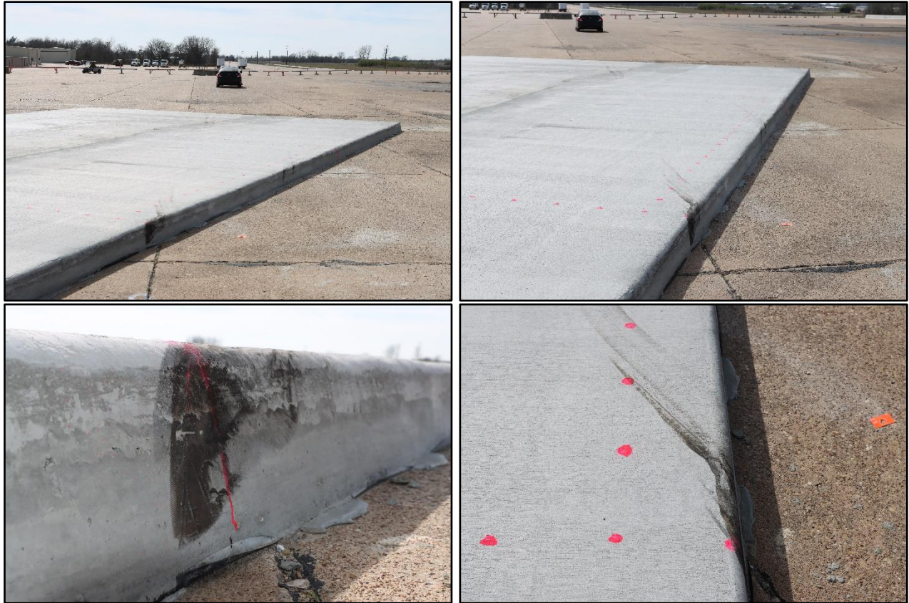
Figure 3.5. Sidewalk After Test No. 614091-01-1
