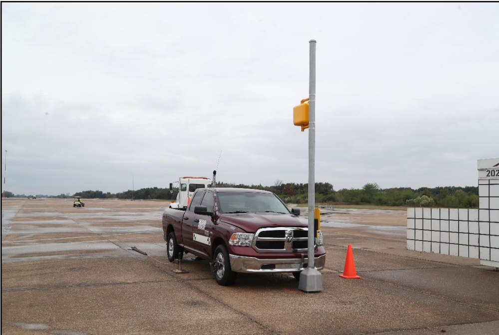
Figure 8.2. MUTCD Standard Pedestrian Signal /Test Vehicle Impact Location 617891-01-2.
