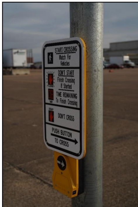
Figure 4.17. MUTCD Standard Pedestrian Signal with Audible Button Prior to Crash Tests 617891-01 3&4.
