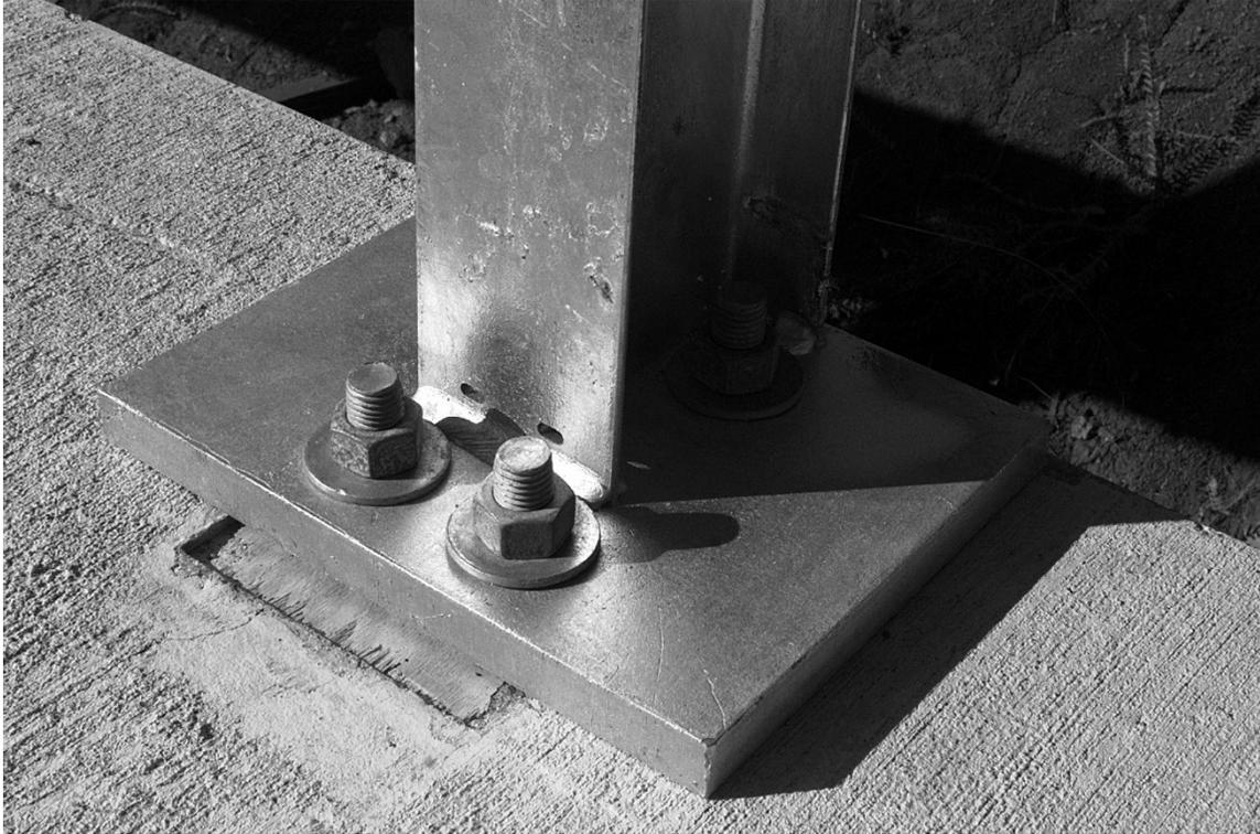
**Figure 2.4. TxDOT T6 Steel Post Welded Connection.**
