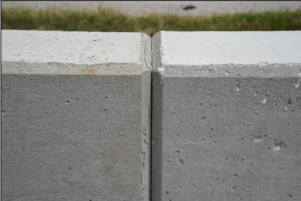
**Figure 3.7. Detail of the Top of the Cold Joint of the TL-5 Concrete Median Barrier with Shallow Embedment Prior to Testing.**
