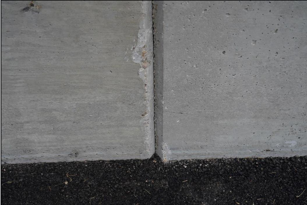
**Figure 3.6. Detail of Cold Joint at Grade of the TL-5 Concrete Median Barrier with Shallow Embedment Prior to Testing.**
