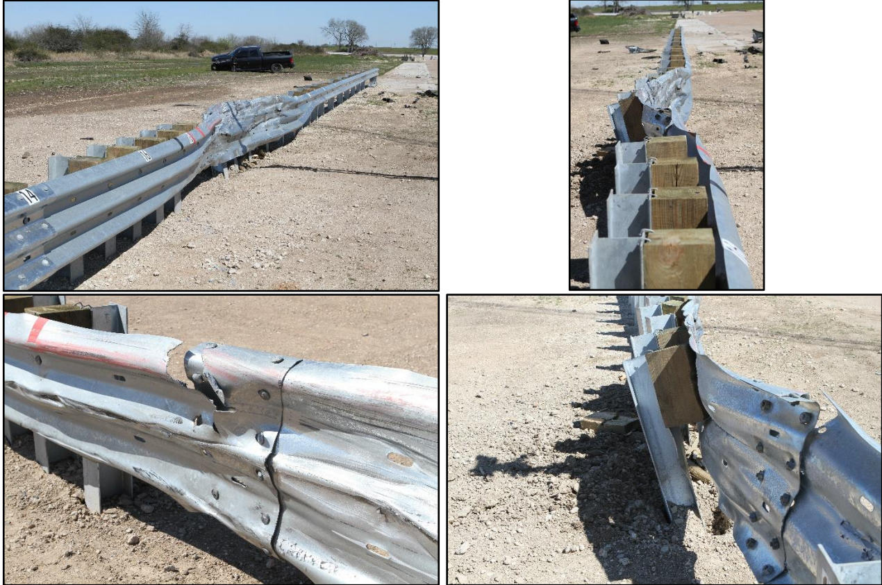
Figure 7.3 Thrie-Beam Guardrail System at a Fixed Object after Test (614031-01-1).
