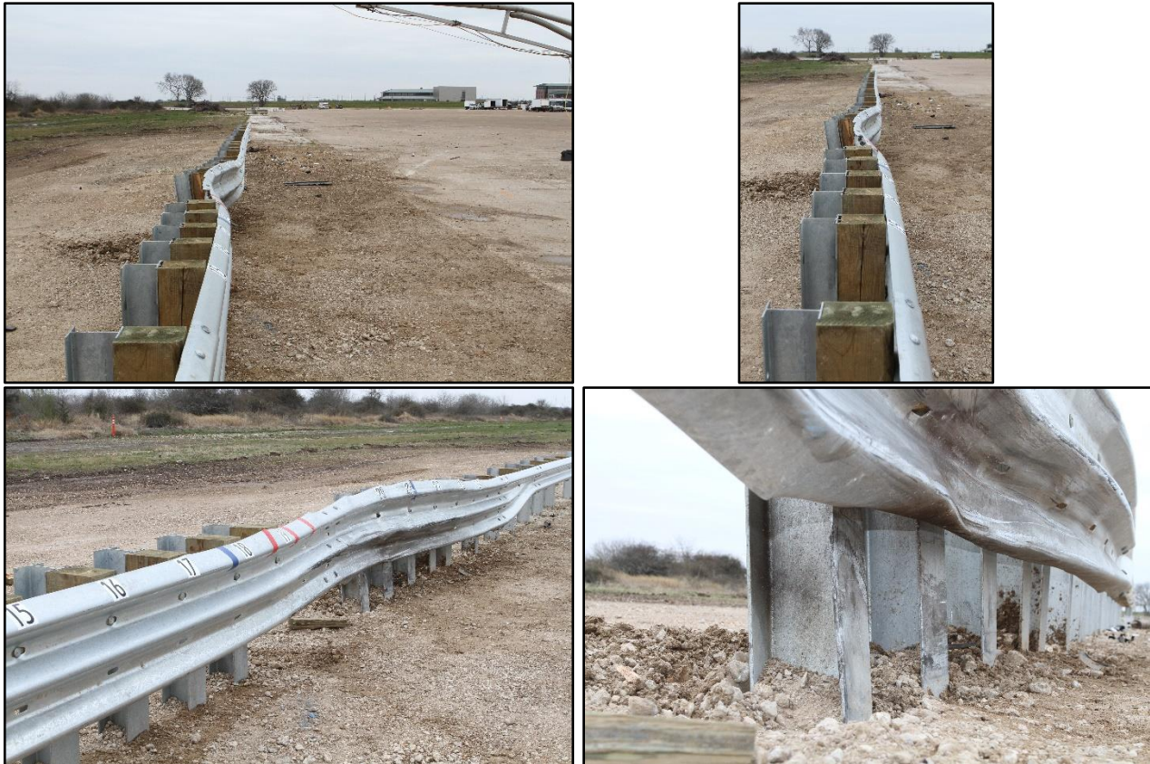
Figure 6.3 Thrie-Beam Guardrail System at a Fixed Object after Test 614031-01-2
