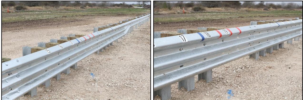
Figure 6.1 Thrie-Beam Guardrail System at a Fixed Object/Test Vehicle Geometrics for (Crash Test No. 614031-01-2)
