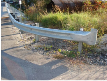
(a) Vermont G1-d W-beam Terminal
