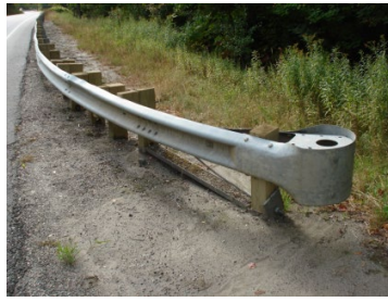
(b) NETC-MELT Guardrail End Terminal
