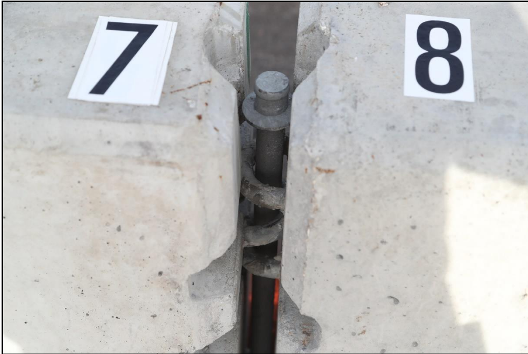
Figure 2.4. Closeup View of Joint Between Barriers 7 and 8 Prior to Testing.
