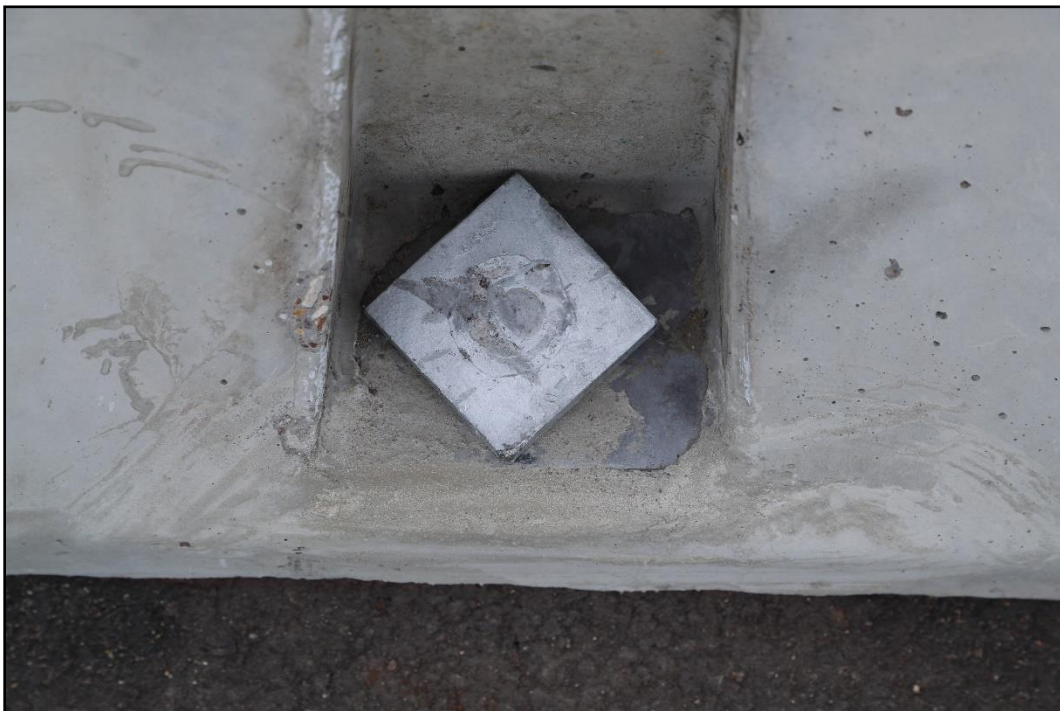
Figure 2.7. Closeup View of Installed Anchor Pin Prior to Testing.
