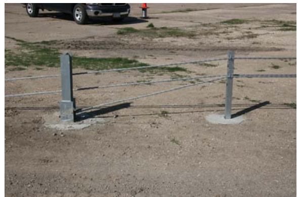
Figure 6. High-tension cable barrier prior to testing at 45 degrees.
