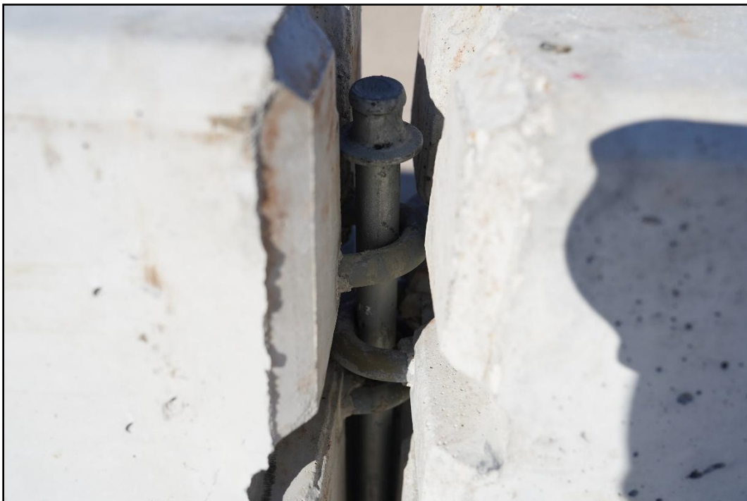
Figure 4.7. Connection Hardware for the Overlapping Precast Portable Concrete Barriers prior to Testing.
