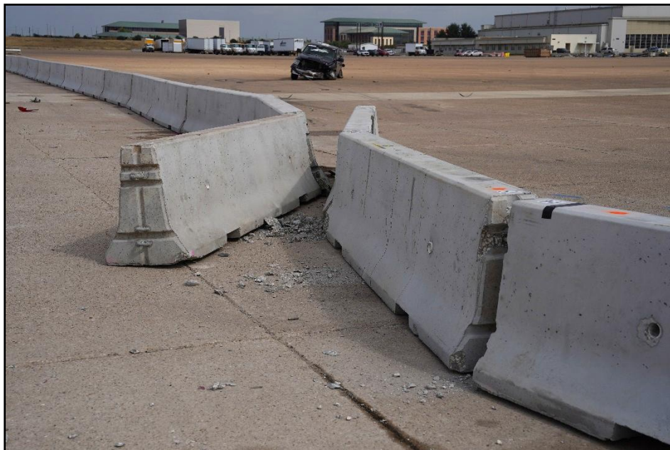
Figure 8.7. Field-Side of the Overlapping Precast Portable Concrete Barriers at Impact after Test 620281-01-2.
