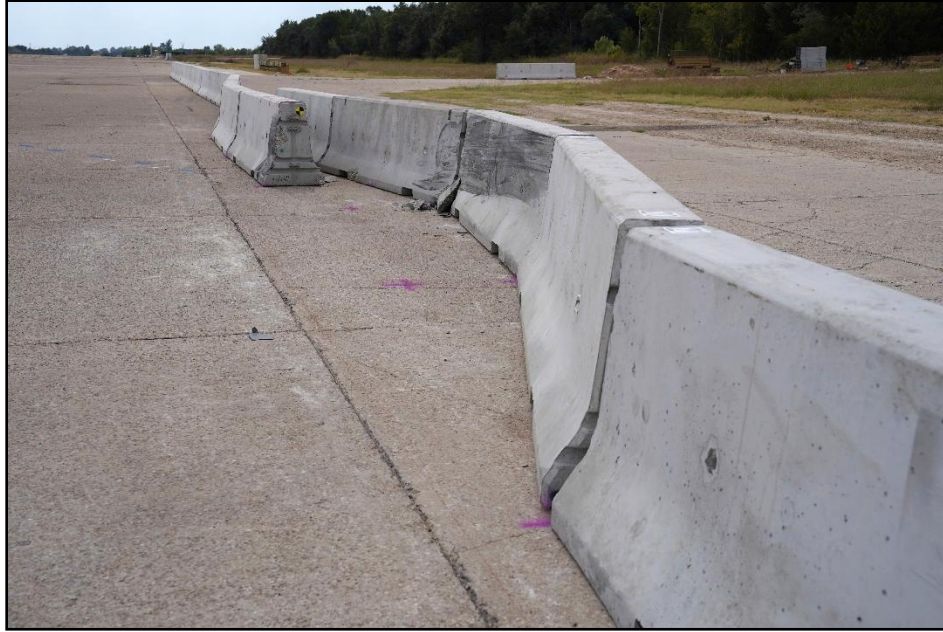
Figure 7.7. Upstream View of the Overlapping Precast Portable Concrete Barriers after Test 620281-01-1.
