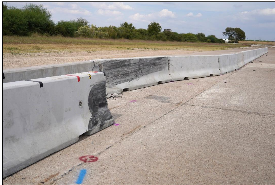
Figure 7.6. Overlapping Precast Portable Concrete Barriers at Impact Location after Test 620281-01-1.
