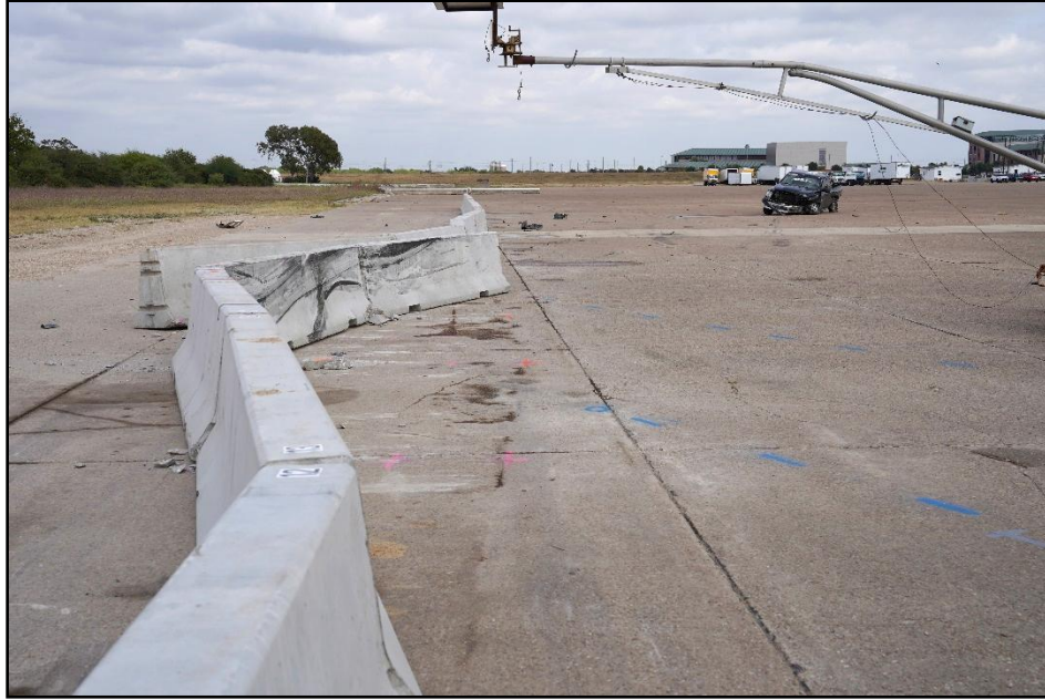
Figure 8.6. Overlapping Precast Portable Concrete Barriers at Impact Location after Test 620281-01-2.
