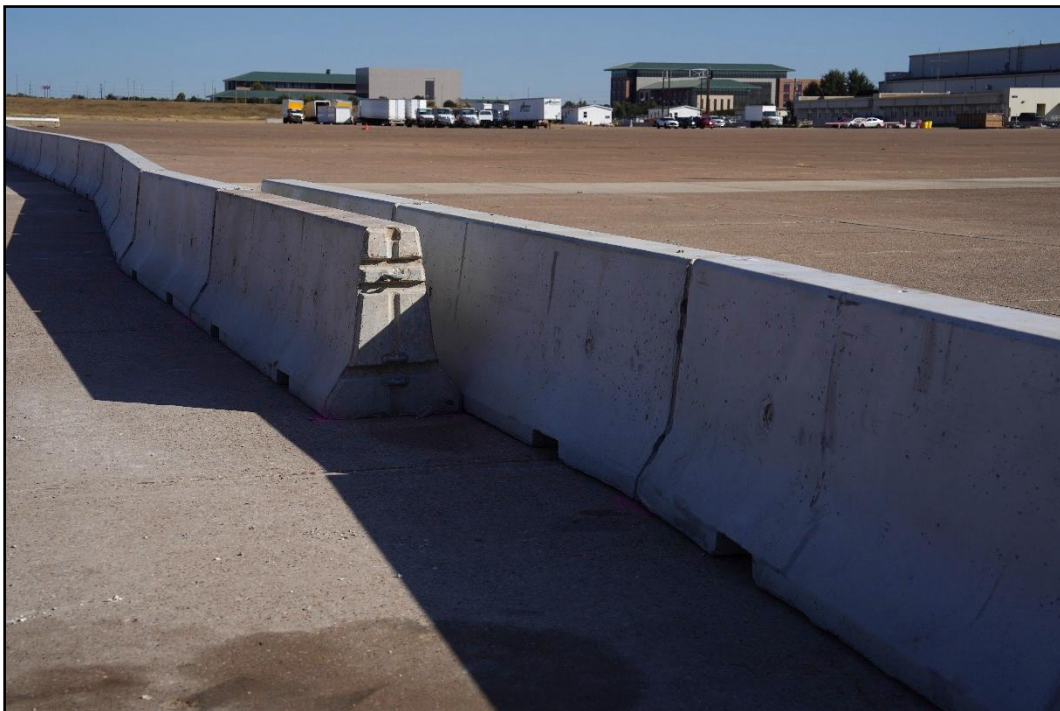
Figure 4.5. Field-Side of the Overlapping Precast Portable Concrete Barriers prior to Testing.
