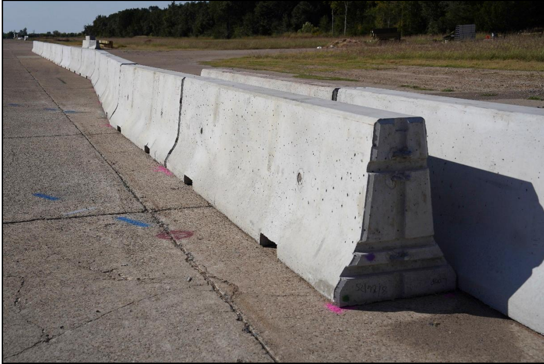
Figure 4.4. Downstream View of the Overlapping Precast Portable Concrete Barriers prior to Testing.
