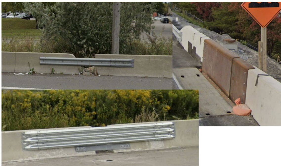
Figure 1.1. Retrofits for Bridging Gaps in Concrete Barriers
