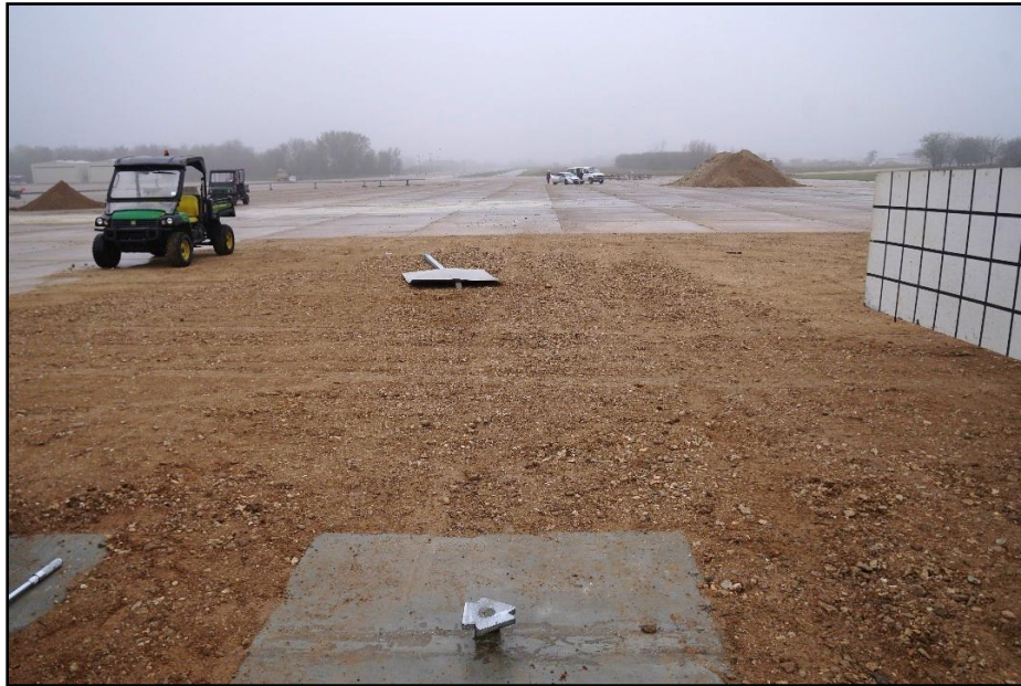
Figure 6.6. 3 × 3 Square Tube Slip Base Sign Support System at Impact Location after Test 621201-01-1.
